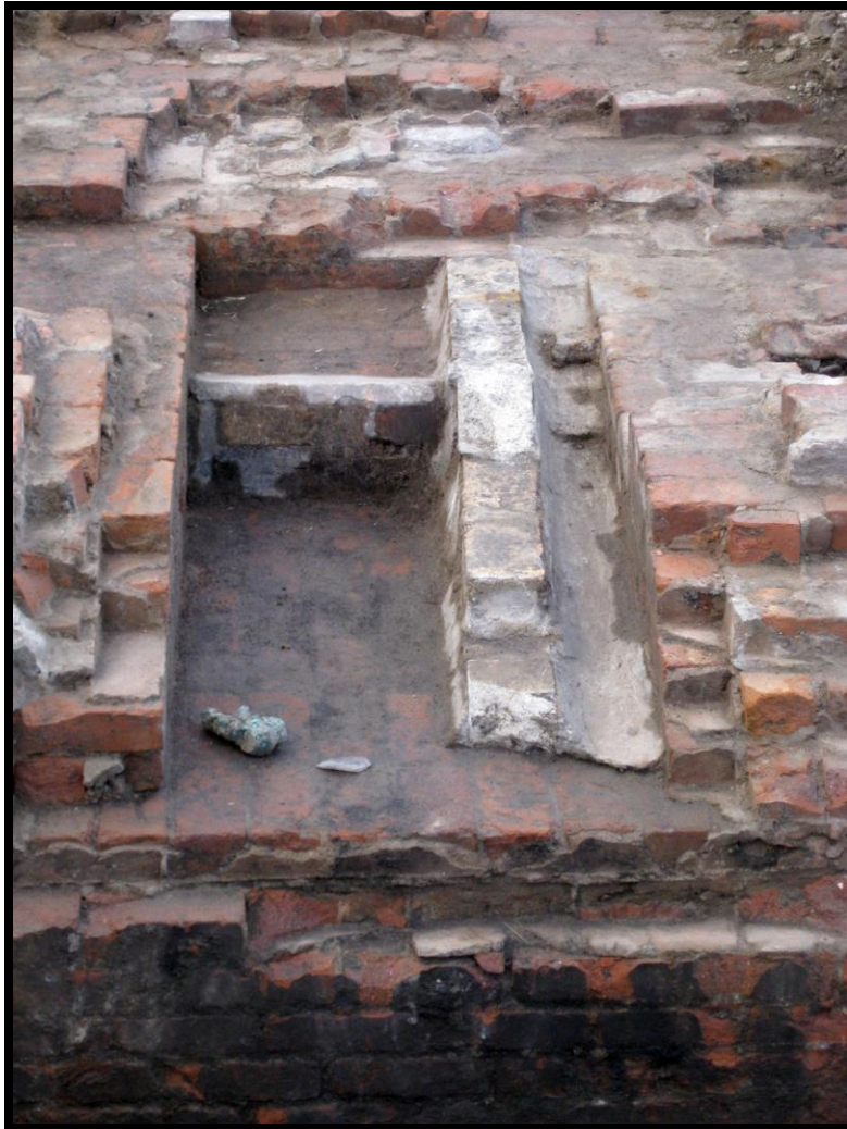
Photograph 4.20 Test Area 7, brick base with channels inset, looking south. The channeled area is constructed of fire-brick and faced with cement.
