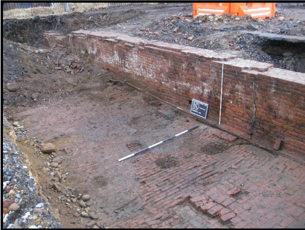
Photograph 4.31 Test Area 7, Trench 7.4, basement surface of main mill structure, looking southeast. Note structural crack in the foundation wall can be seen to the right.
