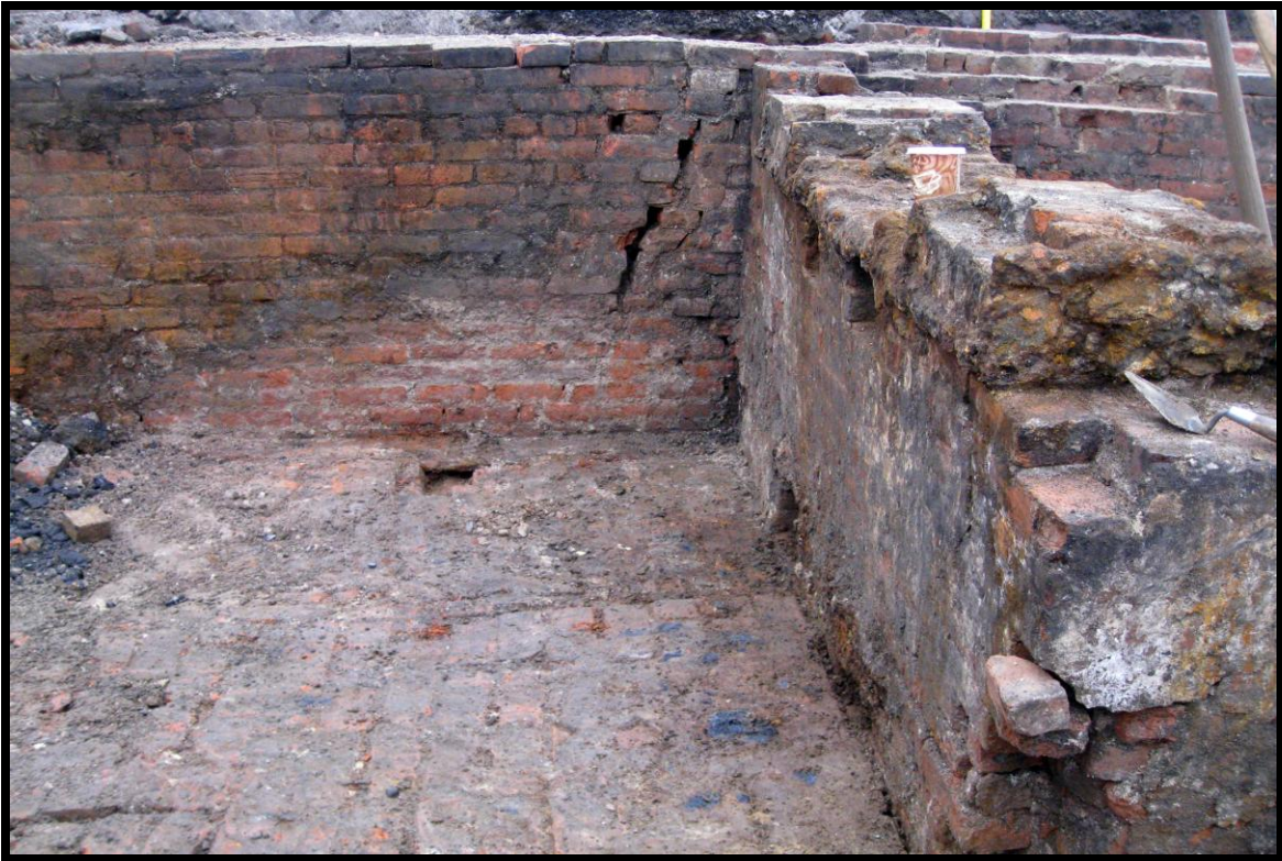
Photograph 4.33 Test Area 7, Trench 7.4, one of several structural cracks observed in the foundation wall, looking south. Boiler explosions, known to have occurred in this area of the mill, likely caused this damage.
