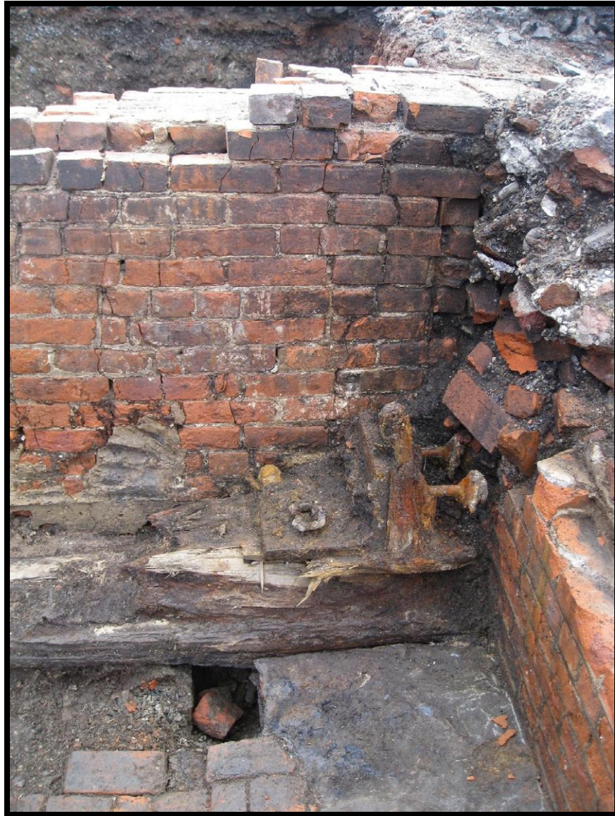
Photograph 4.36 Test Area 7, Trench 7.4, iron brackets securing wooden beams in the basement of main mill structure, looking south.
