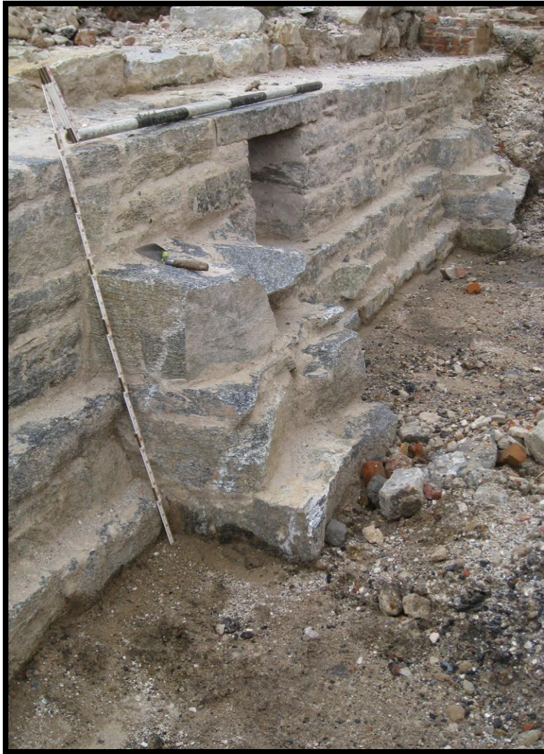
Photograph 4.10 Test Area 6, Feature 17, one of three stepped footers along the southern half of the center/party foundation wall, looking northeast.
