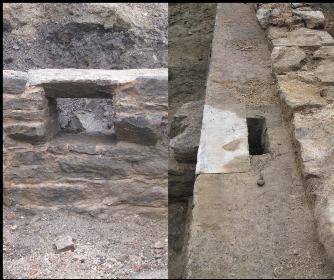
Photograph 4.12 Composite image displaying the side and top of ventilation openings within the foundation wall. This is consistent with the design in diagrams featured in Figures 4.6 and 4.7.
