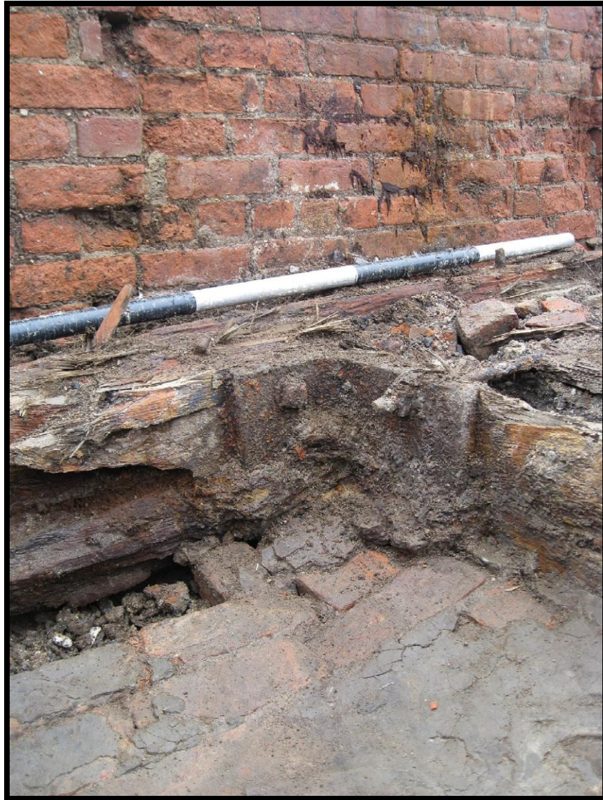
Photograph 4.37 Test Area 7, Trench 7.4, iron brackets securing wooden beams in the basement of the main mill structure, looking southwest.
