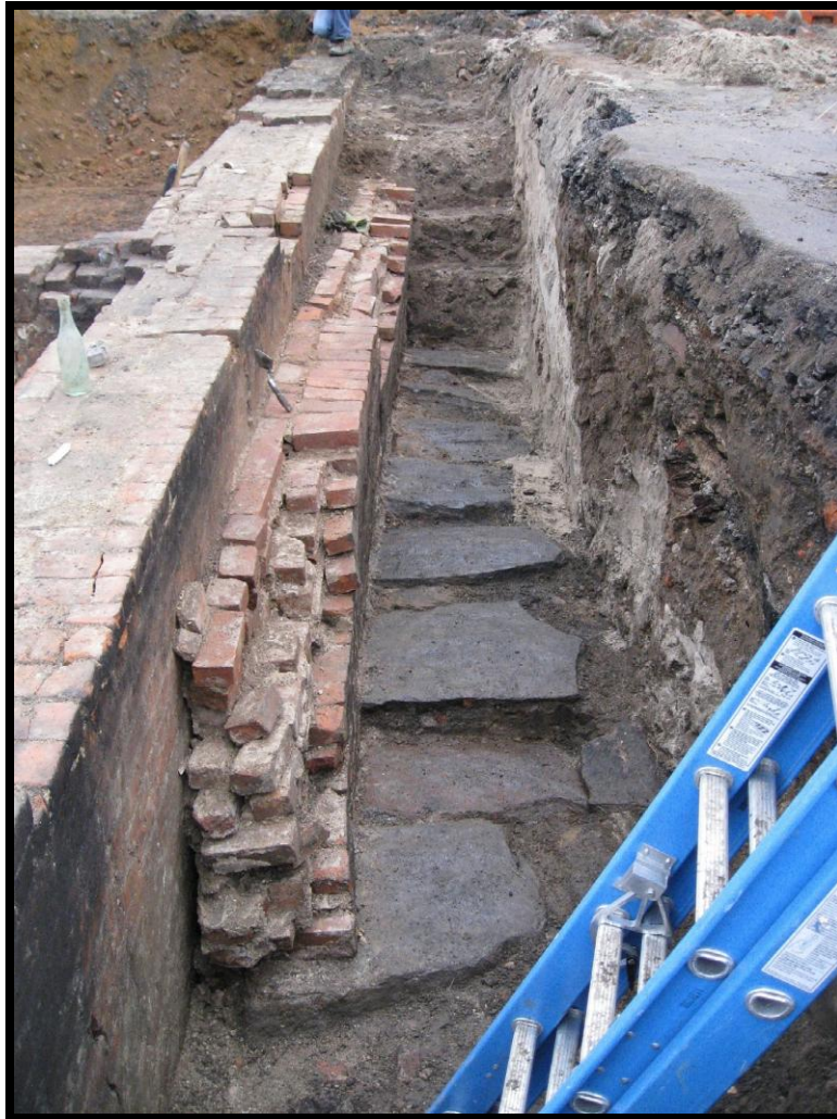
Photograph 4.34 Test Area 7, Trench 7.4, exterior southern foundation wall of the mill structure, looking east. shorter brick wall and stepped blue stone are a separate construction.
