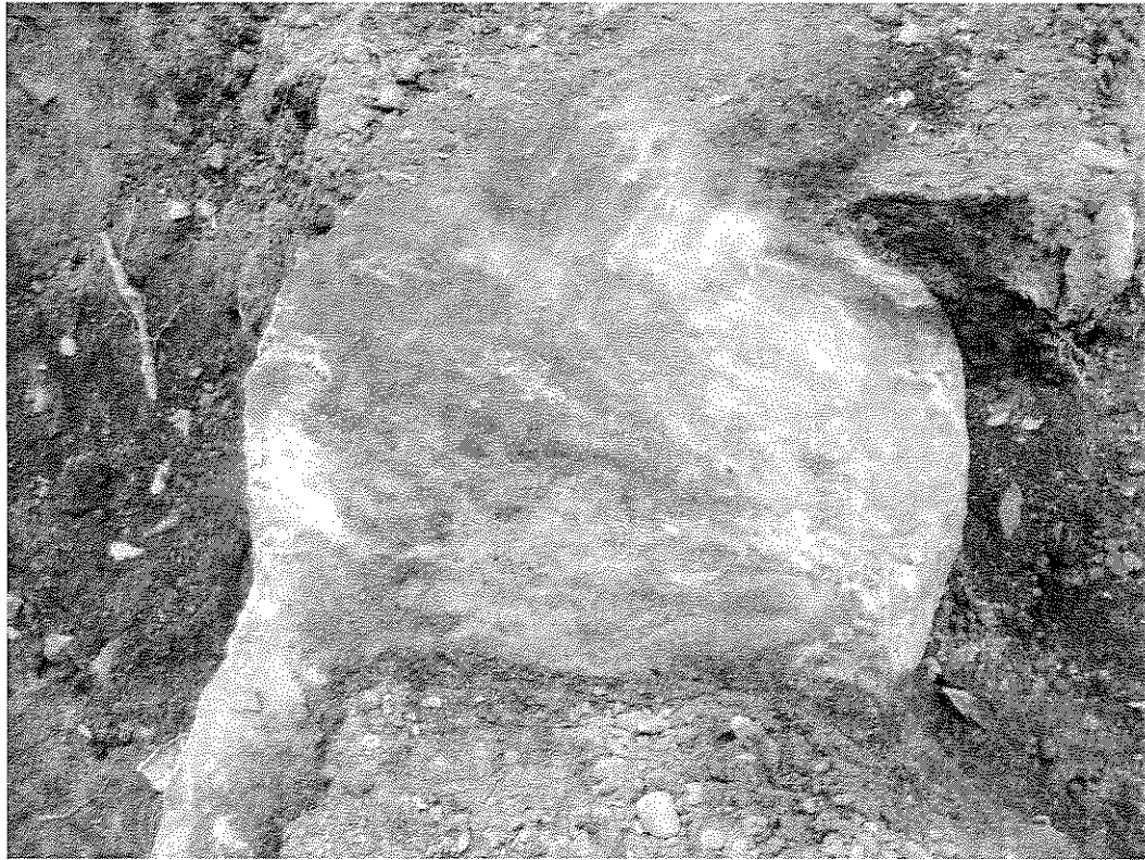
Figure 3B: A close-up of the column base incorporated into Wall C. This matches the location of columns in the wall surrounding the prison in early 20 th century photographs.
