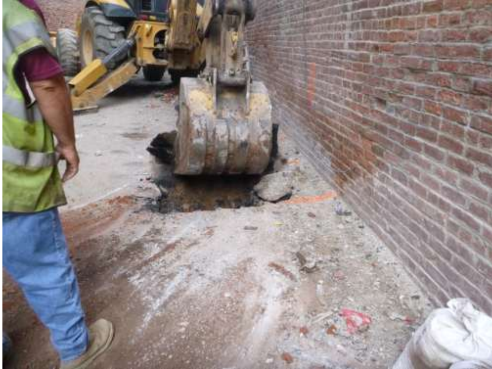
Image 22: Test Pit 02 - Excavation
