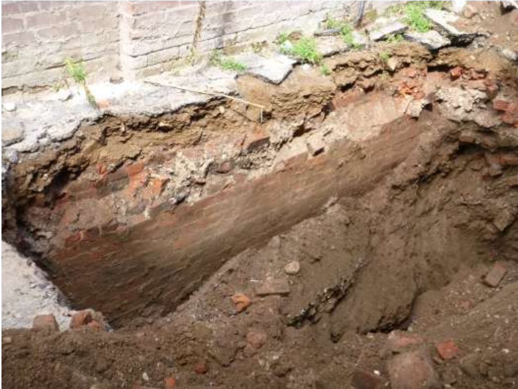
Image 09: Test Pit 3, south wall profile showing foundation wall of 265 Water Street.
