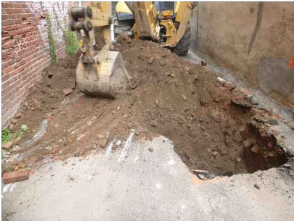
Image 30: Test Pit 05 – Excavation
