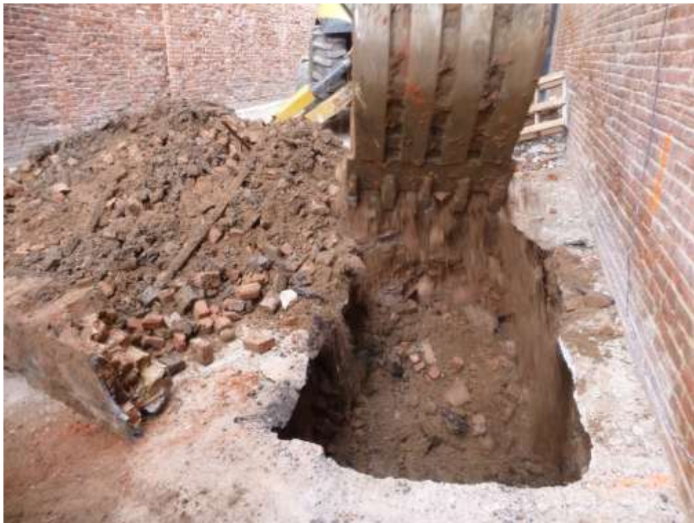
Image 21: Test Pit 02 - Excavation
