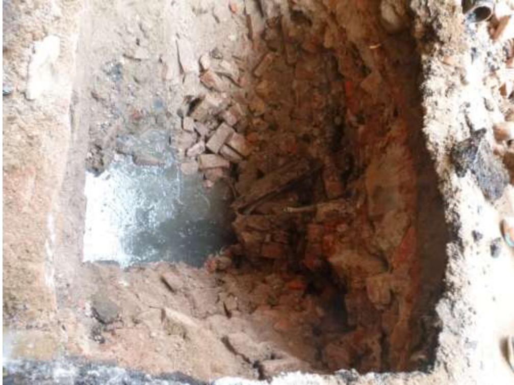
Image 18: Test Pit 01 - Water intrusion
