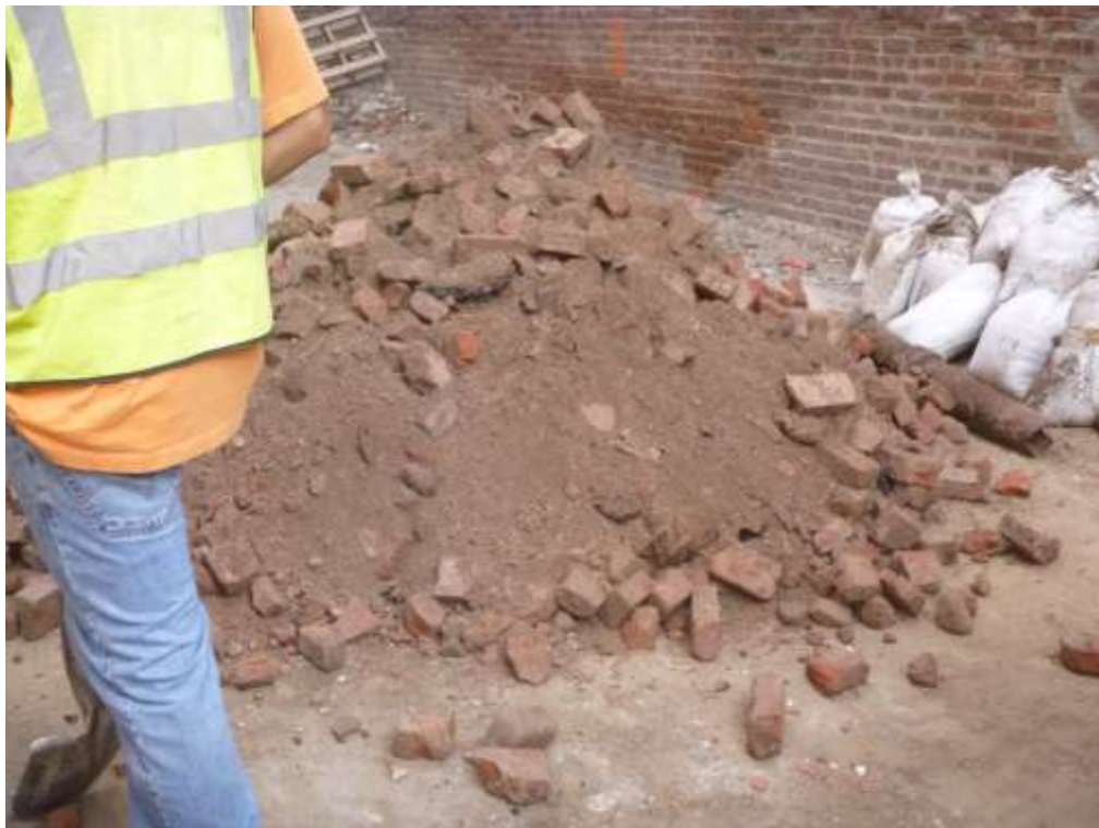
Image 19: Test Pit 01 – Back-dirt/construction rubble fill
