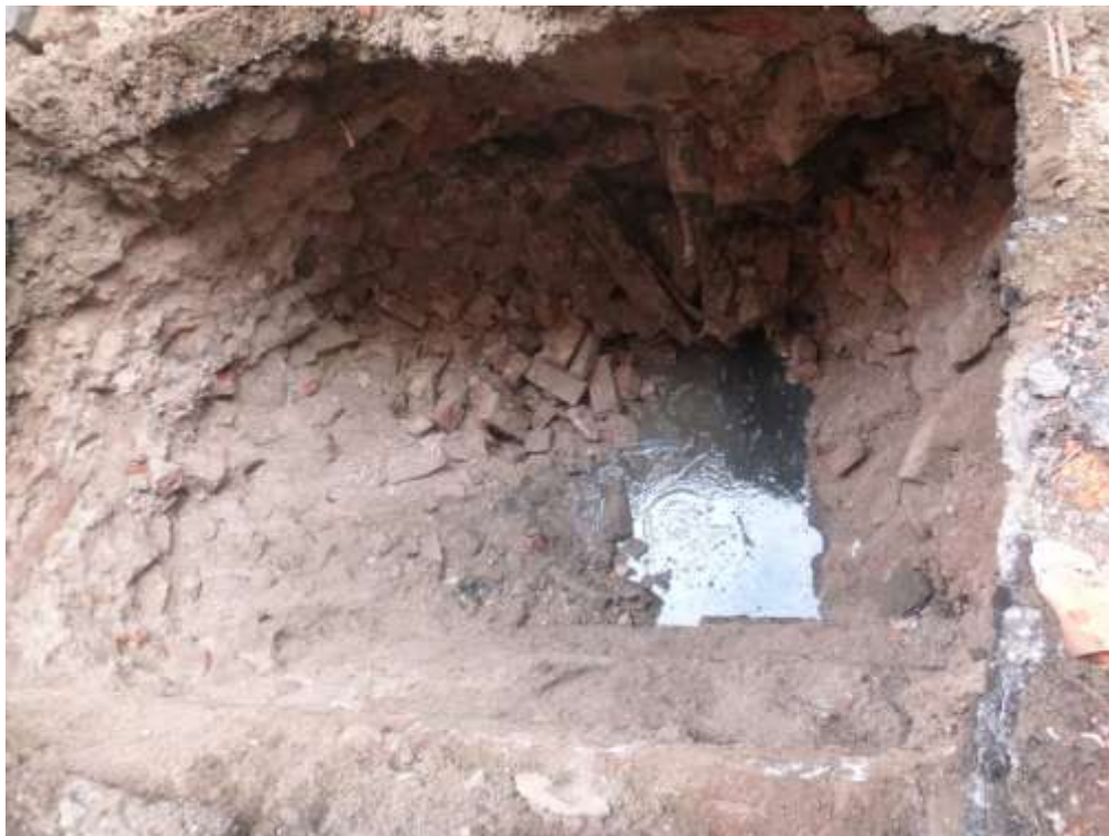
Image 17: Test Pit 01 - Water intrusion
