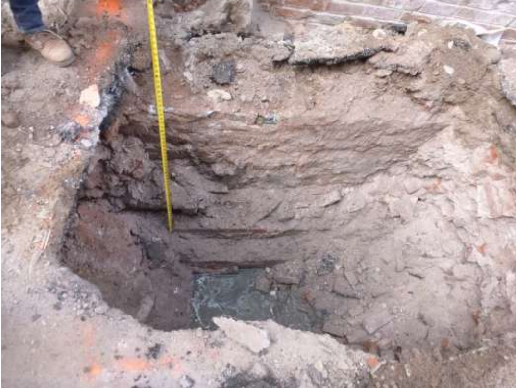
Image 05: Test Pit 1, south profile view of stone foundation and brick base.
