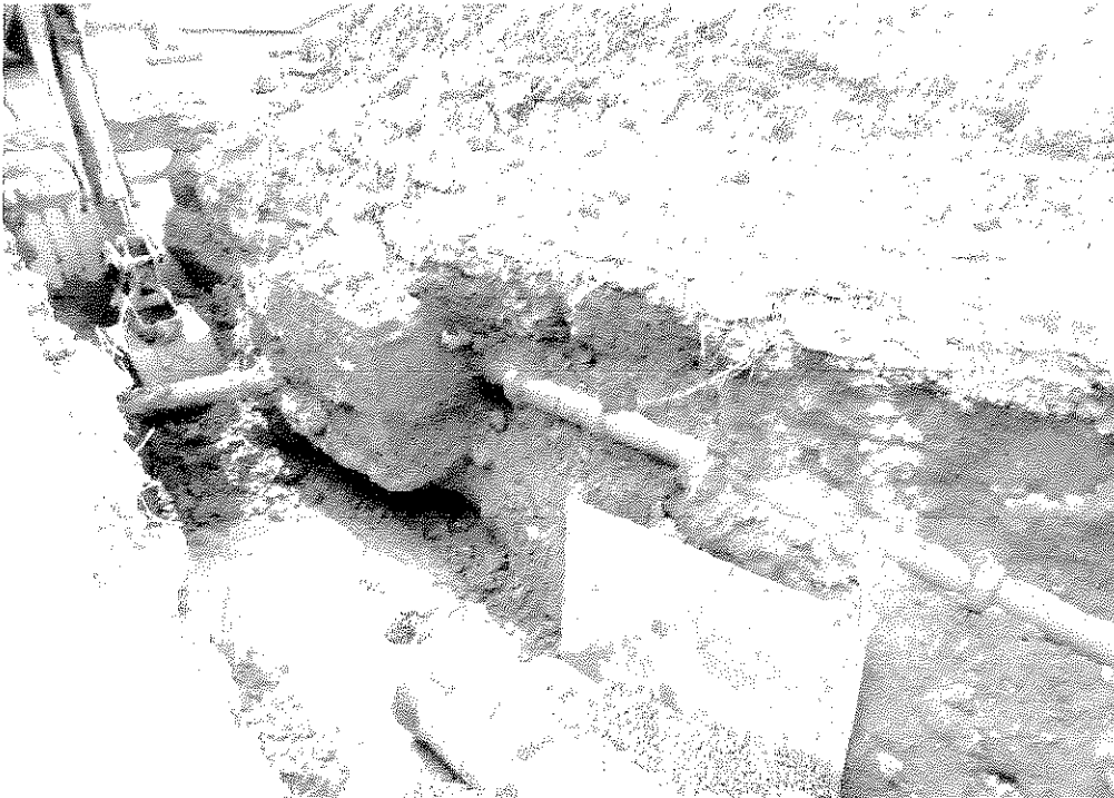
Photo 5 The brick feature first identified in CB 1.03 shown here as a utility encasement in the trench between CB 1.03 and MH 1.09, facing southwest (August 17, 2012).
