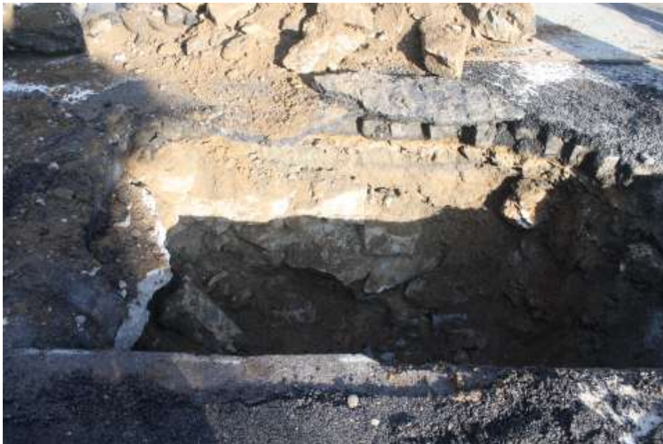
Image 22. SS Fulton, stone wall before collapse
