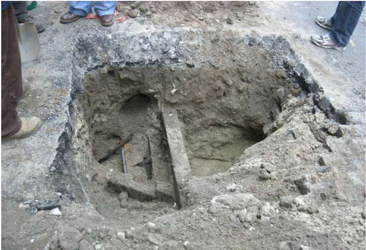
Image 32: Test Pit 9, looking west. Three wooden ducts are visible in the trench.
