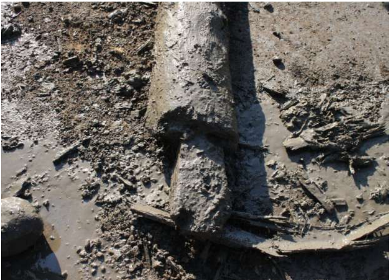
Image 21: Key-like end of log found in trench on Old Fulton Street near brick footings.
