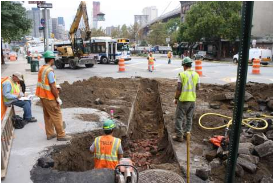
Image 123. Old Fulton and Elizabeth St, location of chute connection trench, looking W
