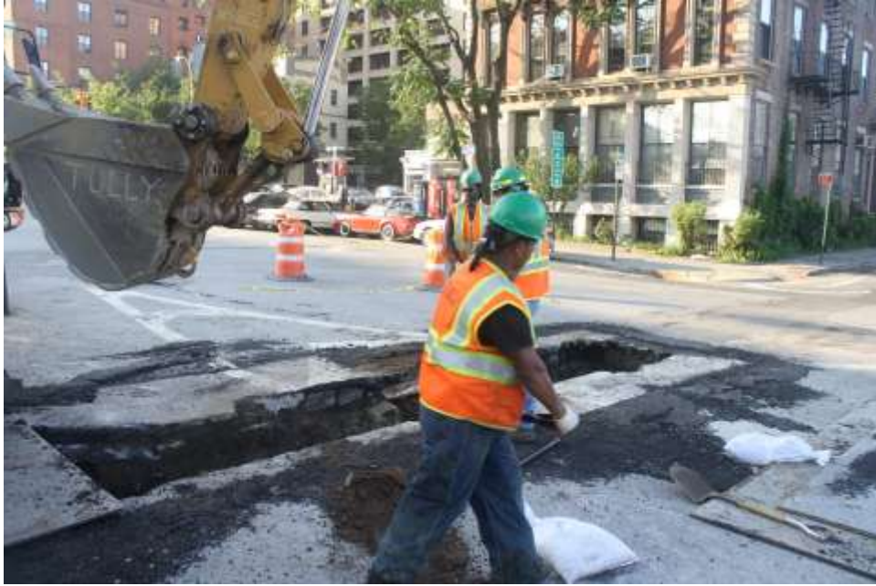
Image 58. Old Fulton, N/S segment of trench at foot of Old Fulton
