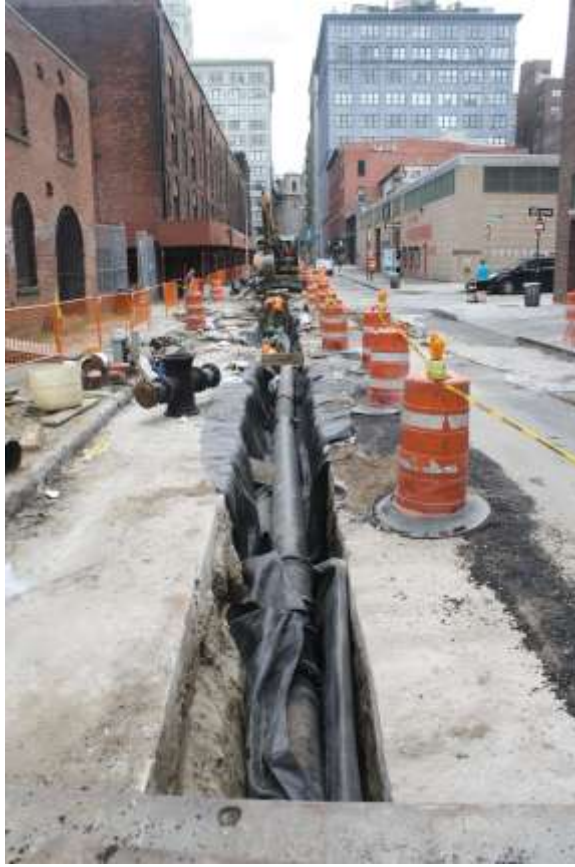
Image 82. Water St., trench looking E
