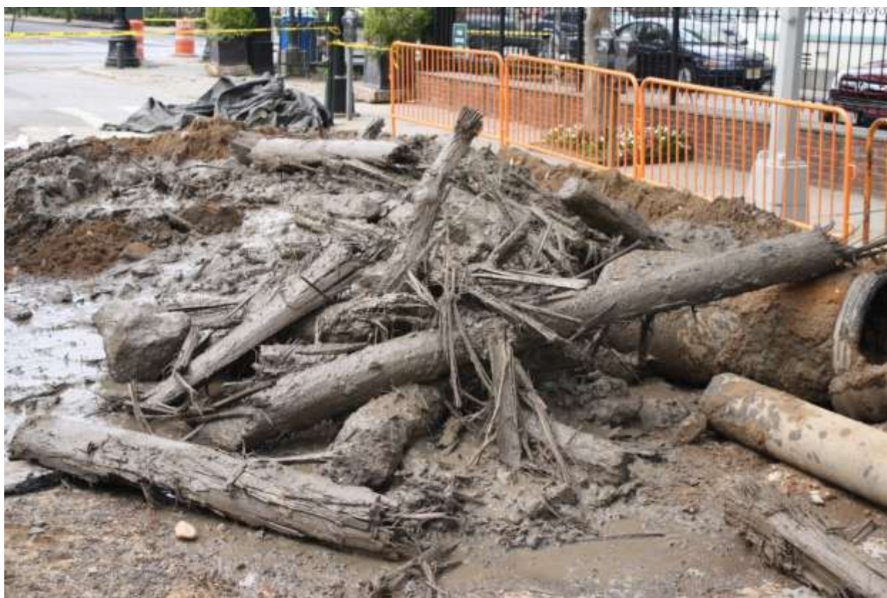
Image 33: Logs removed from the catch basin trench on Water Street north of Old Fulton.
