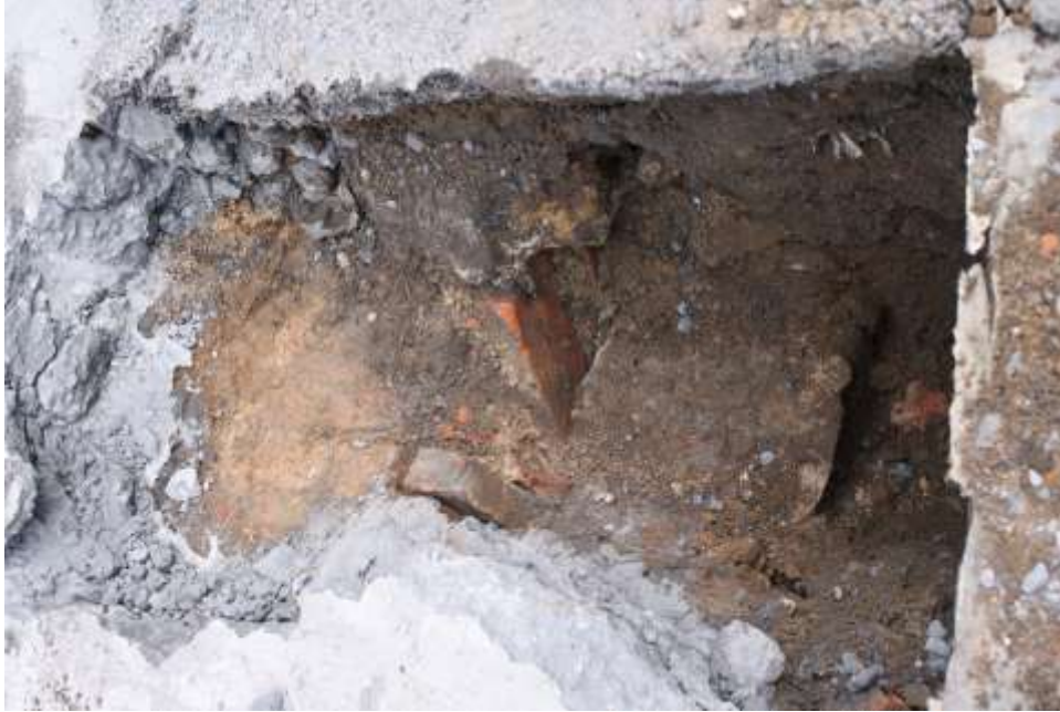
Image 94. Top of Pete's sidewalk vault (Old Fulton, N side, 160' E)
