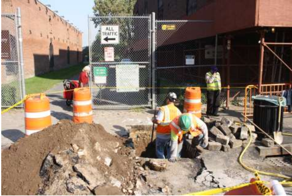
Image 126. Water St., Empire Fulton Ferry State Park driveway trench
