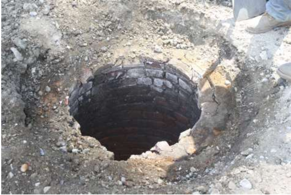
Image 72. Water and New Dock, old brick manhole
