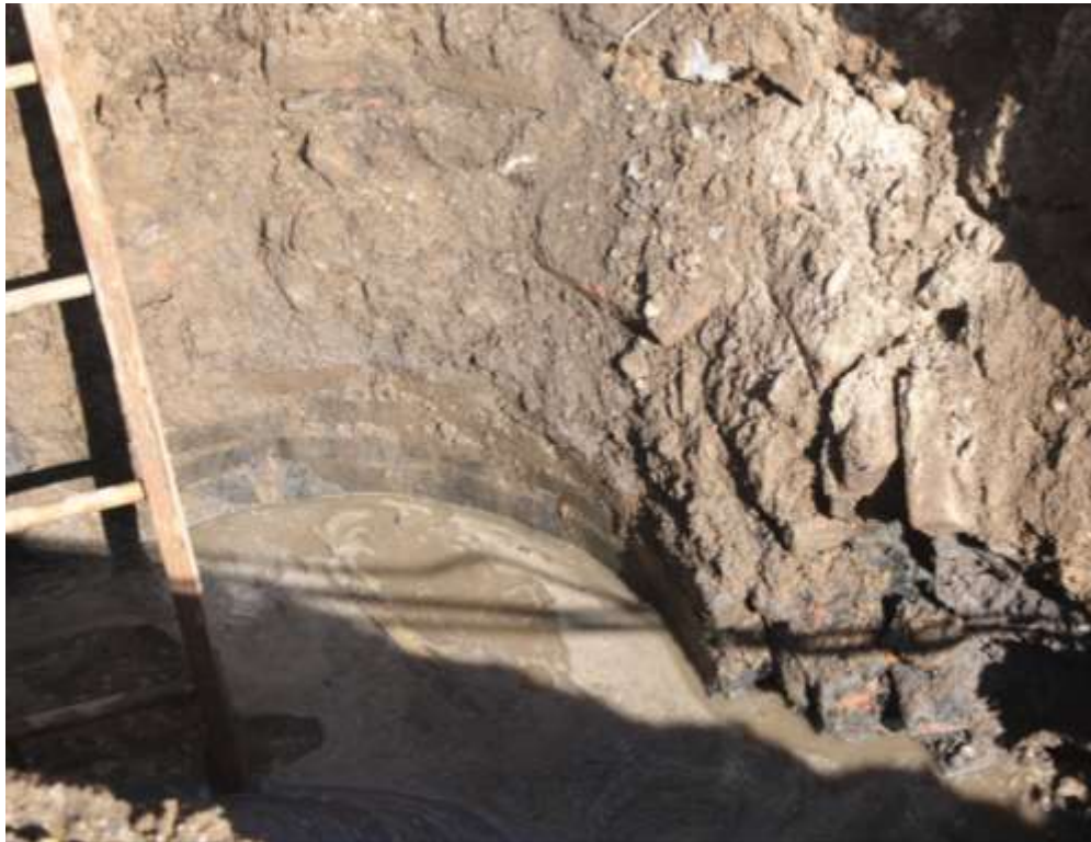
Image 40: Circular brick feature in catch basin trench on the north side of Water Street at Dock Street, looking north.
