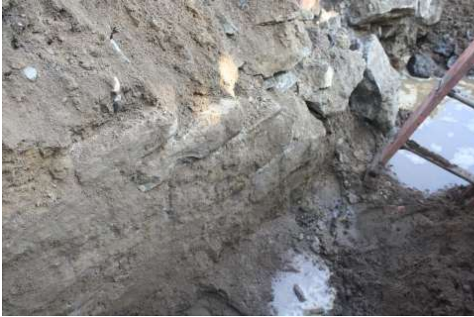
Image 23. SS Fulton, stone wall in fully extended trench (looking NW)— increased uniformity of stone is visible in this photo\
