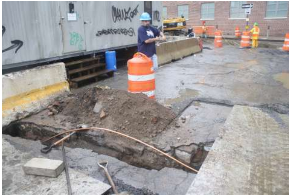
Image 83. Water St, New Dock St. trench, plan view
