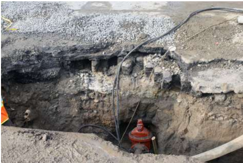
Image 38. SS Fulton, widened segment of trench with newly installed connection valve & S wall stratigraphy
