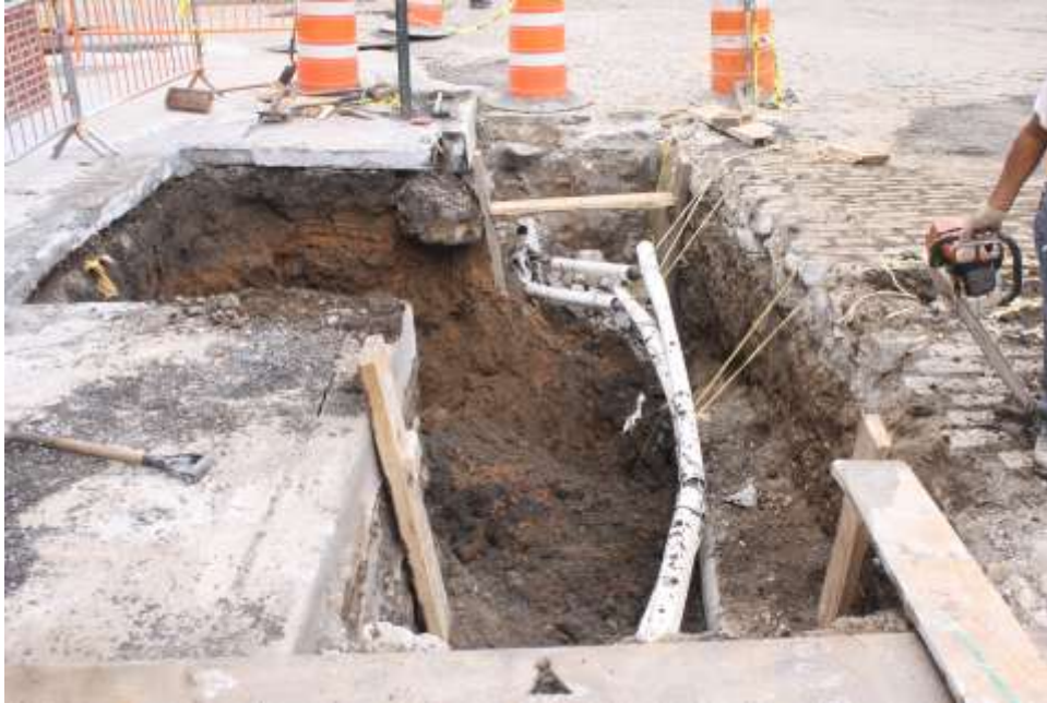
Image 108. Dock St., looking N at CB trench, W side of street
