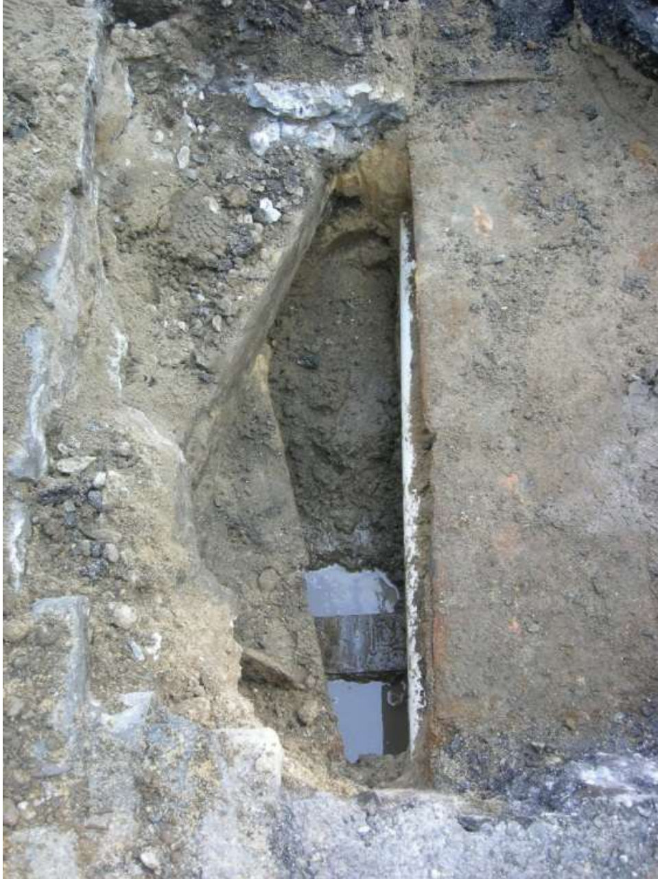
Image 31: Test Pit 8, looking north. A street car tie is present in the upper left corner (northwest) and a wooden utility duct is visible running from left to right in the lower center, beneath the white PVC duct.
