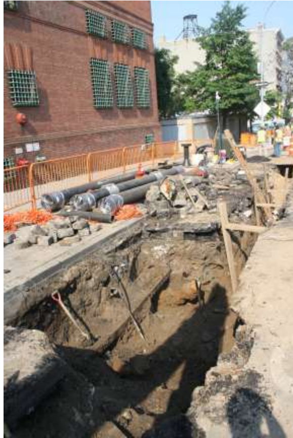
Image 35. SS Fulton, looking W, showing location of side trench relative to Elizabeth St.
