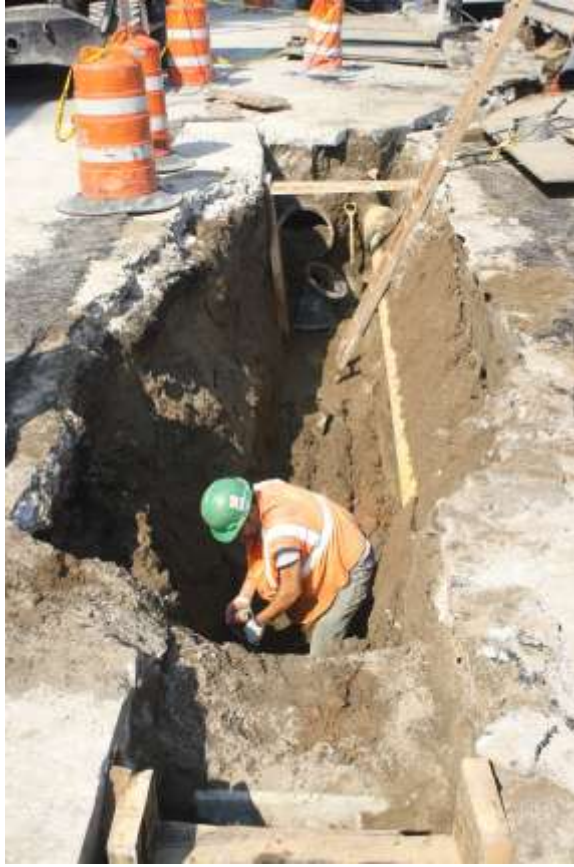
Image 80. Water St, where trench begins heading E at New Dock St.
