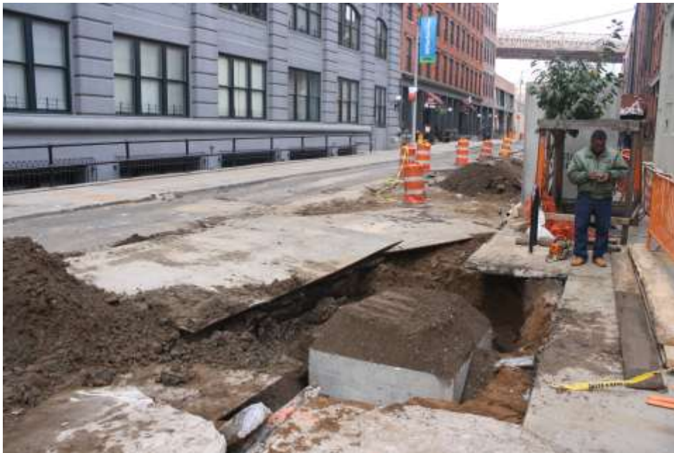
Image 115. Water St., 975' E, catch basin trench after completion
