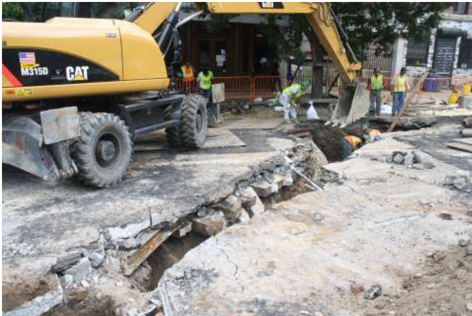
Image 51. NS Old Fulton, looking N, three rails and ties visible in W wall
