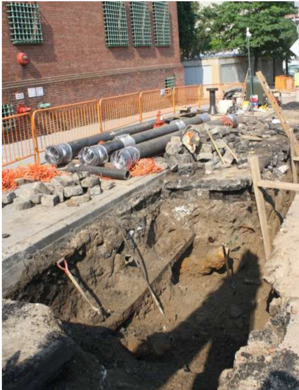
Image 13: Wood duct on Old Fulton Street by the Eagle Warehouse.
