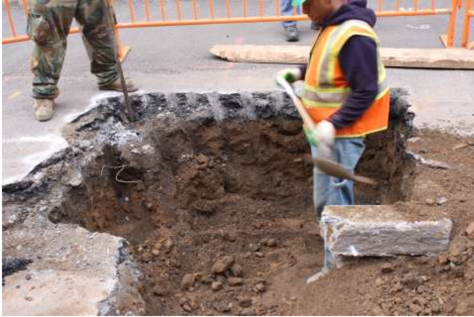
Image 128. Water St., S side, 675' E, excavating sidewalk
