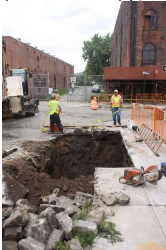
Image 103. Dock St. 10' S catch basin trench looking N
