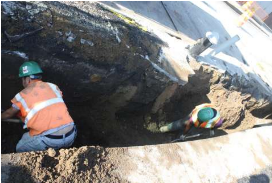
Image 75. Water/OF, test pit looking E
