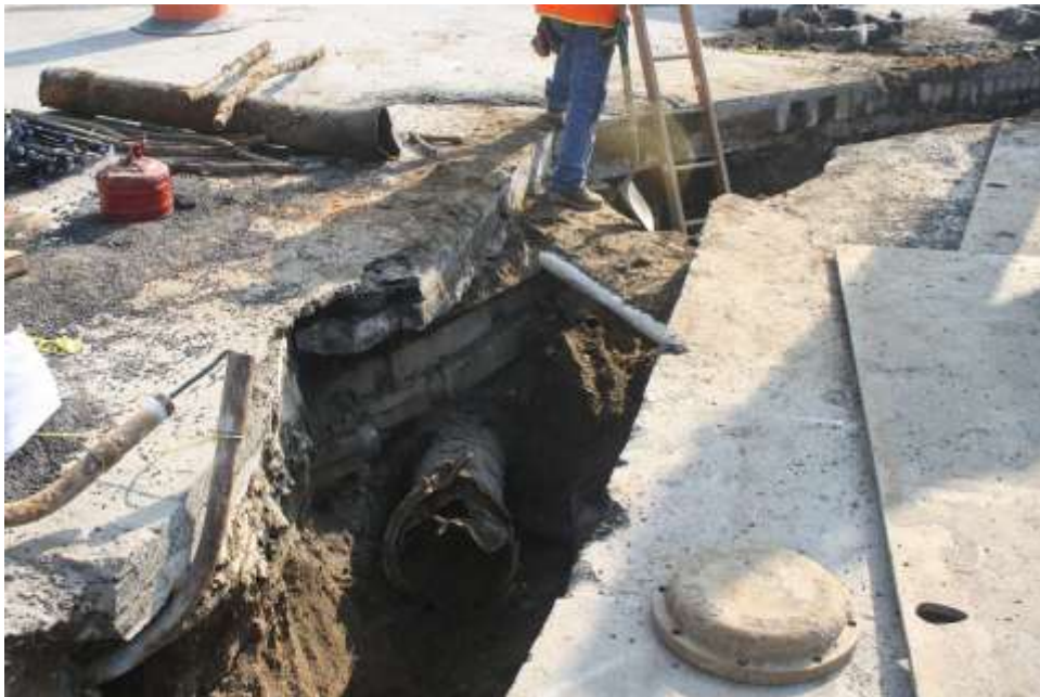
Image 59. OF trench, N side at turn to head E, 73', showing concrete conduits curving out of wall
