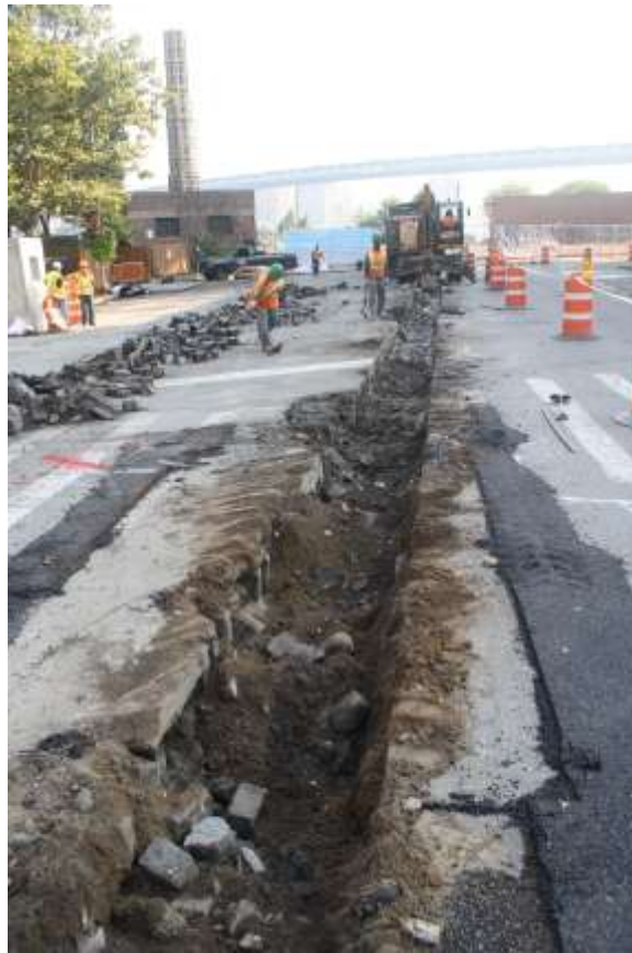
Image 63. Water Street trench plan view
