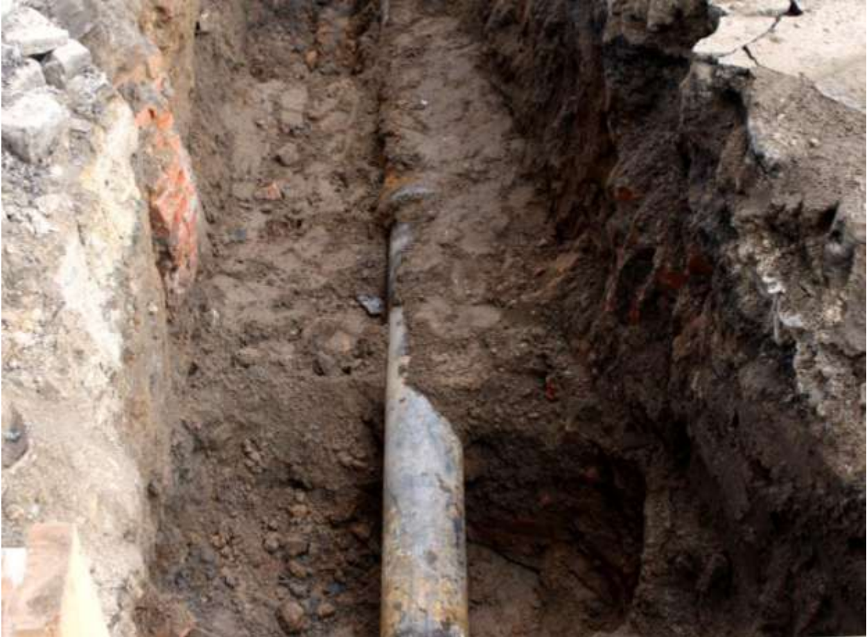
Image 39: Looking north in the New Dock Street trench at the remains of a brick wall, visible to each side and below right of the water main.
