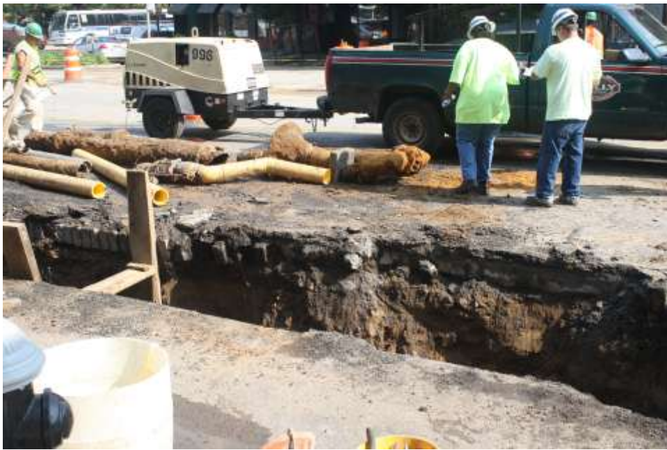
Image 30. SS Fulton, N wall of trench near intersection Elizabeth showing widened trench with no CS
