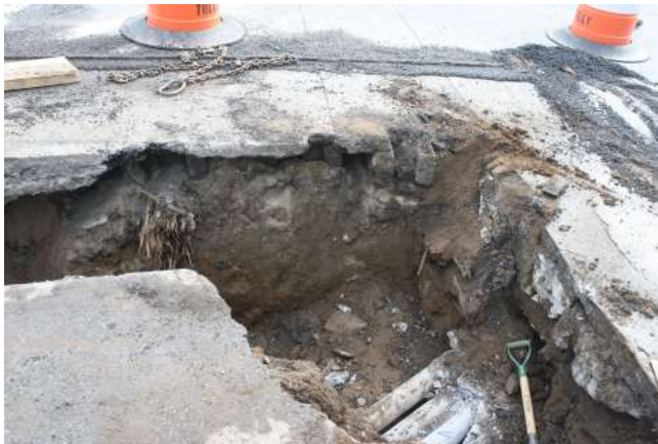
Image 6. Furman St, N end of Furman trench showing both wood pieces
