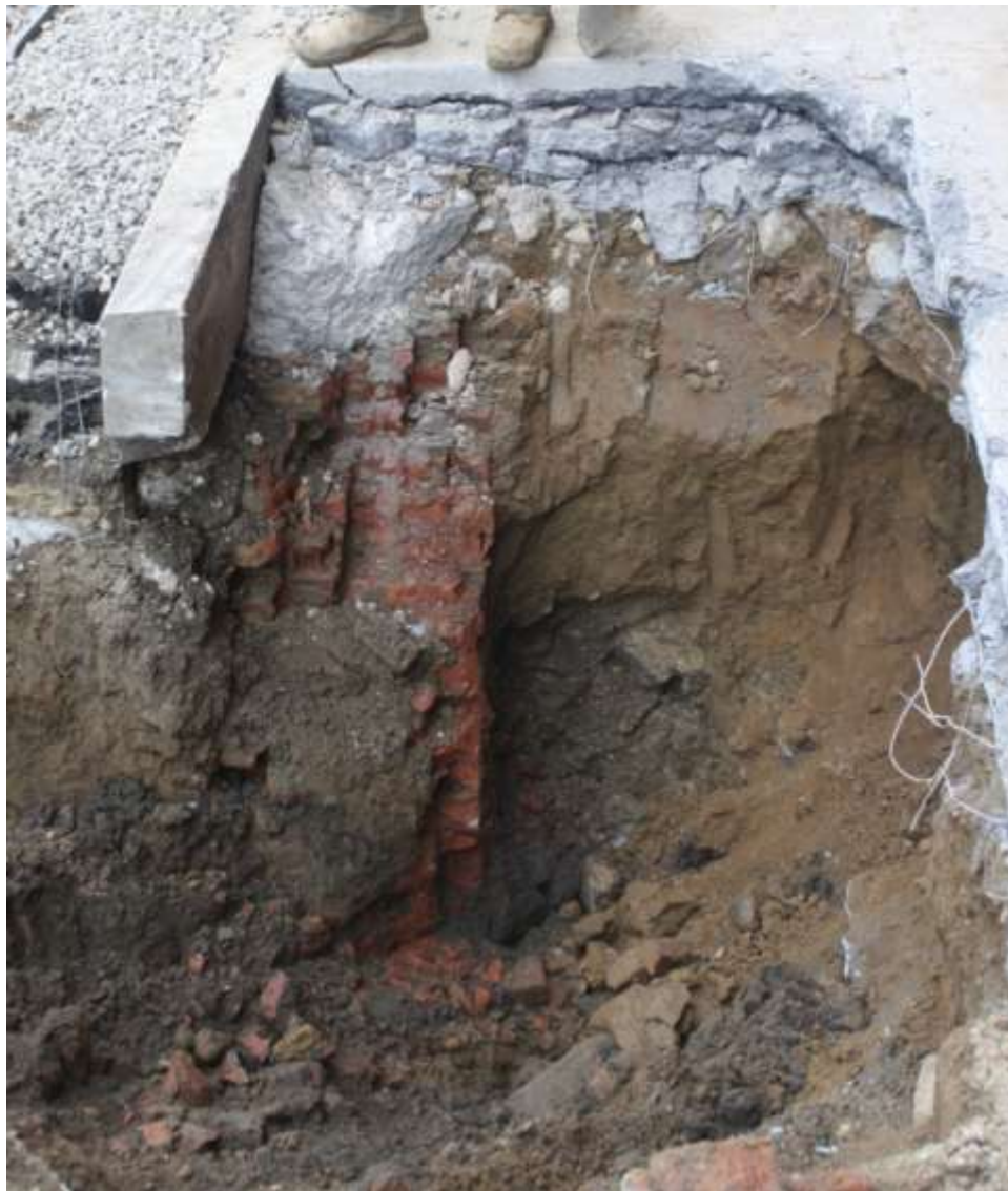
Image 19: Brick wall on Old Fulton Street west of Front Street, looking east.
