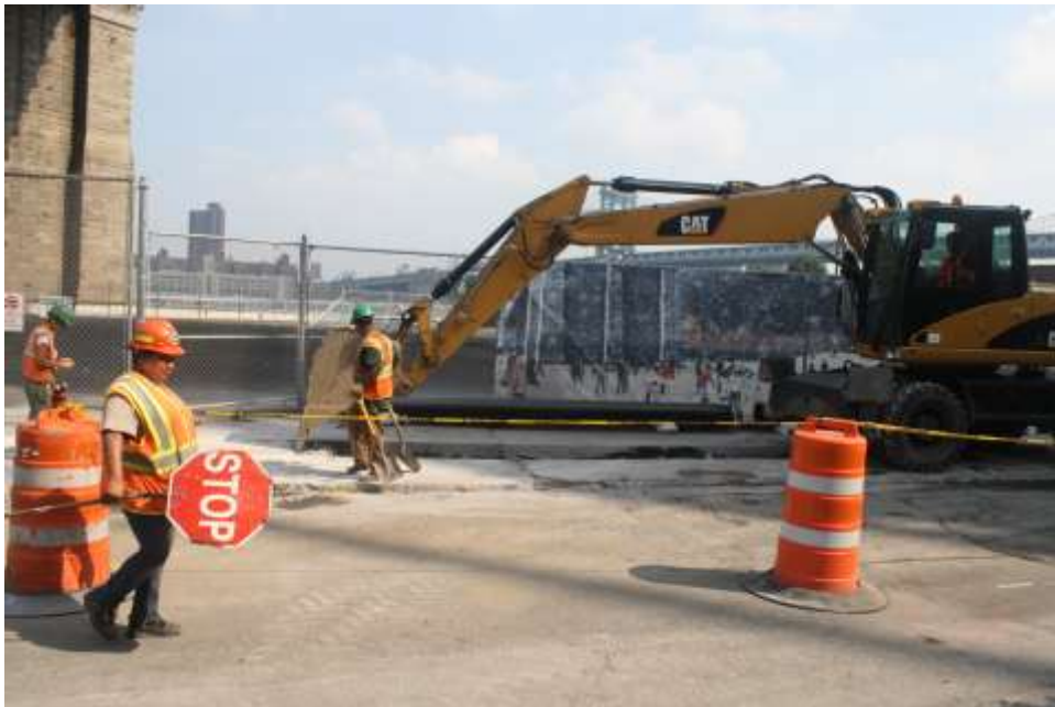
Image 69. Water St., location of sidewalk trench
