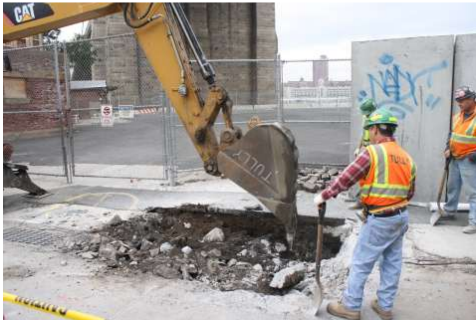
Image 97. Water St/Purchase Bldg lot trench for catch basin – looking NW, showing location
