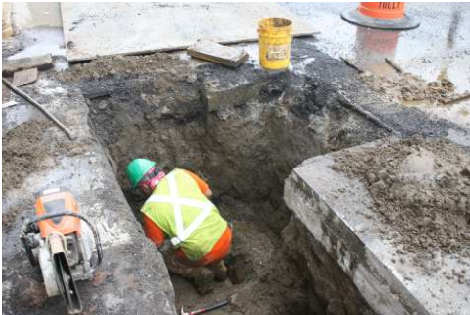
Image 4. Furman St, S end of Furman trench
