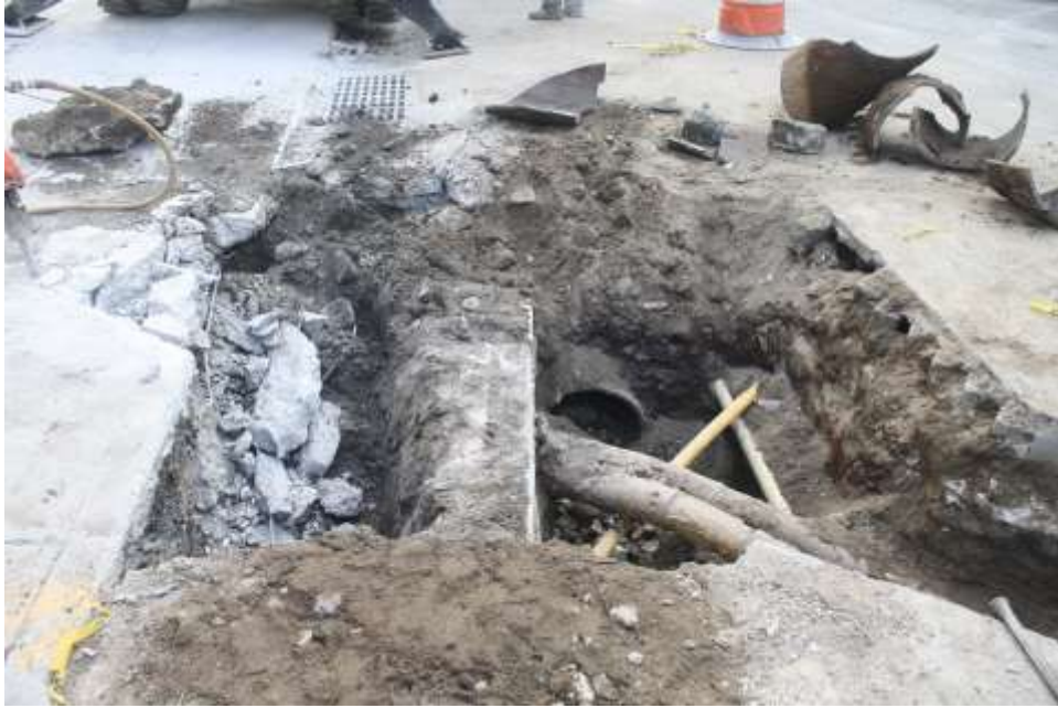
Image 68. Water St., utilities in N end of trench
