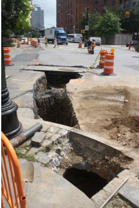
Image 78. OF/Water St, looking E, sidewalk segment visible in foreground
