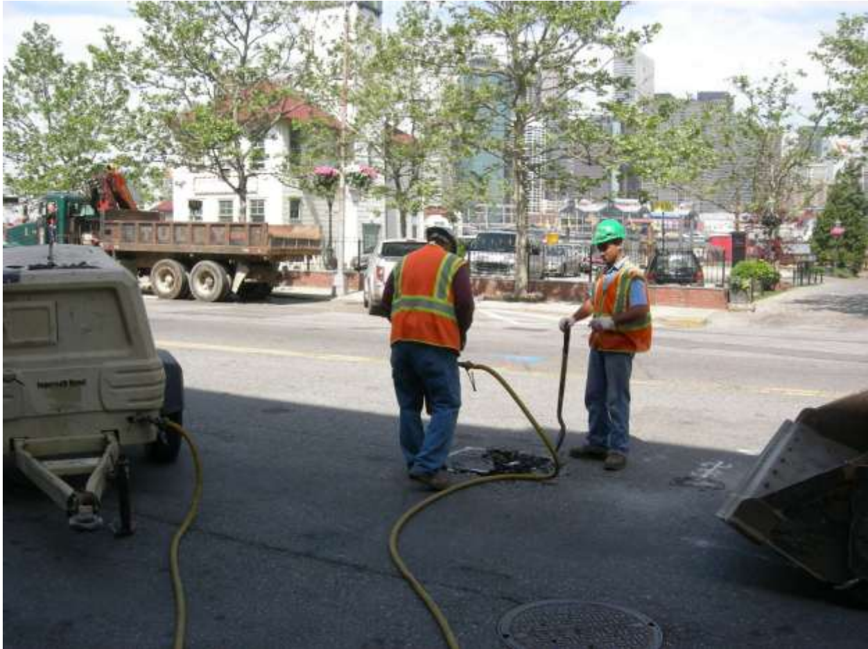
Image 02: Initial Test Pit work in 2009 – Fulton Ferry Landing area
