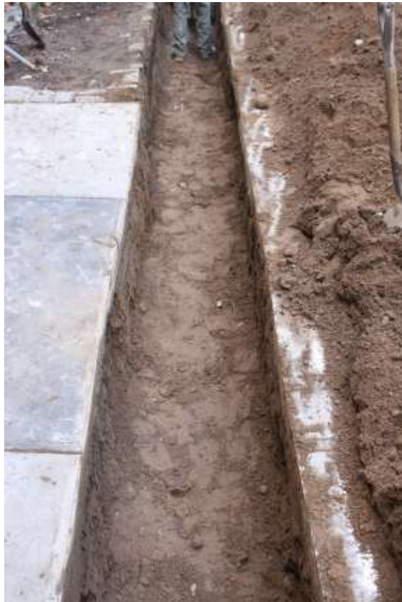
Image 135. Water St., Main St. sidewalk plan view, fire cable trench looking N
