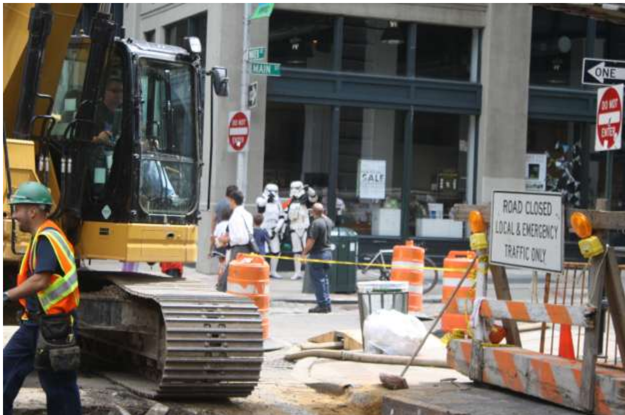
Image 09: Due to its location and site conditions there were several government inspectors on site at any given time.
