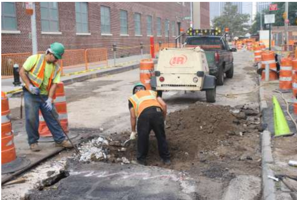
Image 107. Water St. 475' E beginning excavation (looking W)
