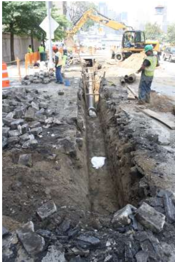
Image 32. SS Fulton, looking W along OF trench at end of excavation for the day
