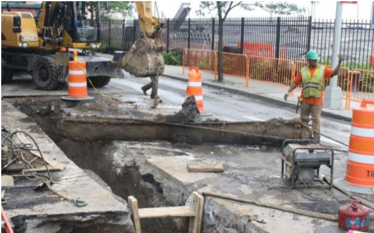
Image 12: Cast iron water main laid in the 1890s being removed from Furman Street.
