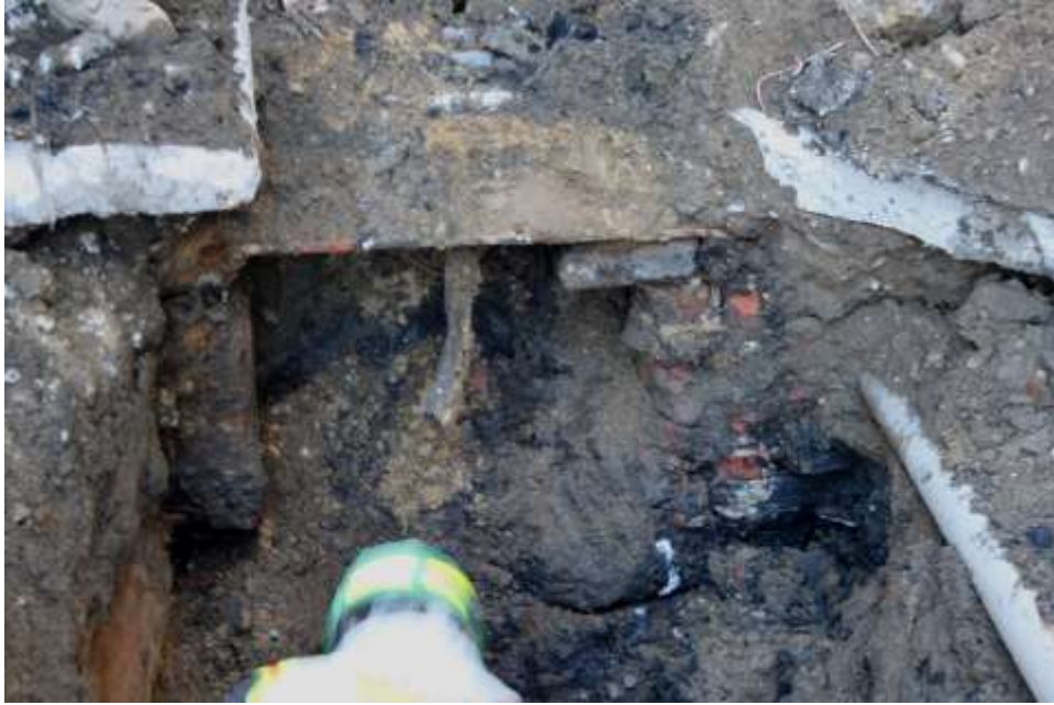
Image 122. Water St., E of Main St., brick trench in E wall of CB trench
