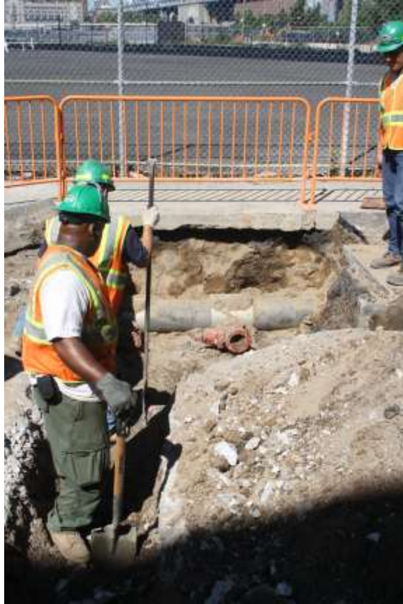
Image 90. Water St., hand digging extension of Water St. 175' E
