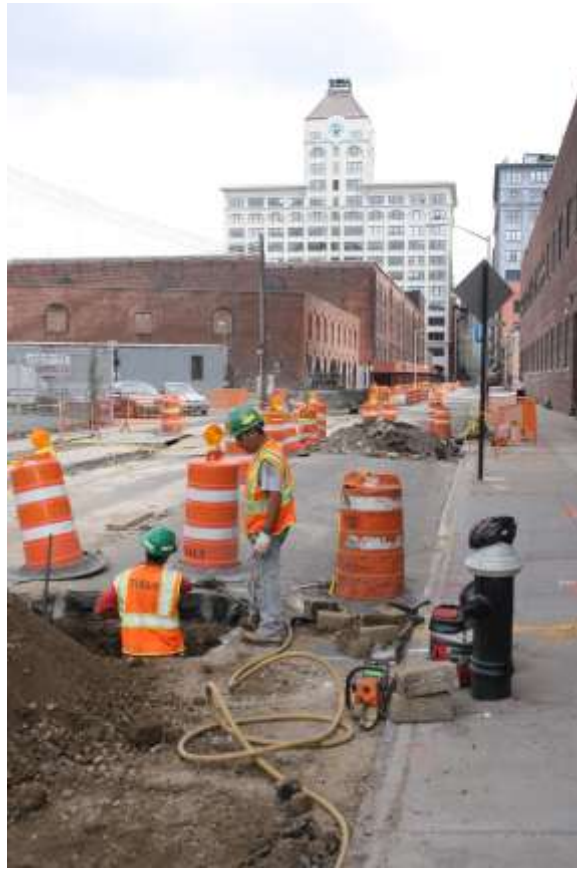
Image 96. Water St, looking E showing 175' E and 245'E trenches
