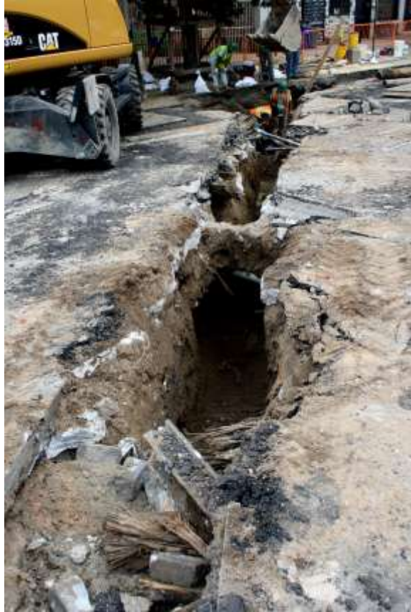
Image 52. NS Old Fulton, looking N, entire section of trench
