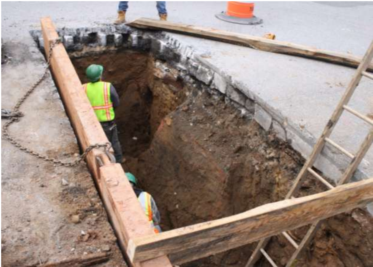
Image 20: Brick footing in sewer trench on Old Fulton Street, looking southwest.
