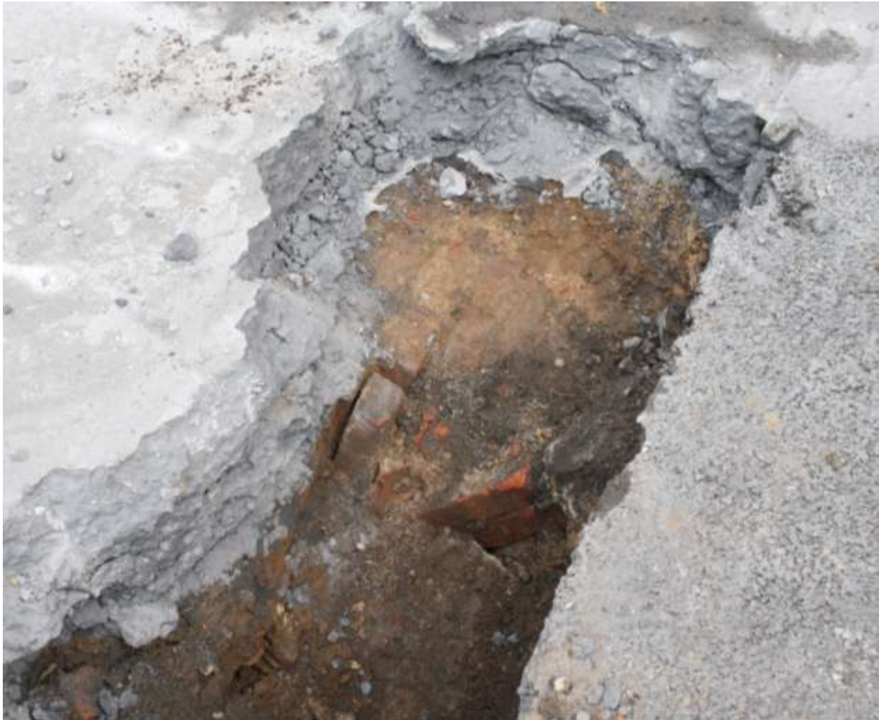
Image 28: Top of sidewalk vault in front of No. 2 Water Street, on the south side of the building.
