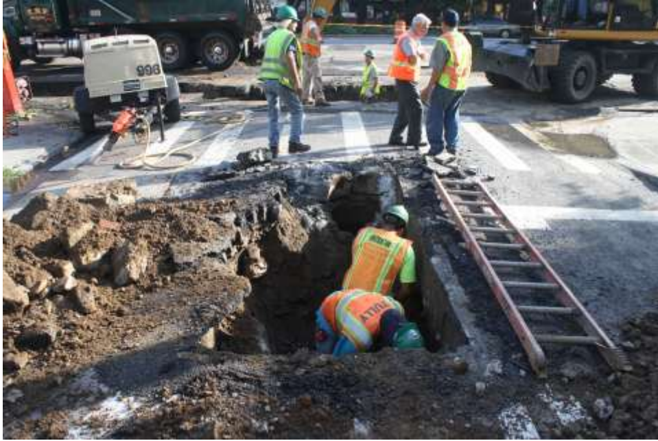
Image 21. SS Fulton, excavating Everit trench in area where wall was found
