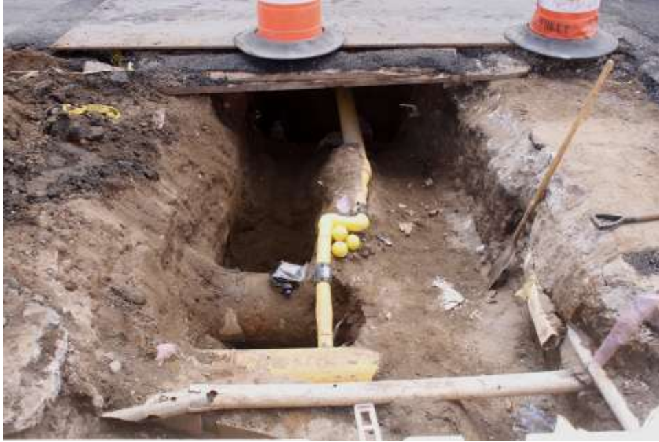
Image 100. Water St. 175' E, looking S, showing areas of excavation below existing utilities
