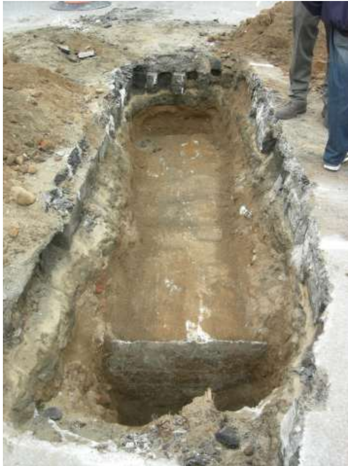
Image 10: Concrete sewer housing in Test Pit 2.
