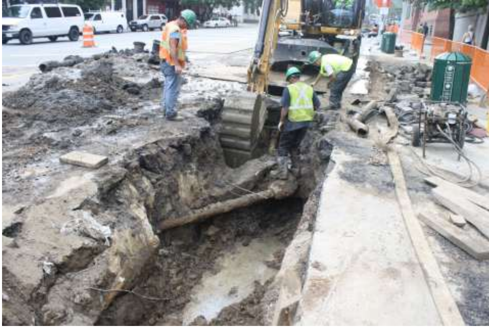
Image 27. SS Fulton, looking E, view of utilities including first concrete casing
