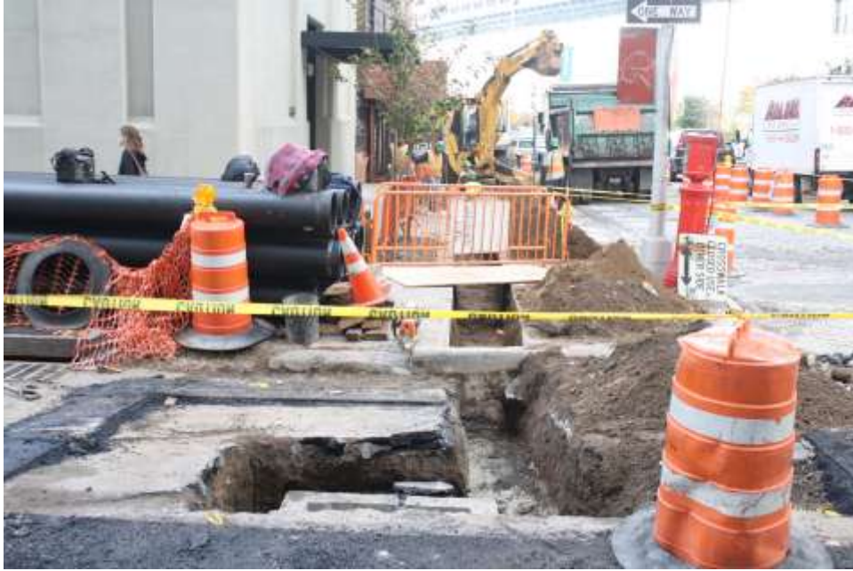
Image 134. Water St., fire cable trench on Main St (sidewalk), looking N from Water
