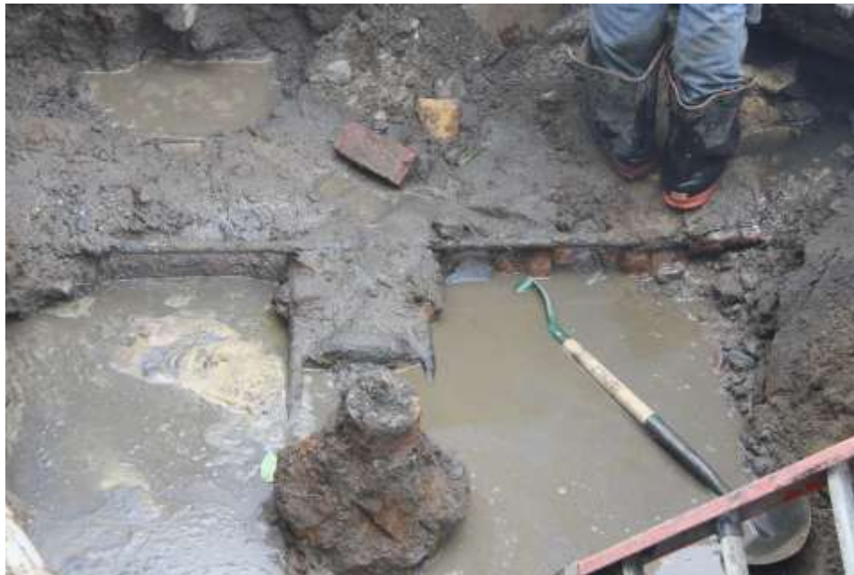
Image 8. Furman St, junction of Furman and OF trenches looking W from OF; part of 1890s water main system, brick supports underneath
