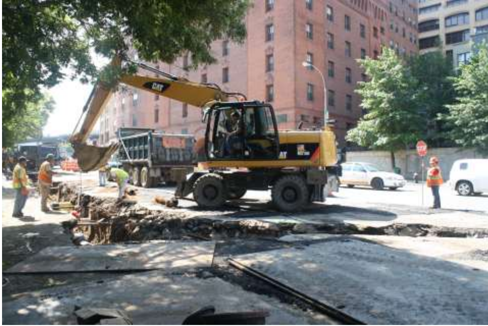
Image 50. NS Old Fulton, wide angle showing first turn in trench
