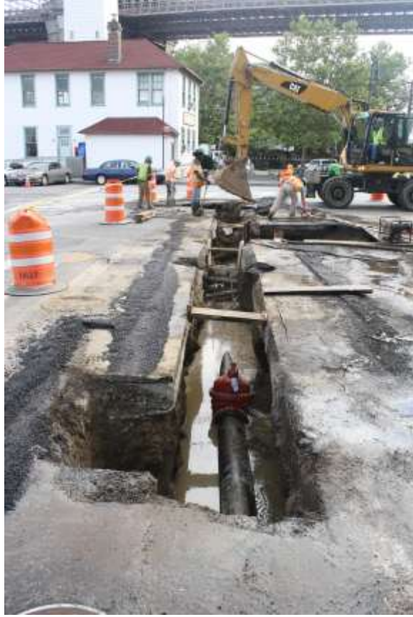
Image 9. Furman St, looking N along trench, new main visible in S end
