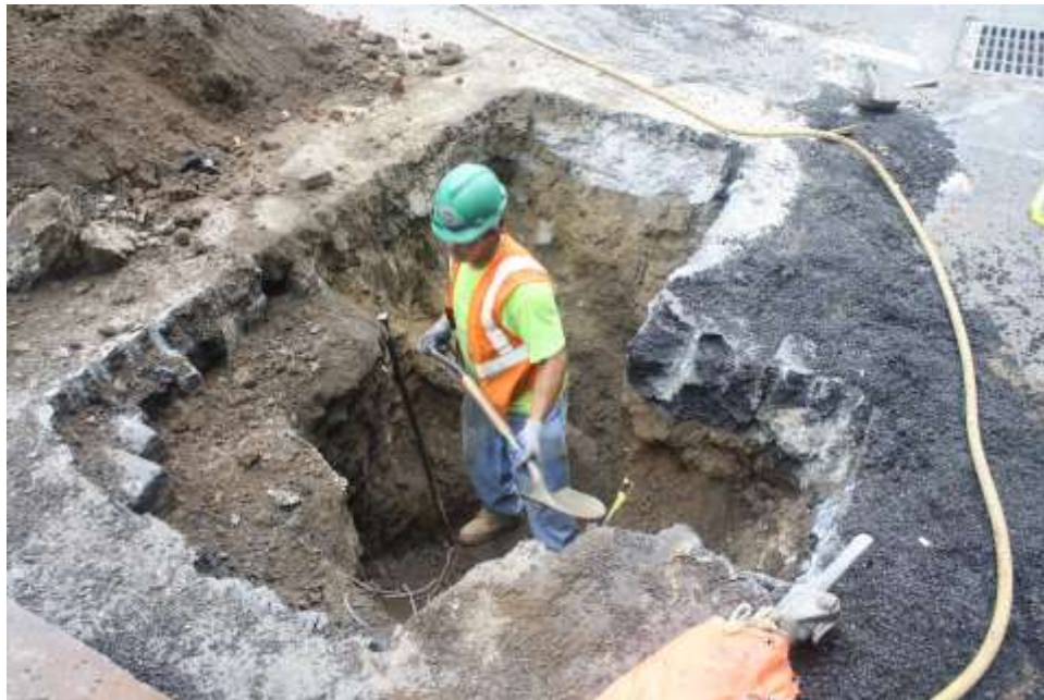
Image 57. Old Fulton, excavation pit with extensions
