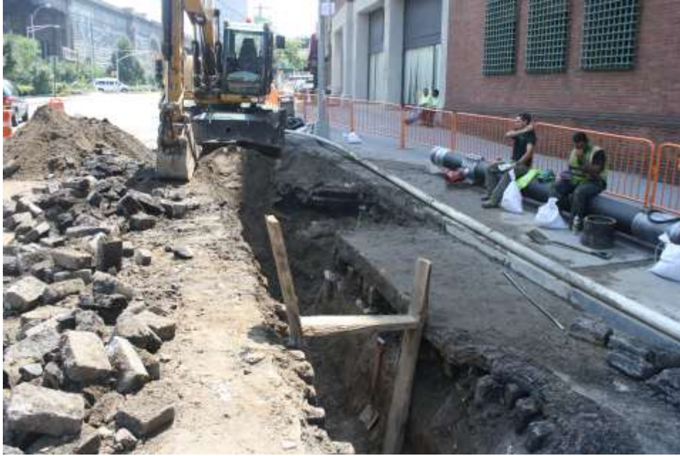
Image 37. SS Fulton, looking E showing location of side trench #2
