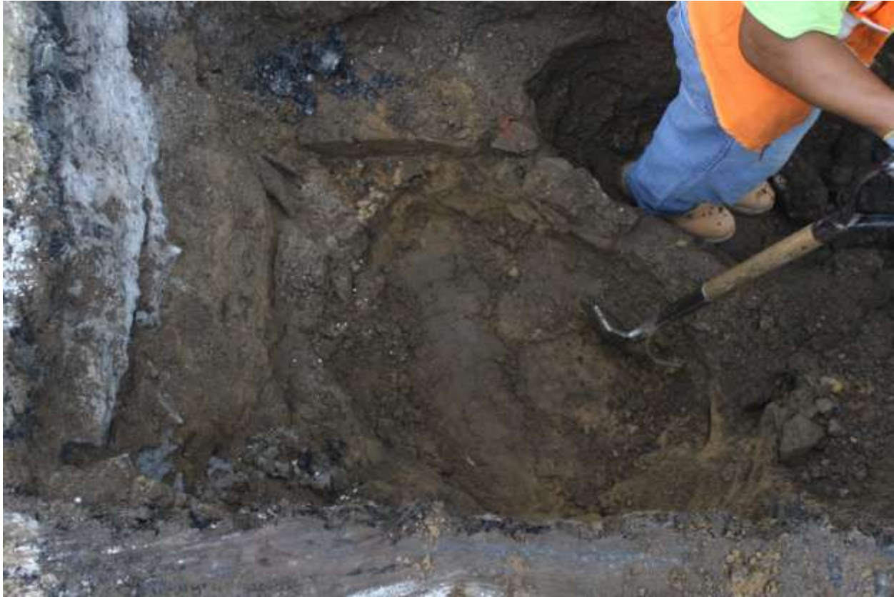
Image 26: Bottom of circular brick feature in southwest corner of test pit one on Old Fulton Street east of Water Street.
