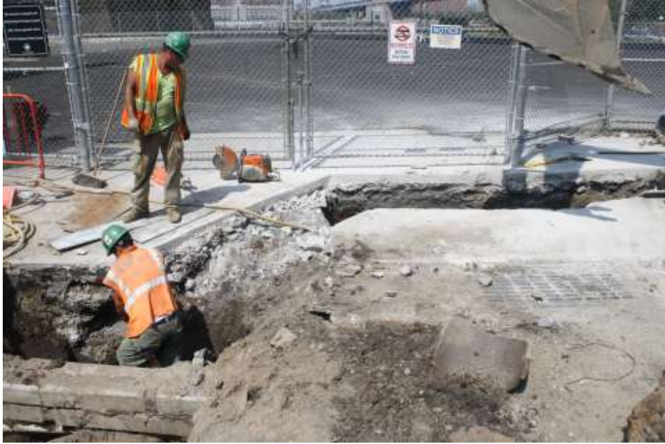
Image 70. Water St., sidewalk trench connecting to street trench
