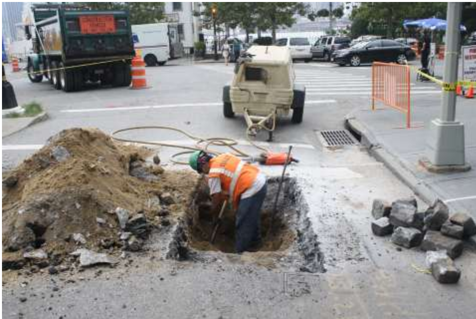
Image 55. Test pit at OF and Water
