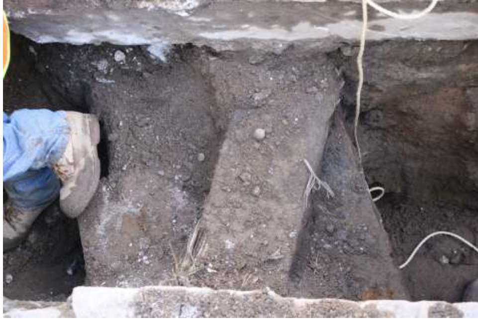
Image 132. Water St., rail tie with metal plate in trench
