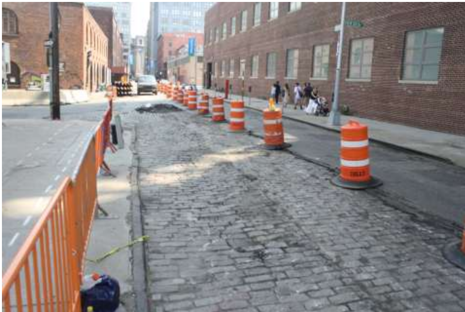
Image 61. Water St, cobblestone surface after asphalt removed
