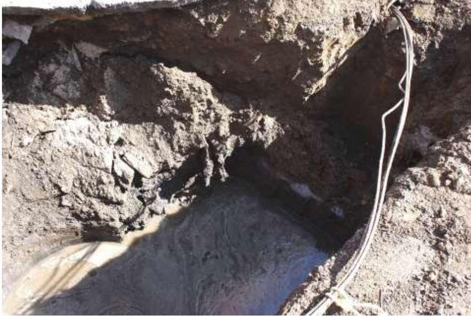
Image 112. Water St., brick, wood, and concrete in Water St. CB trench (looking NE)
