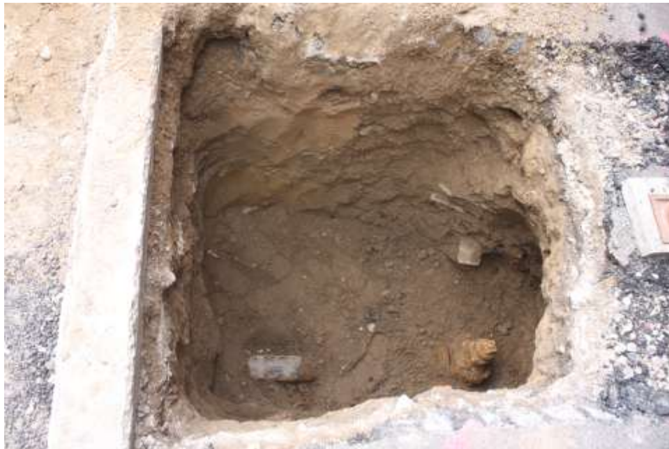
Image 117. Water St., sidewalk trench in Water 745' E
