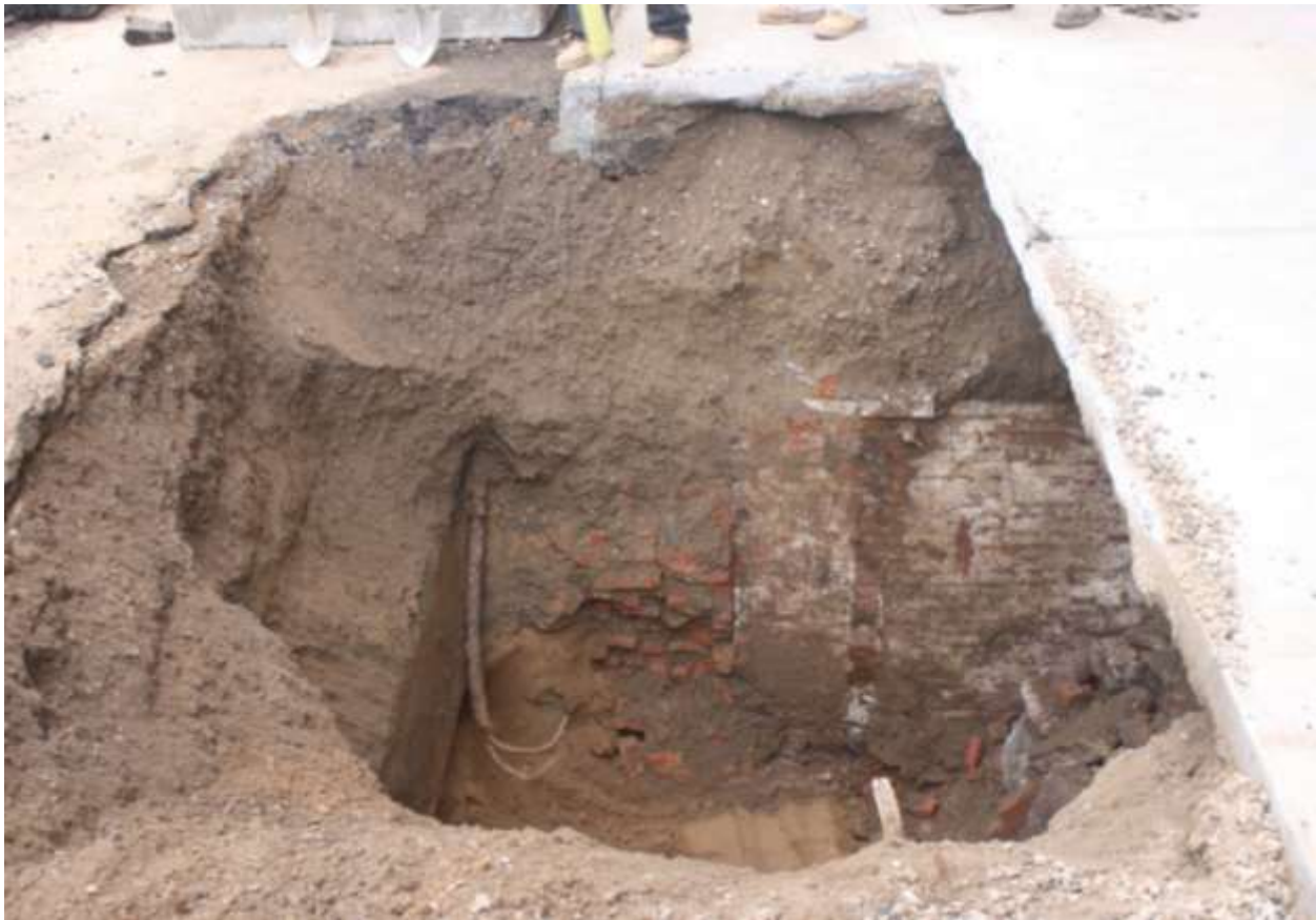
Image 17: Sidewalk vault in front of the Eagle Warehouse, looking east.
