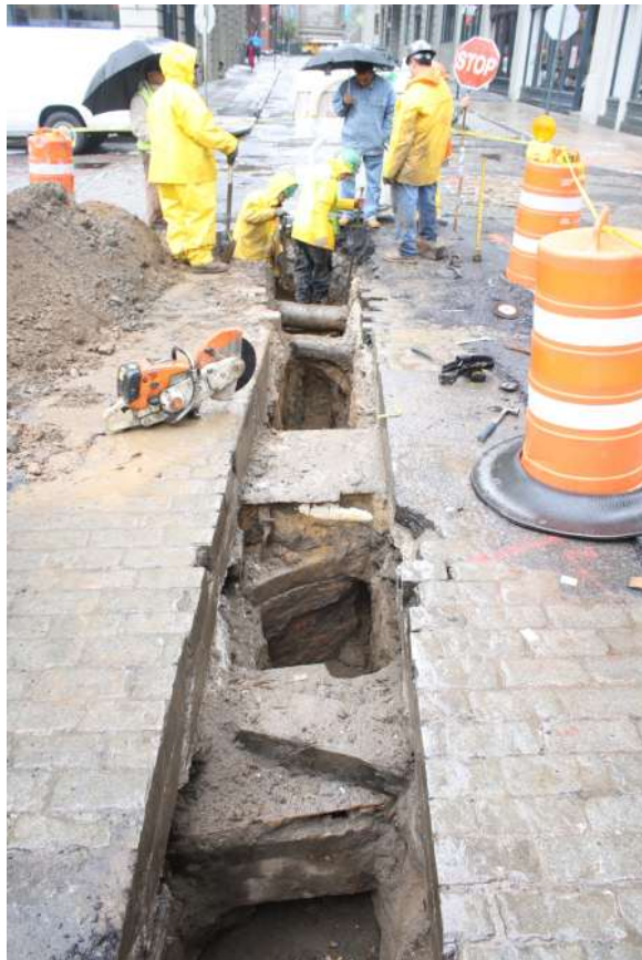
Image 131. Water St. series of street car ties in trench, W of Main St intersection
