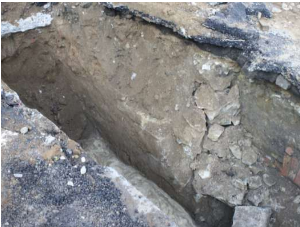
Image 22: Rough-cut, mortared stone wall adjacent to dry fieldstone wall and brick structure.
