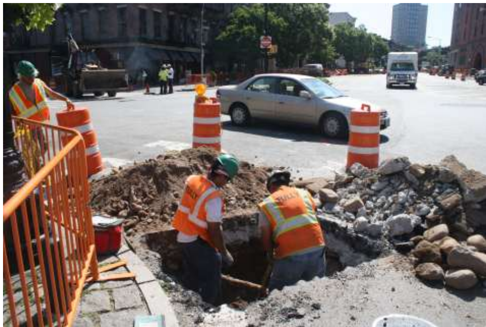
Image 45. NS Old Fulton, location of excavation pit, looking NE
