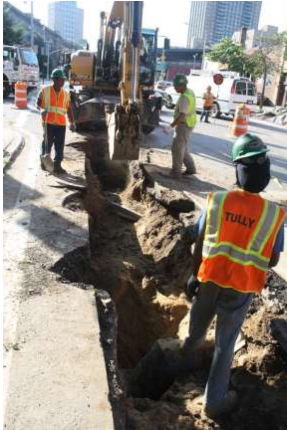
Image 44. NS Old Fulton, extending the E end of the trench
