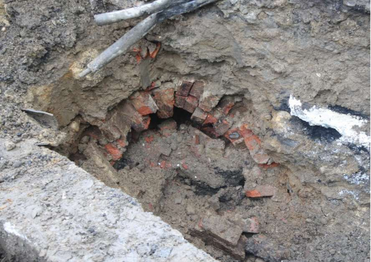
Image 16: Brick sewer on Old Fulton Street west of Everit Street.
