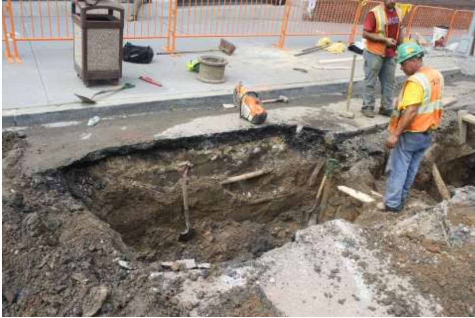
Image 39. SS Fulton, E end of trench (metal utility pipes in S wall visible)
