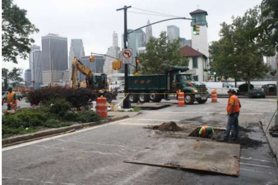
Image 56. Old Fulton, Overall plan view showing two locations of excavation
