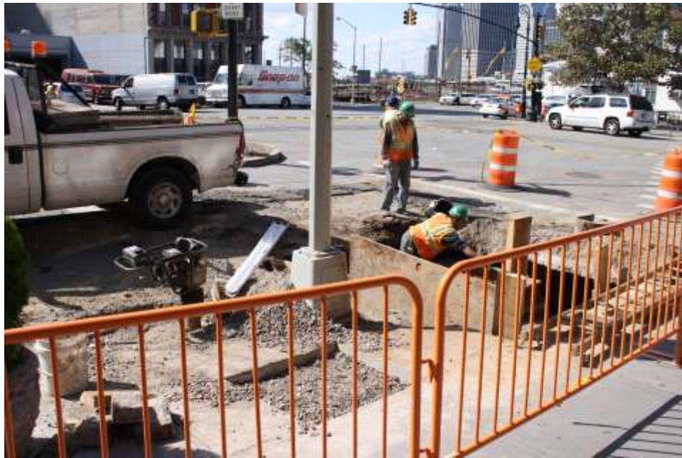
Image 119. Old Fulton, 148' E, looking SW, showing location of 2 smaller trenches
