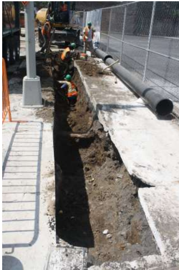
Image 71. Water St., sidewalk trench looking W
