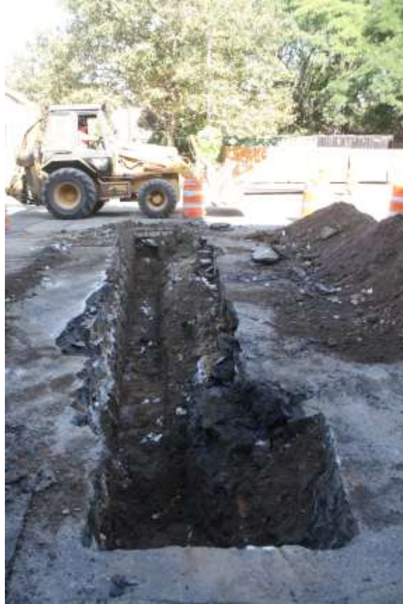
Image 86. Water St., 70' N of OF, 7' W of curb
