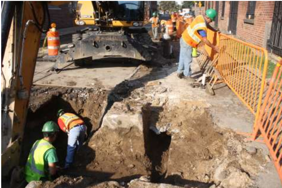
Image 109. Water St. Empire Fulton Ferry Park entrance catch basin trench, looking W
