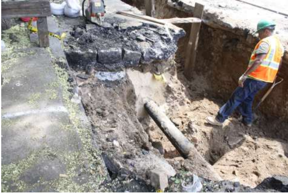
Image 46. NS Old Fulton, E wall of side trench showing sand fill around large utility pipe
