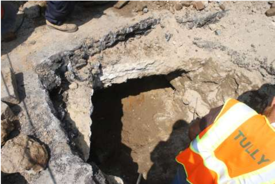
Image 79. River Café trench looking under W wall
