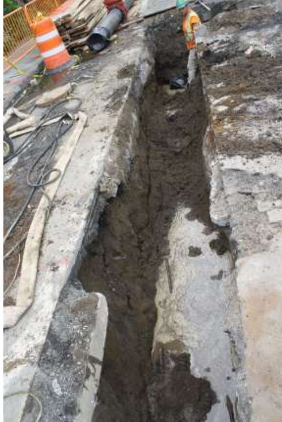
Image 7. Furman St, trench looking S after removal of old main
