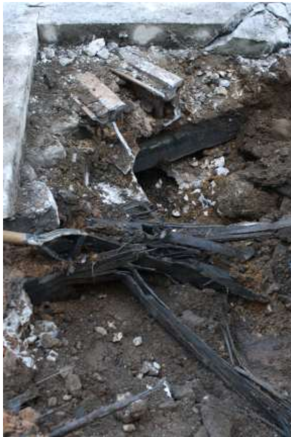
Image 121. Water St., E of Main St. catch basin looking N after tracks partially removed. Note creosote-soaked wood ties and concrete base under rails.
