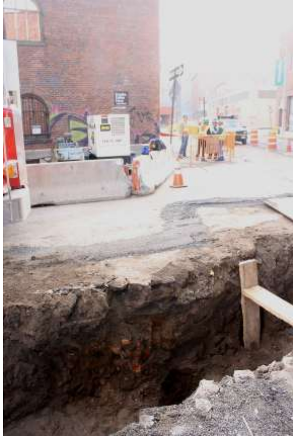
Image 124. Water Street, E wall profile of New Dock St. trench
