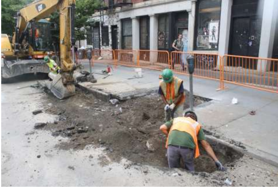
Image 92. NS Old Fulton, beginning catch basin trench, 310' E. Looking NW
