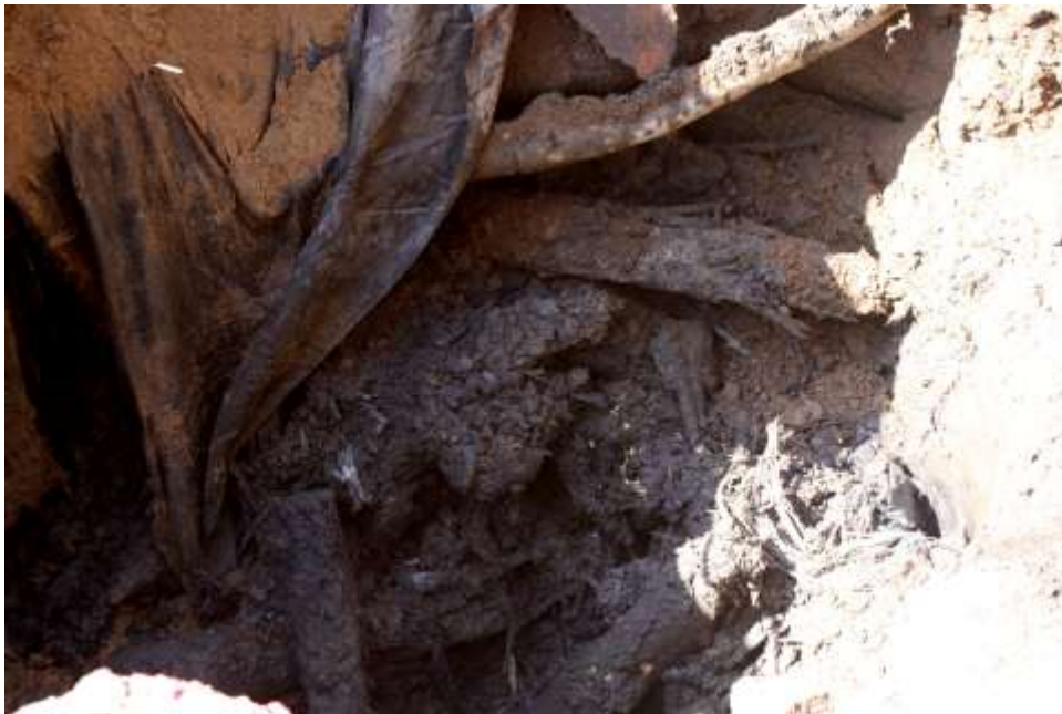
Image 113. Water St., wood in bottom of CB trench (E of park entrance)
