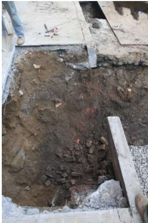
Image 40. SS Fulton, W wall of sidewalk trench, brick visible at curb
