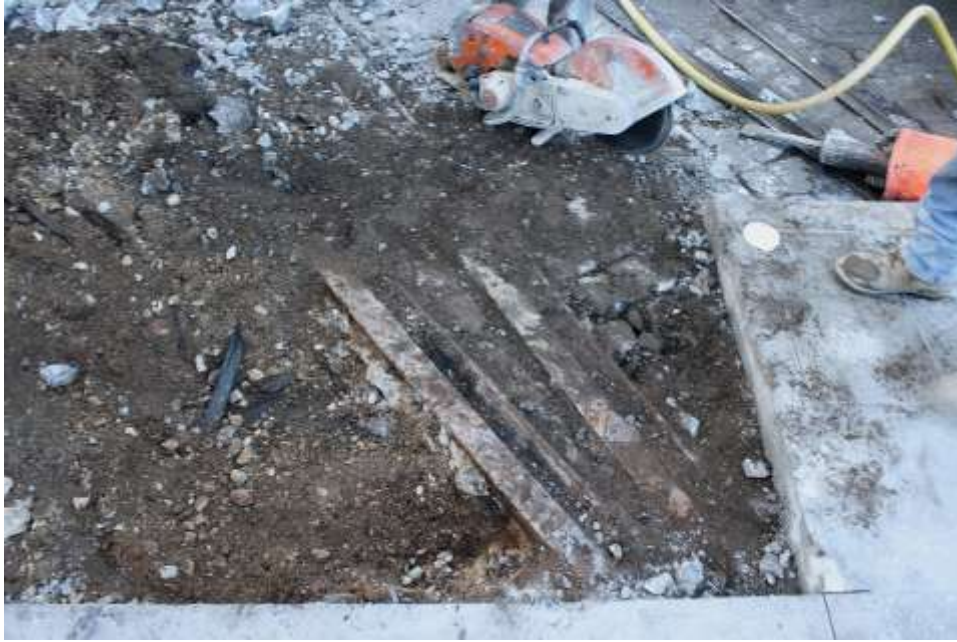
Image 120. Water St., 20' E, near Main St, trolley tracks under sidewalk
