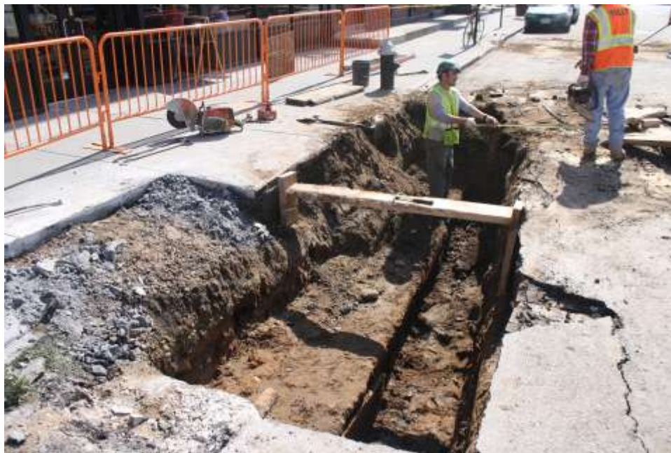
Image 99. Water St./Ignazio's trench showing trench location and concrete plating over electrical (looking S)
