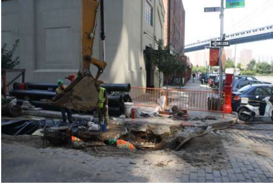
Image 88. Water St., E end Water St. trench at Main St. looking N
