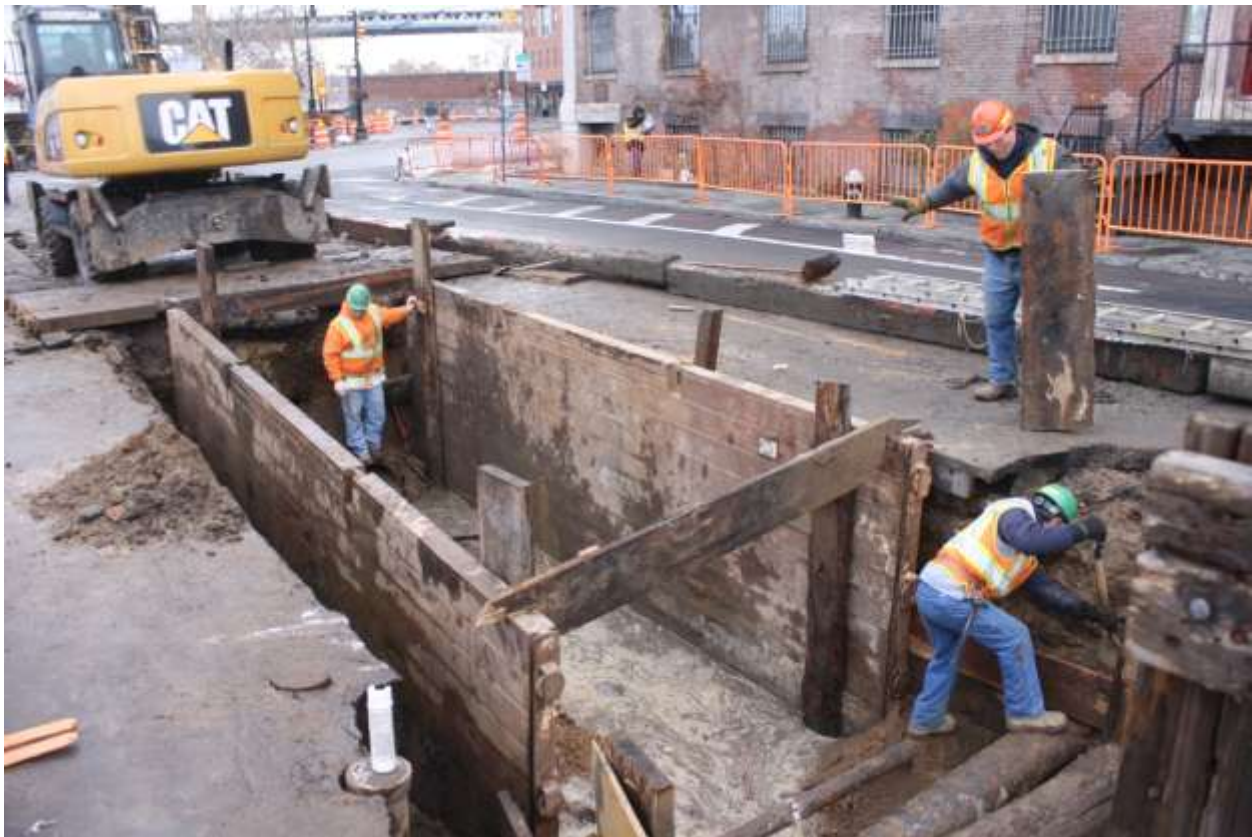
Image 06: Example of mechanical and hand excavation.
