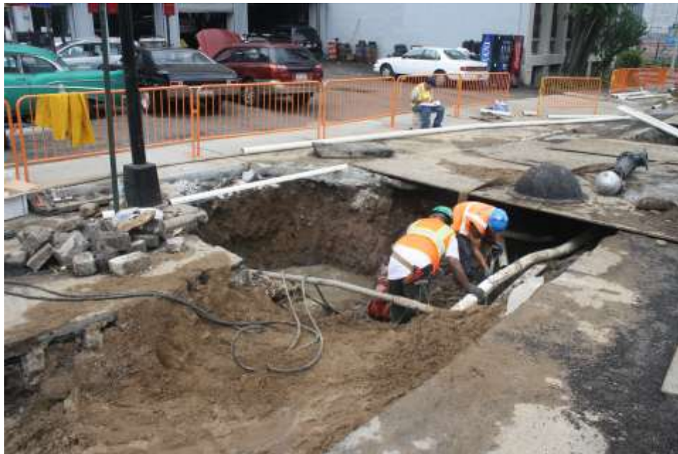
Image 26. SS Fulton, wide angle view of hydrant trench
