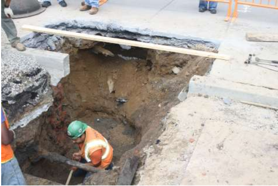
Image 41. SS Fulton, looking at S wall of sidewalk trench from N side OF trench, PVC pipe and wood visible
