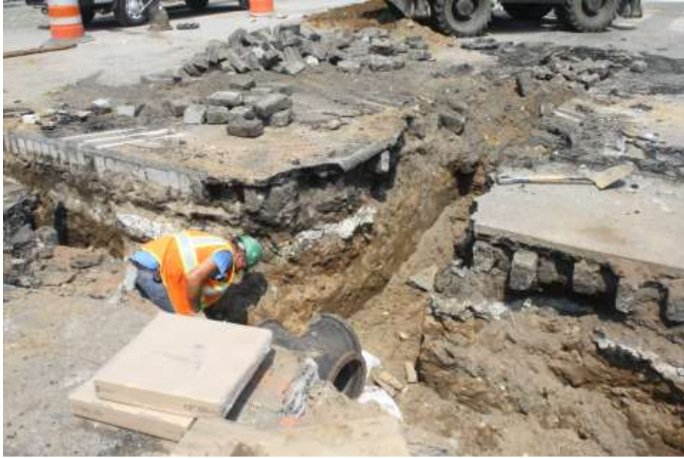
Image 62. Water St trench branching off of OF trench
