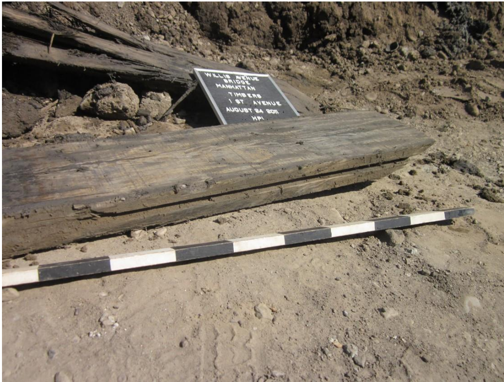
Photograph 26: (9/30/11 memo) First Avenue, one of the upright planks from the bulkhead. Note tongue and groove construction and beveled base.
