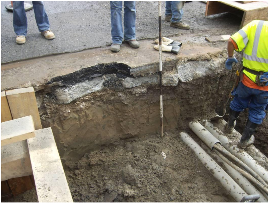
Photograph 20: (9/8/11 memo) First Avenue, Utility Trench 2/2 – 2/3, facing northeast to north wall. Note electrical lines at .7m below grade at right.
