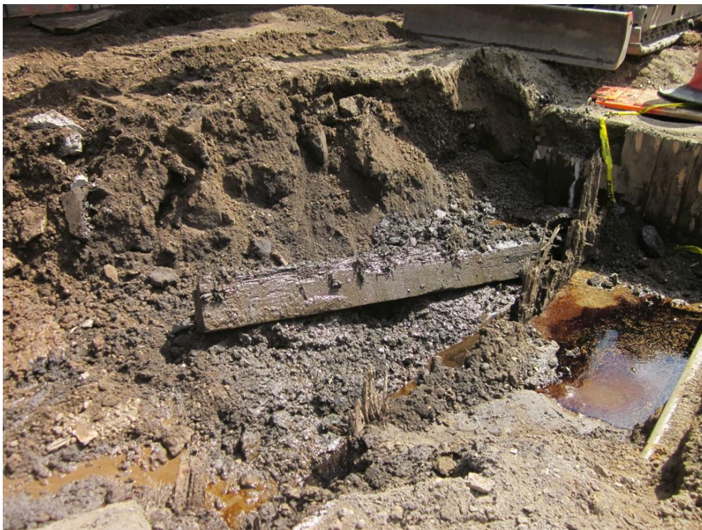
Photograph 25: (9/30/11 memo) Remains of former bulkhead at intersection of First Avenue and access road, looking north. Tops of upright planks have been sheared off. Oily water can be seen at right.
