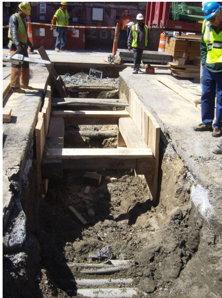
Photograph 19: (9/8/11 memo) First Avenue, Utility Trench 2/2 – 2/3 facing west. Utility lines are visible in foreground and at center of photograph. Shoring walls is in progress.
