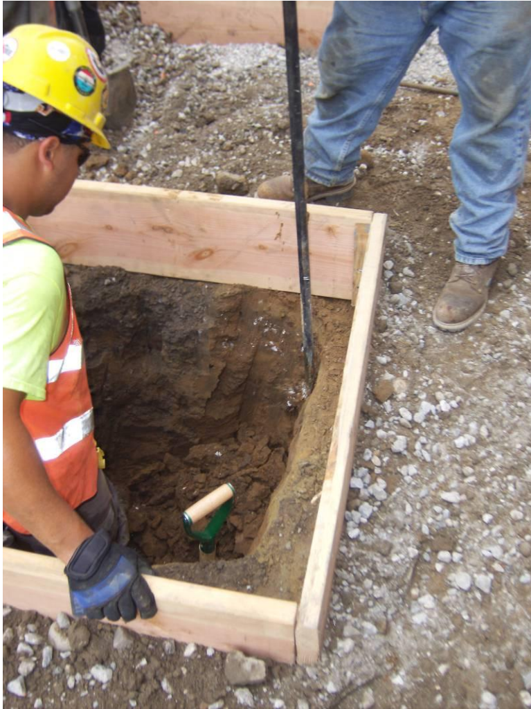
Photograph 36: (9/8/11 memo) East 127 th Street, excavating for lamp post installation.
