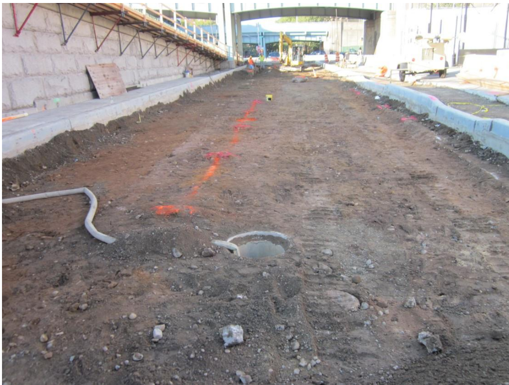
Photograph 29: (9/30/11 memo) First Avenue looking south, from intersection at East 126 th Street. Orange paint shows location of large gas main.
