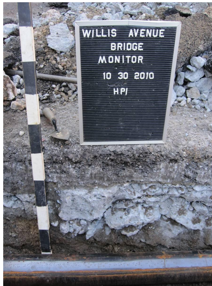
Photograph 6: (11/1/10 memo) First Avenue, south profile of hand-excavated utility trench. Note the multiple levels of blacktop and concrete above ash fill, and final installation of 4" iron utility pipe.
