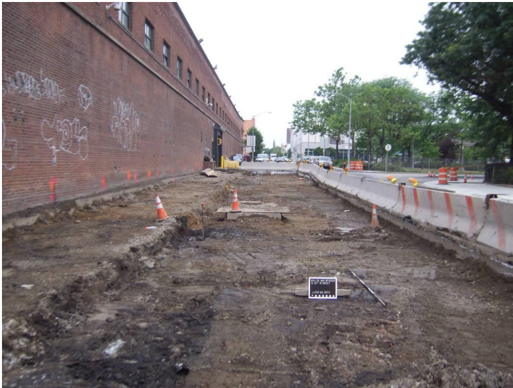
Photograph 42: (9/8/11 memo) East 127 th Street, view looking west following the removal of the southern sidewalk, curb, and south lane roadbed.
