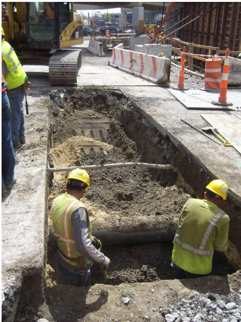
Photograph 18: (9/8/11 memo) First Avenue, Utility Trench 2/2 – 2/3 facing east. Water main in foreground and telephone conduit at center of photograph.
