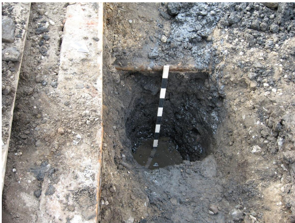
Photograph 8: (12/1/10 memo) First Avenue, Sono tube excavation.
