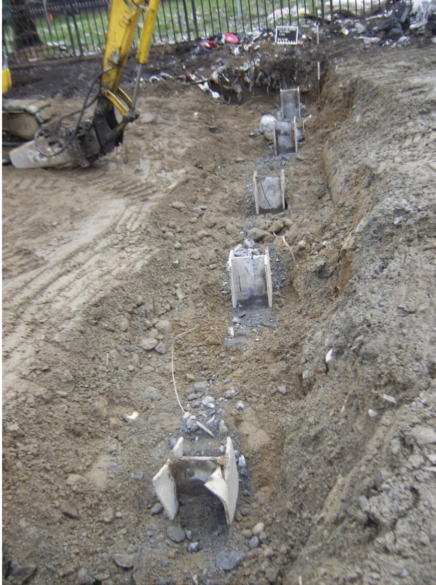
Photograph 34: (4/22/11 memo) East 127 th Street, Test Trench 8, looking north showing truncated pilings.
