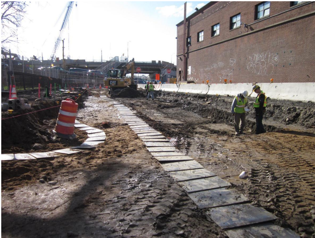
Photograph 40: (5/24/11 memo) East 127 th Street, utility pipes covered by steel plates, looking east.
