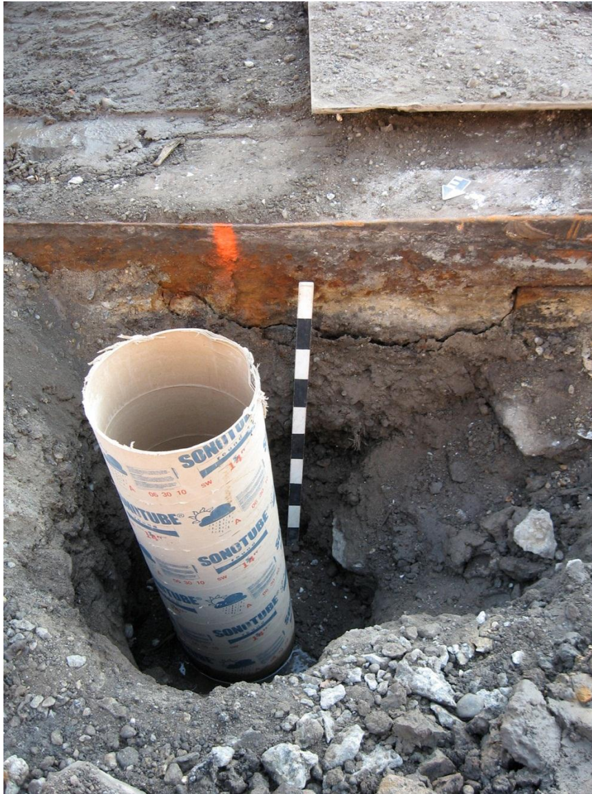
Photograph 9: (12/1/10 memo) First Avenue, Sono tube in place.
