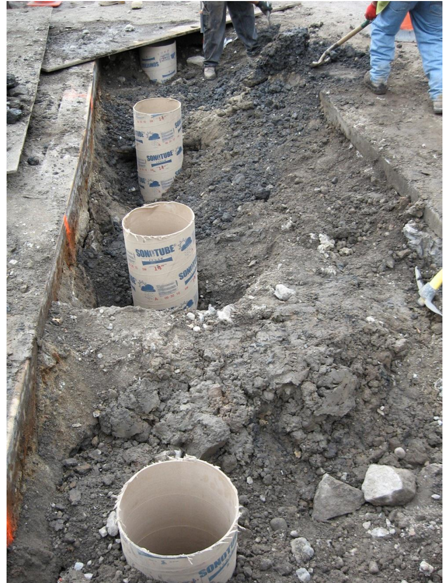
Photograph 10: (12/1/10 memo) First Avenue, Sono tube series in place.
