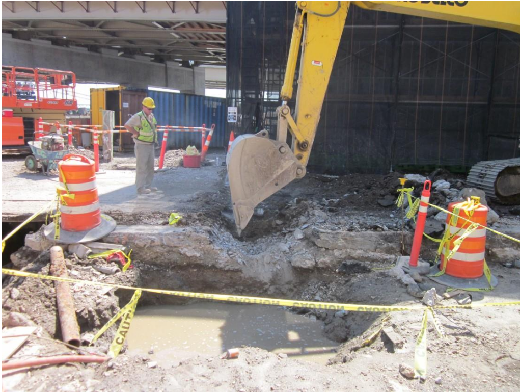
Photograph 24: (9/30/11 memo) First Avenue, north end by bridgetender's house, looking east. Trench for water connection to bridgetender's house.
