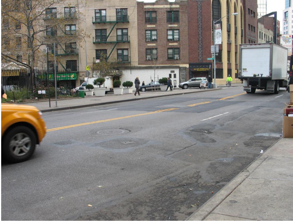
Photograph 3: Example of embedded utility covers in pavement and patched asphalt. View looking northeast with Mulberry Street in background.
