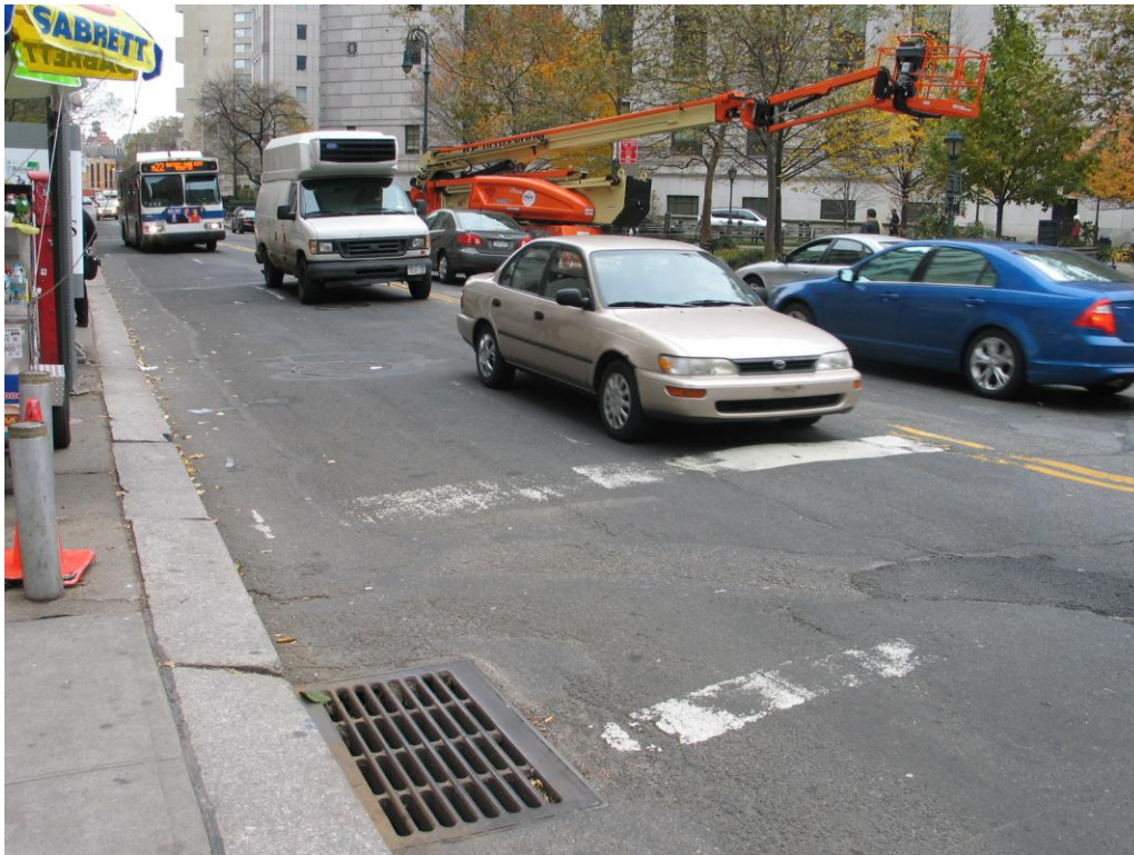
Photograph 4: Example of catch basin embedded in pavement. View looking southeast from near Centre Street intersection.
