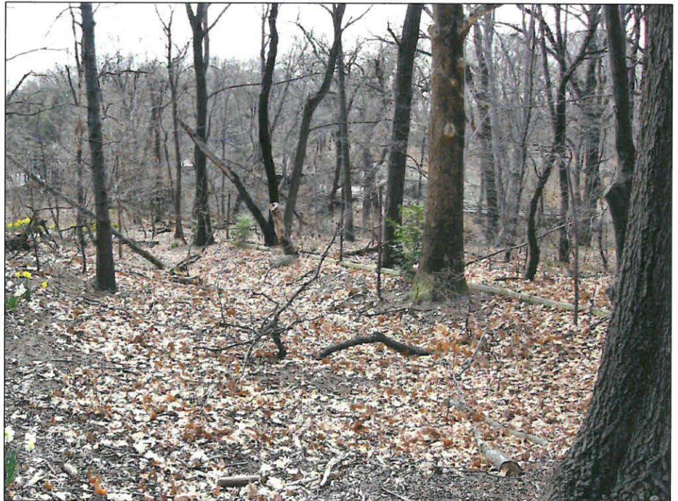
Low concrete wall running through woods between the eco-restroom and the river; looking southwest 16
