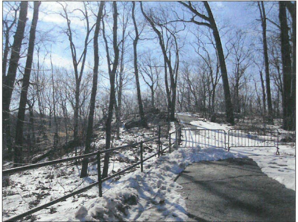
An asphalt path leading up a steep slope south of Jungle World Road 17 immediately west of the existing bridge
