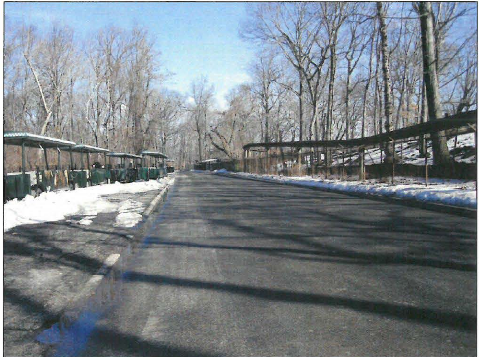
Looking north along Jungle World Road; the concrete footings and tracks of the Bengali Express Monorail are at the right of the photograph 21
