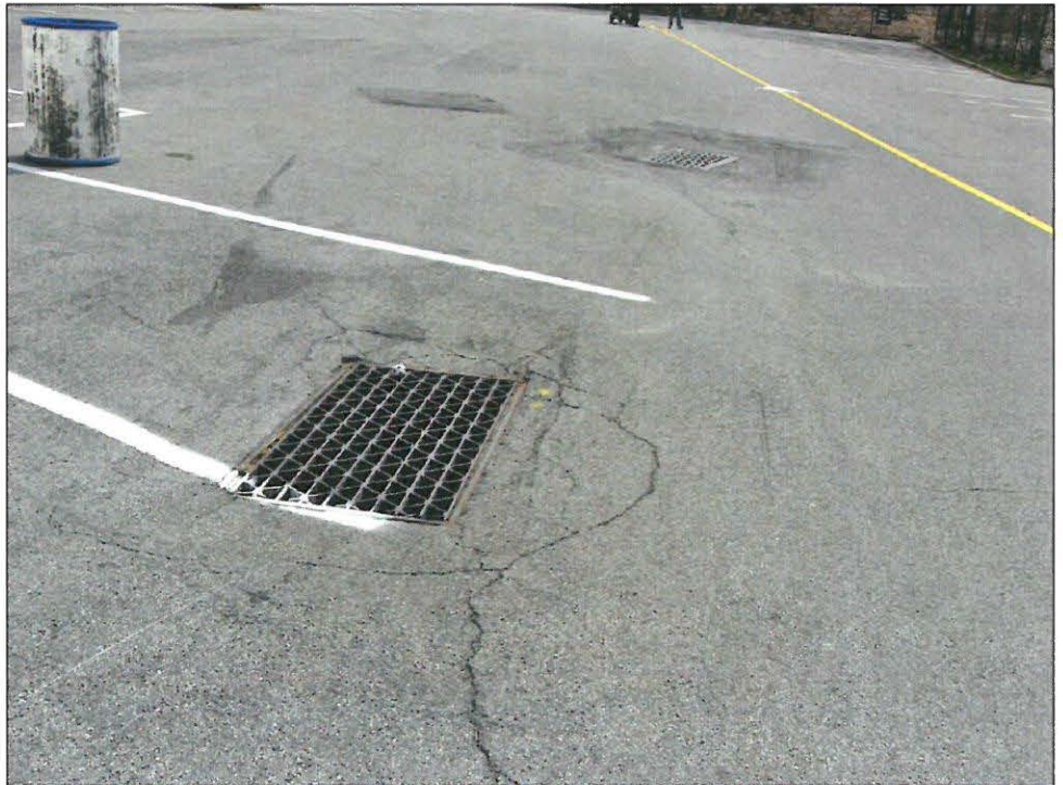
Catch basins in Bronxdale Parking Lot 2
