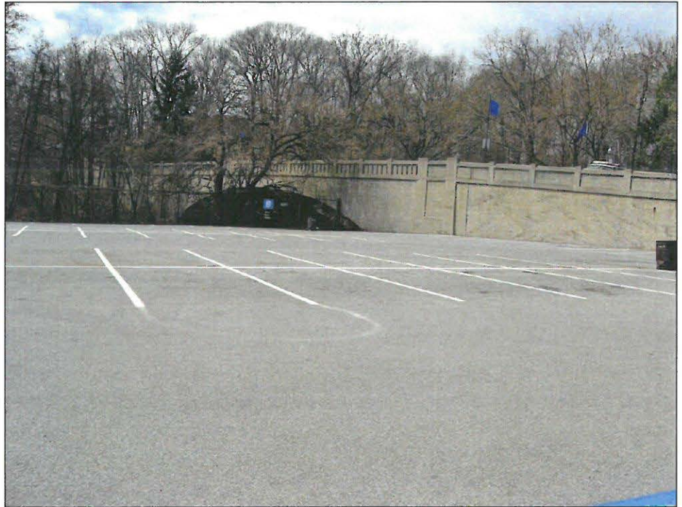
Bridge over Bronx River at Boston Road, looking northwest 3
