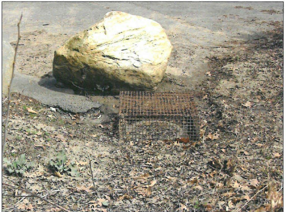
Catch basin in southern portion of overflow parking area and large boulder characteristic of those in the area 10
