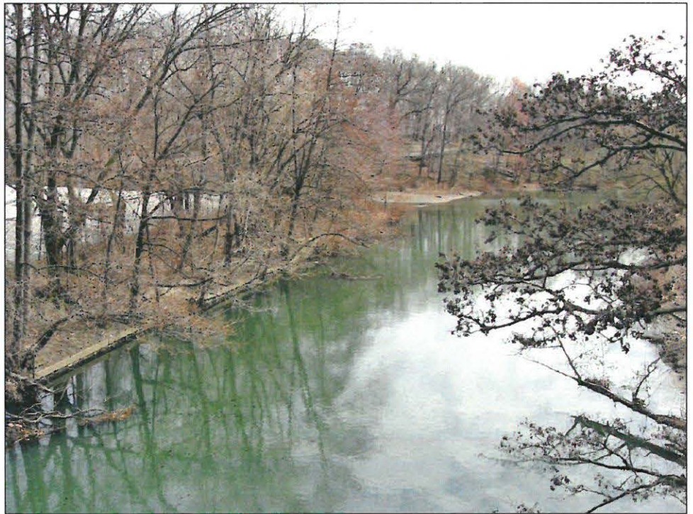
Bronx River and retaining wall along western side of parking lot, looking southeast 4
