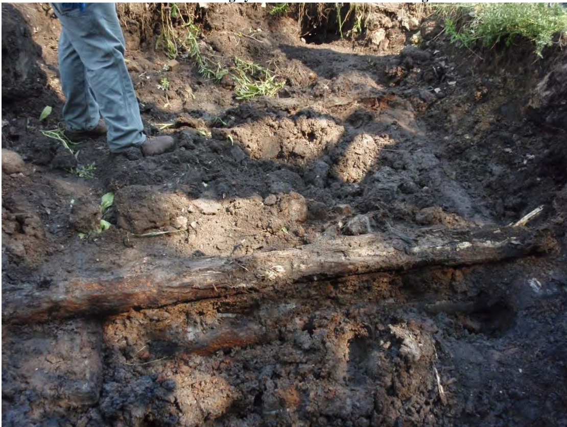
Photo 8 – View of additional layers of cribbing at 400 Carroll Street.
