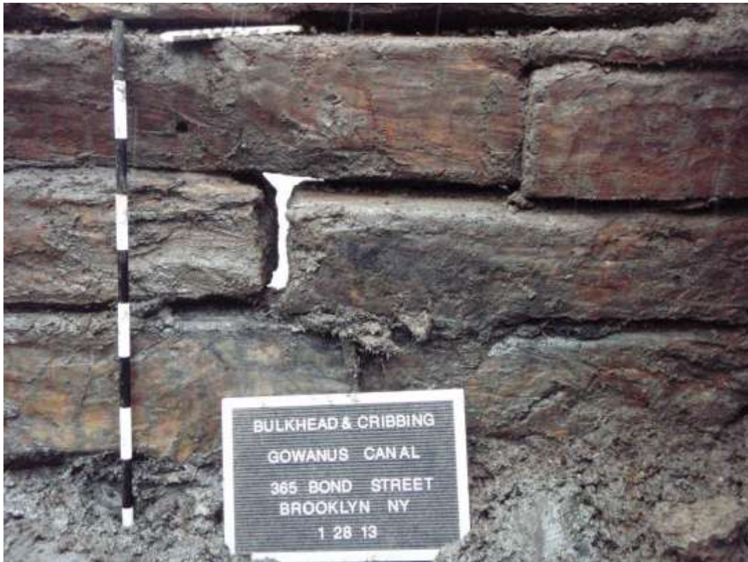
Photo 12 – Close up of landward side of bulkhead wall, facing southeast. Notice gaps from deterioration. Photograph taken by Michael Audin 1/29/2013.
