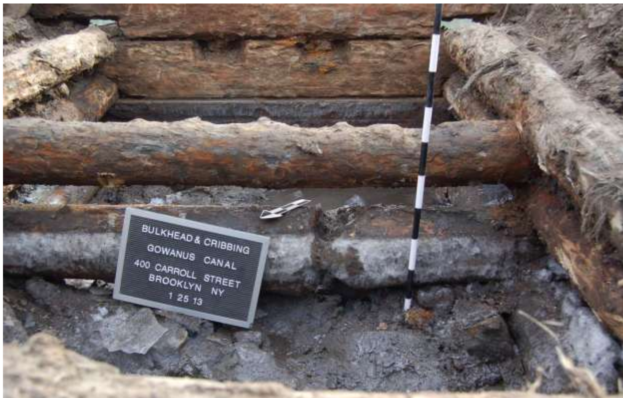
Photo 6 – View of central timbers of cribbing, facing east, notice joint in second row of one timber ending and another beginning. Photograph taken by Michael Audin, 1/25/2013.
