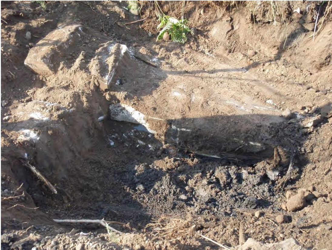
Photo 4 – View of concrete slab found approximately 2 feet below surface at 365 Bond Street.
