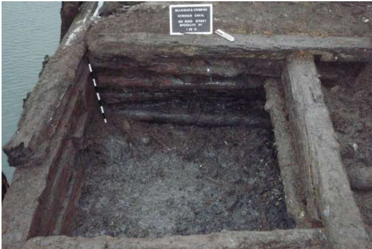
Photo 14 – View of the south wall of cribbing, facing southwest. Notice the top timbers are square and lower timbers are round with 3rd row of round timbers pushed out. Photograph taken by Michael Audin 1/29/2013.
