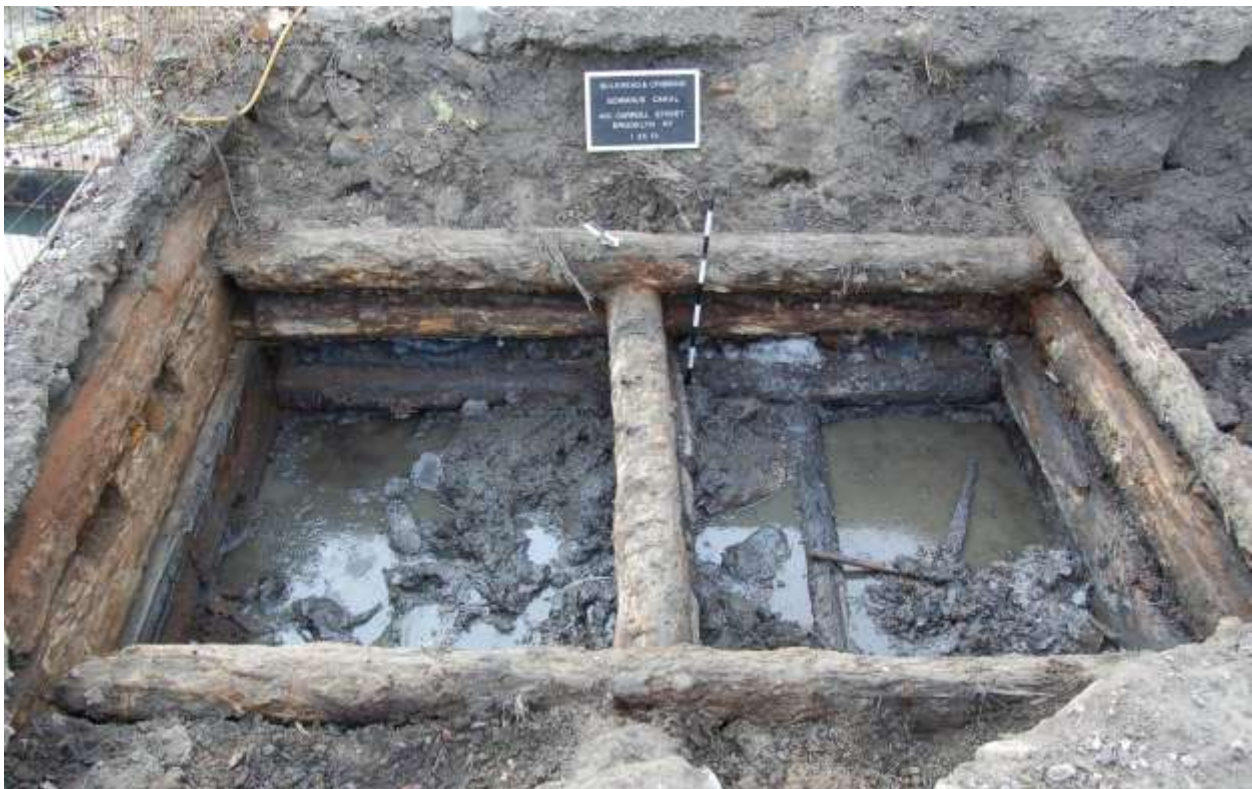
Photo 5 – Plan view of the 400 Carroll Street cribbing and interior of bulkhead wall, facing south. Photograph taken by Michael Audin, 1/25/2013.
