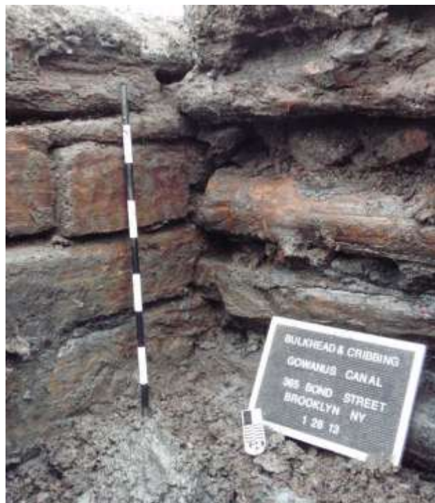
Photo 13 – Close up of tie back timbers taper cut to fit into bulkhead wall slots, facing south. Photograph taken by Michael Audin 1/29/2013.
