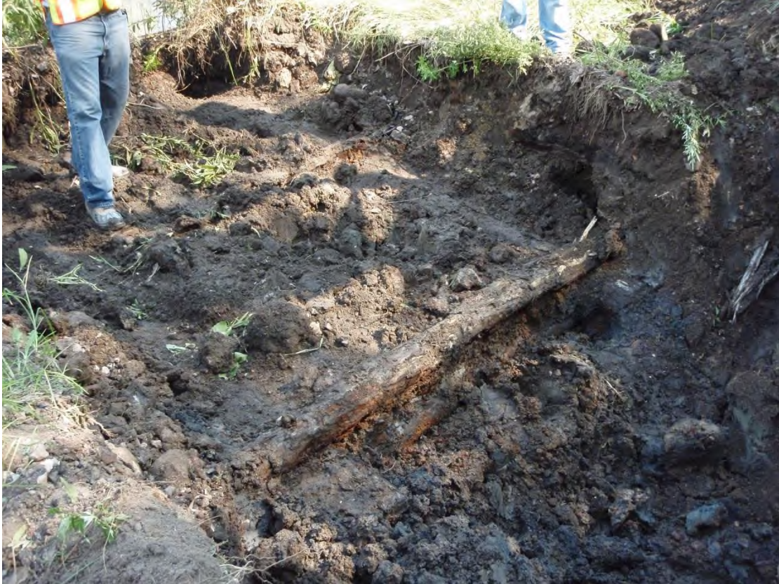
Photo 7 – View of cribbing system at 400 Carroll St. looking southeast.
