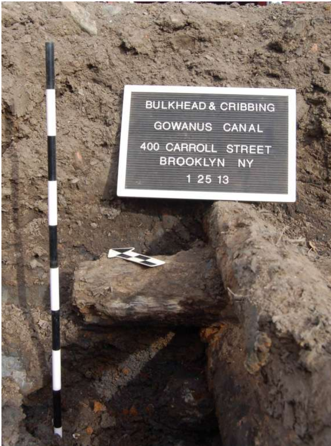
Photo 8 – Close up of end of tie back timbers at west end of cribbing, facing north. Photograph taken Michael Audin 1/25/2013.
