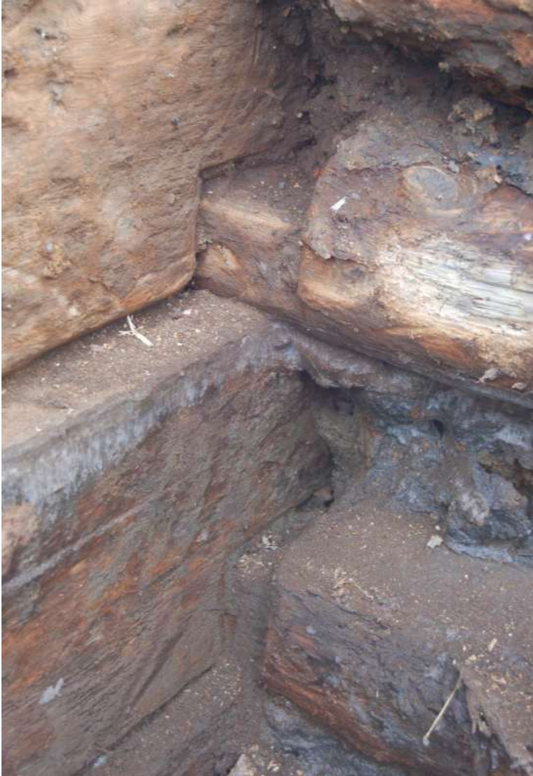
Photo 9 – Close up of tie back timbers tapered to fit into the bulkhead wall, facing southeast. Photograph taken Michael Audin 1/25/2013.
