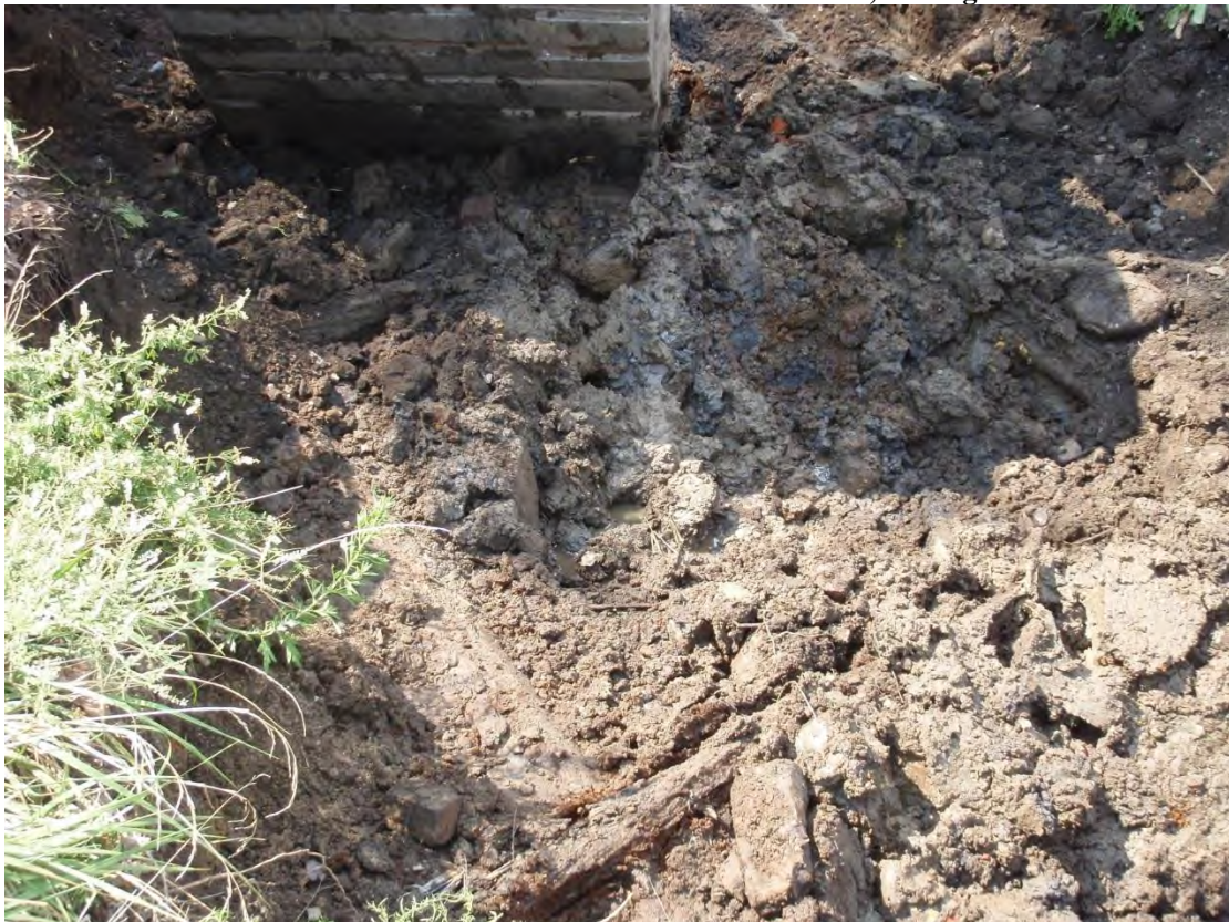
Photo 6 – View of excavation at 400 Carroll St with first portion of cribbing exposed.
