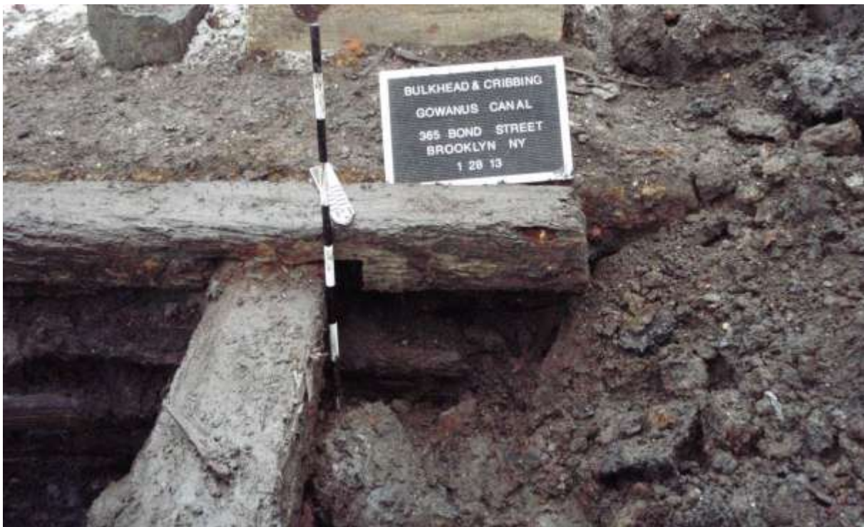
Photo 17 – View of notch cut for top square timbers of cribbing most likely more recent than the round timbers below, facing south. Photograph taken by Michael Audin 1/29/2013.
