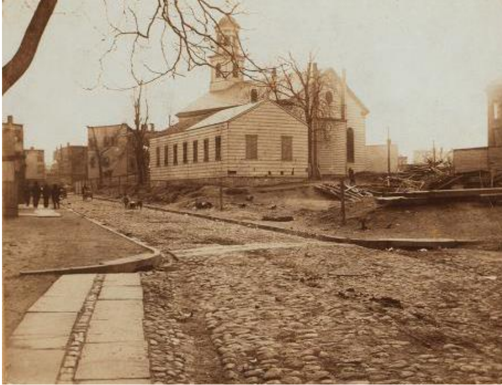
Photograph 17: Rear of second Bushwick Reformed Dutch Church as seen in 1907. Former cemetery located in area with ground disturbance shown, to rear of church, more than 100 feet north of the APE. View looking southwest from intersection of Woodpoint Road and Skillman Avenue. Courtesy New York Public Library.
