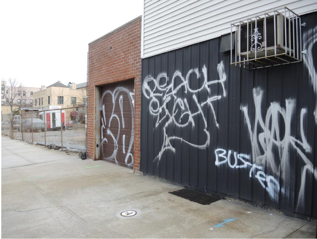
Photograph 1: Former Lot 2 with brick faced one-story garage abutting and connecting to the building on former Lot 1. View looking northeast from Humboldt Street.
