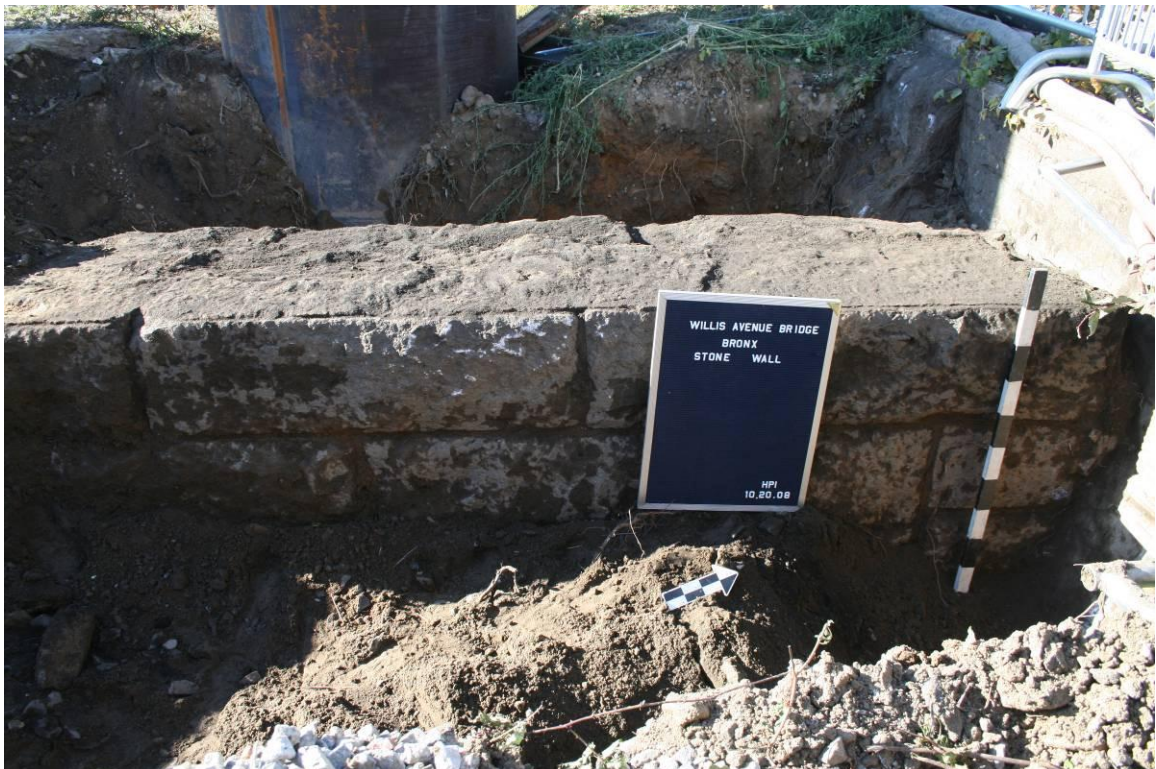
Photograph 8: Stone wall encountered in excavation pit for Pier BI, facing west. Note that the material and design match both the extant stairwell and the historical retaining wall, and that the northern end of the wall abuts the historical retaining wall, at the right.
