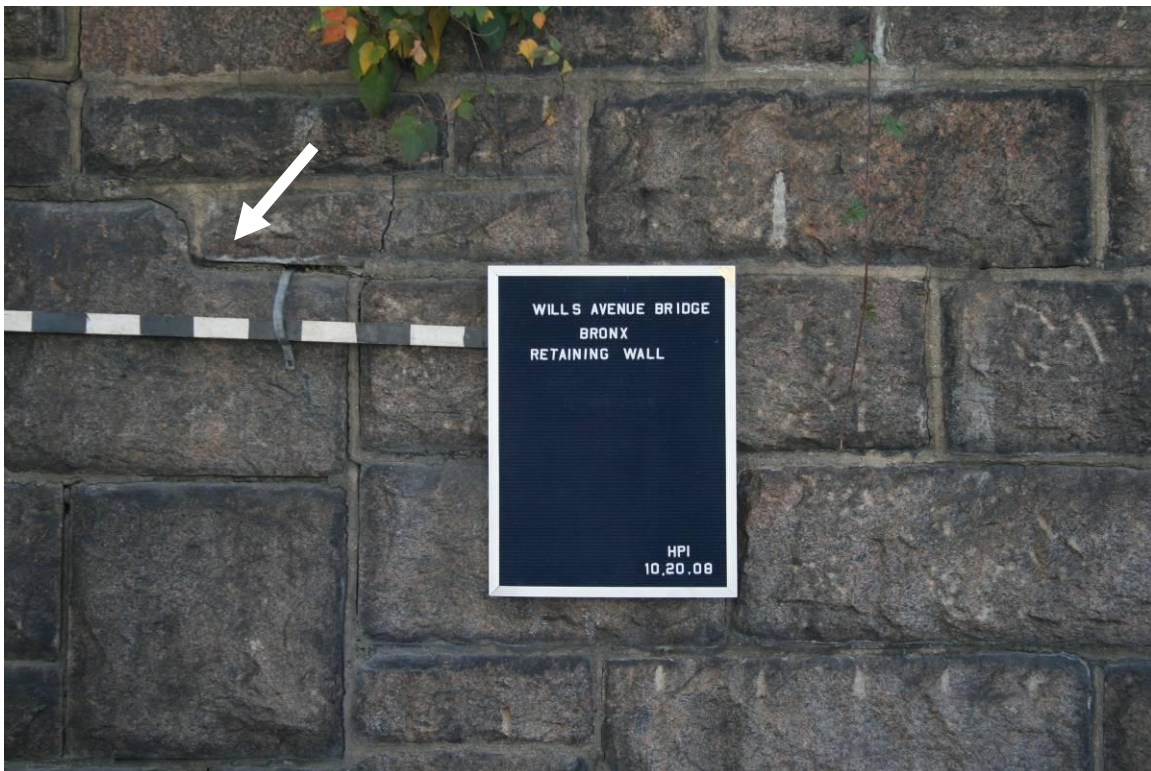
Photograph 6: Close up of historical stone retaining wall on Willis Avenue, facing southwest. Note the cracked joints that demarcate where the wall was patched after the stairwell was abandoned and sealed up.
