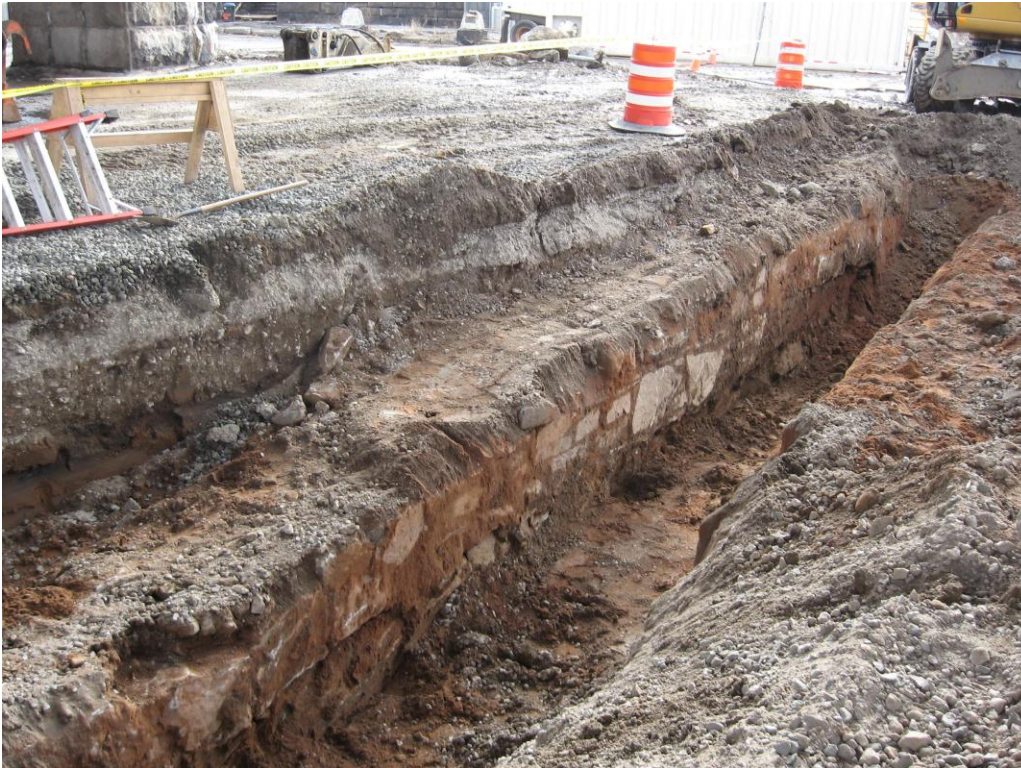
Photograph 1: Exterior edge of the 1870s railroad roundhouse wall, shown within Pier 11 trench. View looking southeast.
