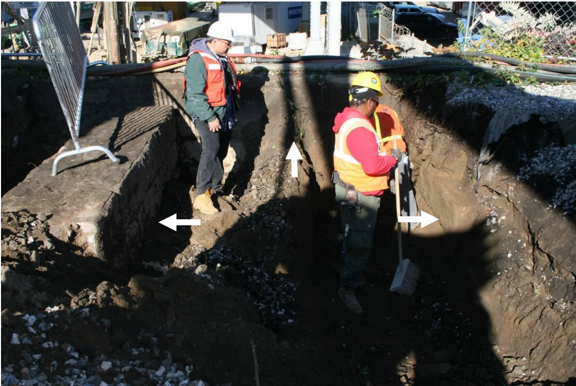
Photograph 9: First stone wall encountered in Pier BI on left, and second stone wall encountered at right. Note that the men are standing in what would have been the stairwell before it was filled. The patched historical stone retaining wall that fronts onto Willis Avenue is between the two stairwell walls in the rear of the photograph.
