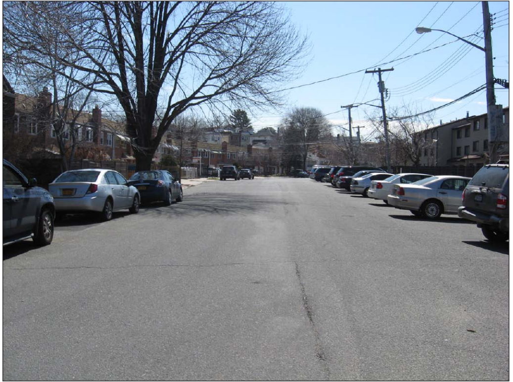
Looking south along 115th Street from Poppenhusen Avenue 9
