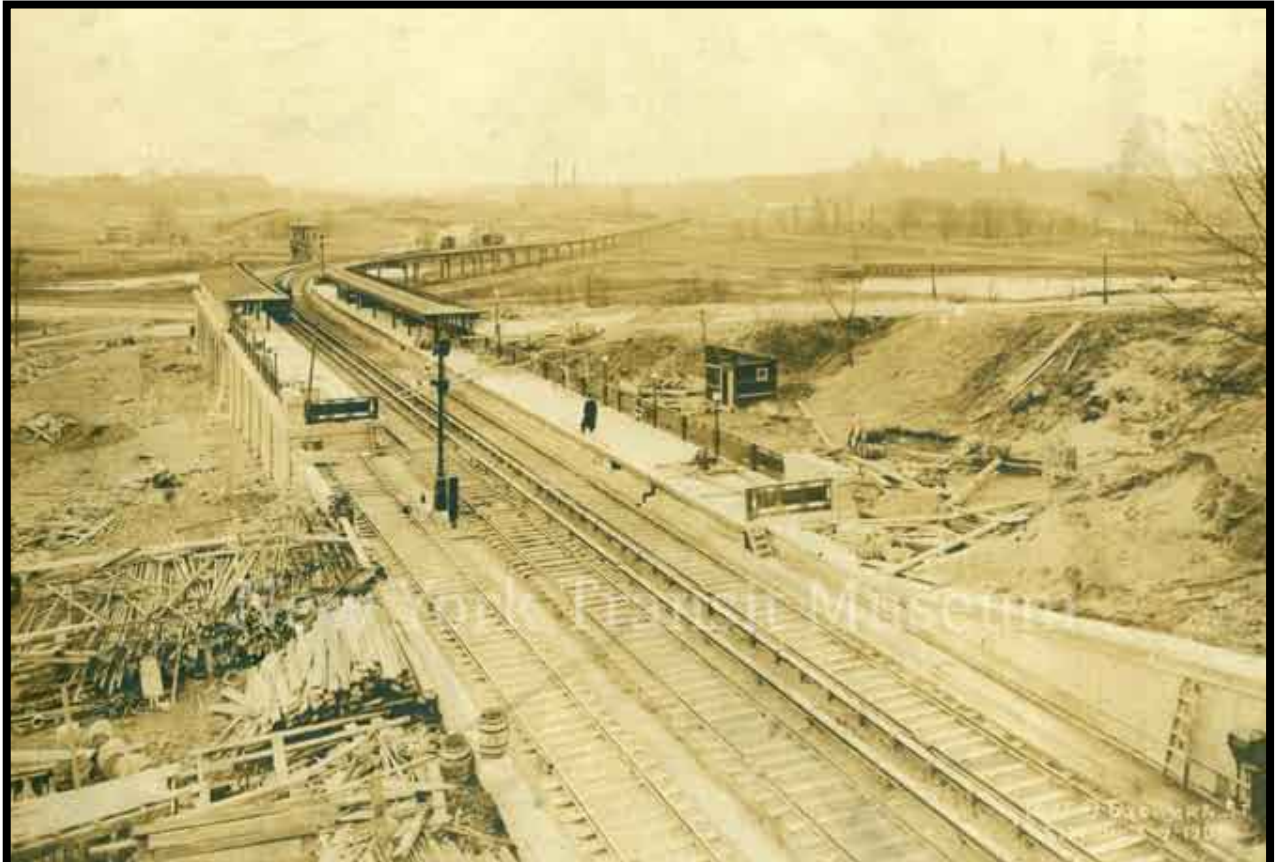
Construction of the Dyckman Street IRT station in 1906, looking northeast (NYTM).
