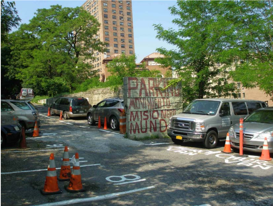
Photograph 5. Concrete Retaining Wall on West Side of Site.
