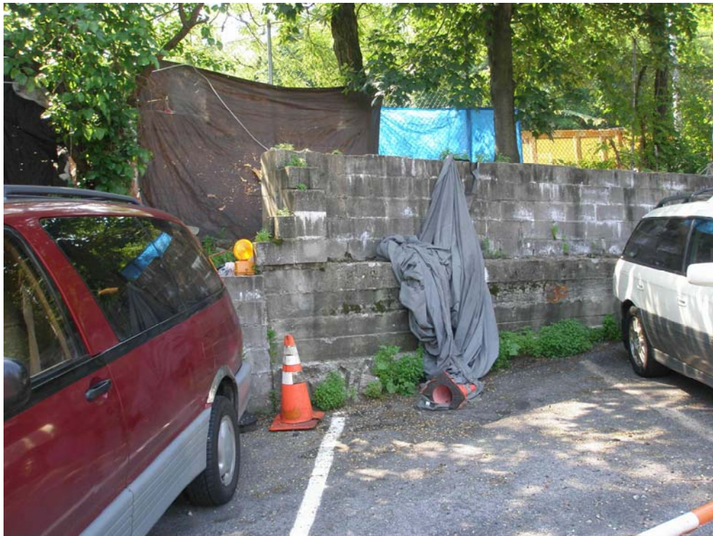
Photograph 6. Modern Concrete Block Retaining Wall on East Side of Parking Lot where Surface was Leveled for Parking.
