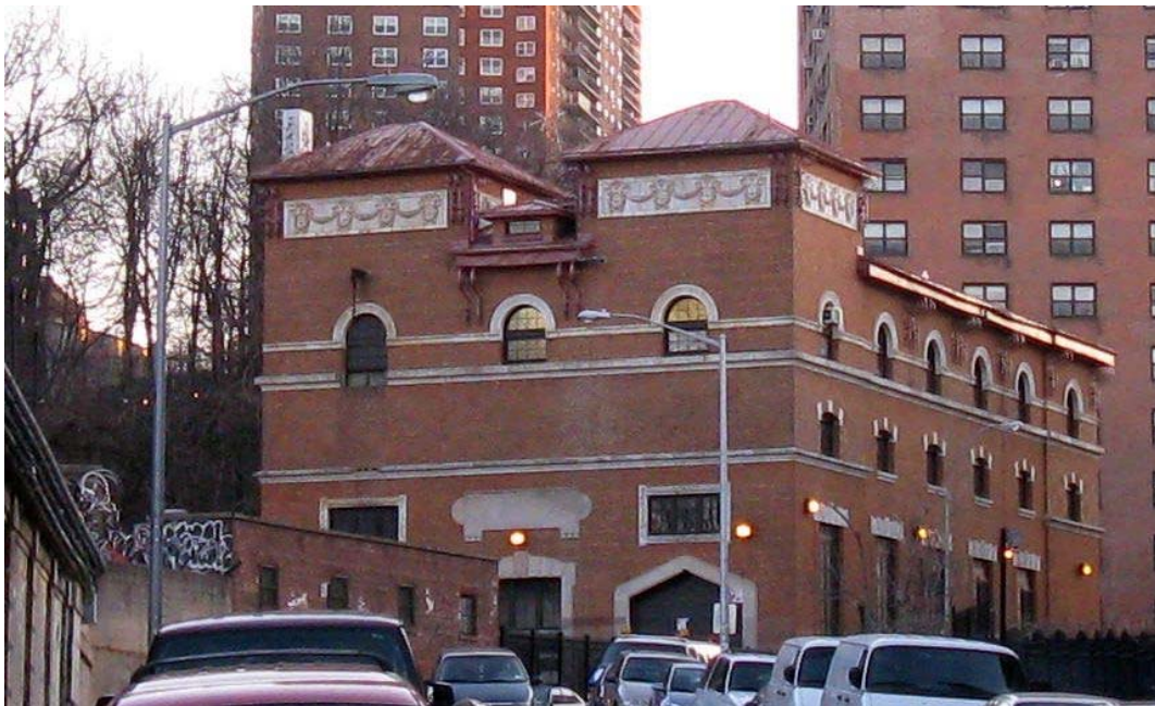
Photograph 10. Sub Station #17, Facing South. Project Site is at Left.
