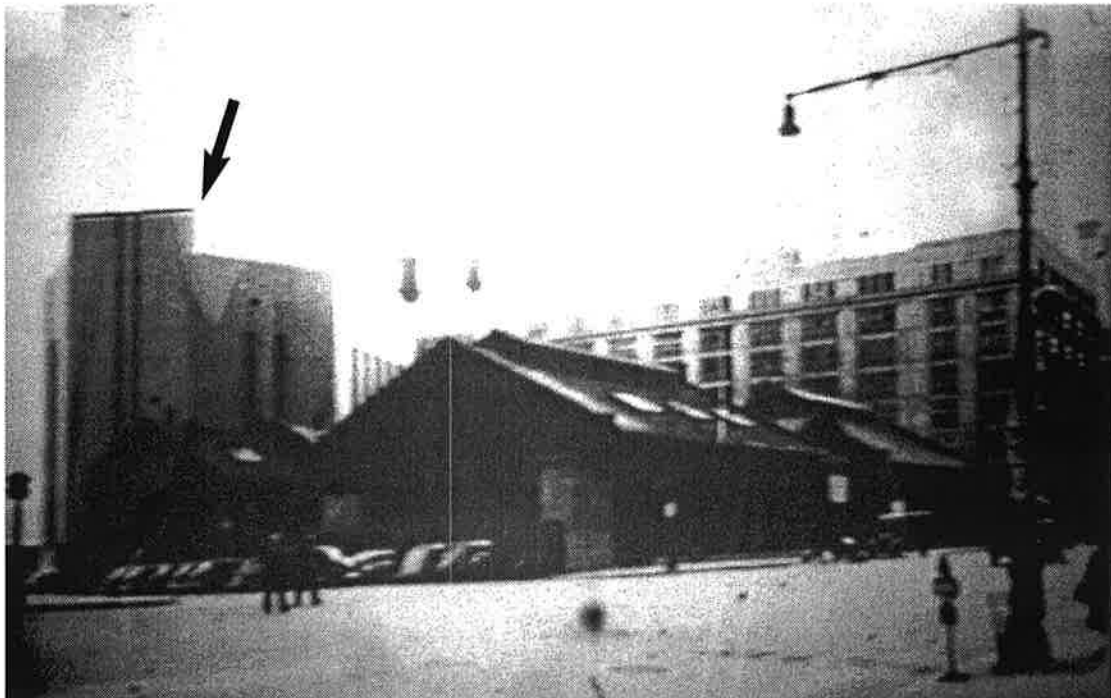
7 View from the southeast corner of East 42nd Street and First Avenue on October 3, 1940, as construction of the Queens Midtown Tunnel was drawing to a close. Gas company buildings are still standing on the project site, and the 6-story tunnel ventilator building (arrow) is located on the east side of the block, beyond the project APE. (Sperr 1940: 524-B8)
