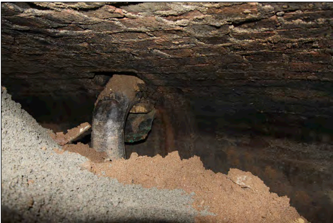
Image 7.17: Cistern interior showing inlet connection from the roof gutters.
