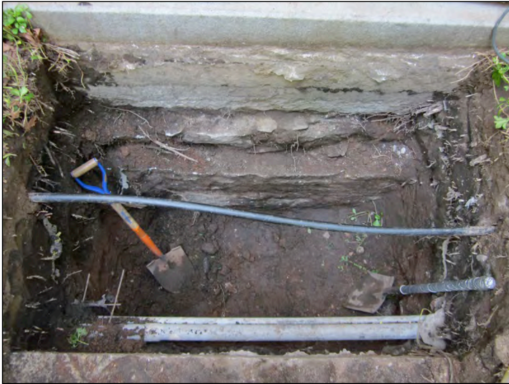
Image 7.02: Excavation of the area connecting Manhole 3 with Tweed Courthouse. The window well foundation for Tweed Courthouse is visible in the top portion of the excavation area.
