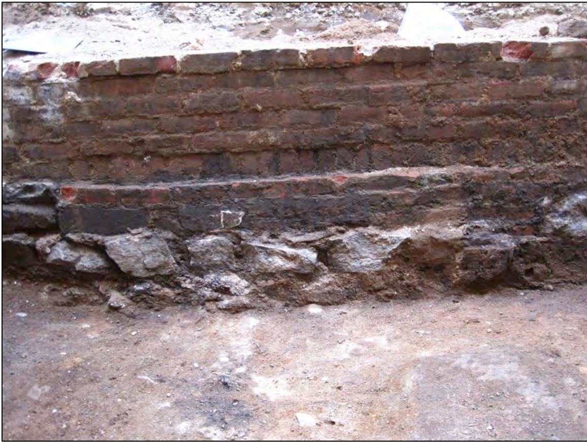
Image 7.79: Feature 4, view of interior brickwork and schist footers of northern wall.
