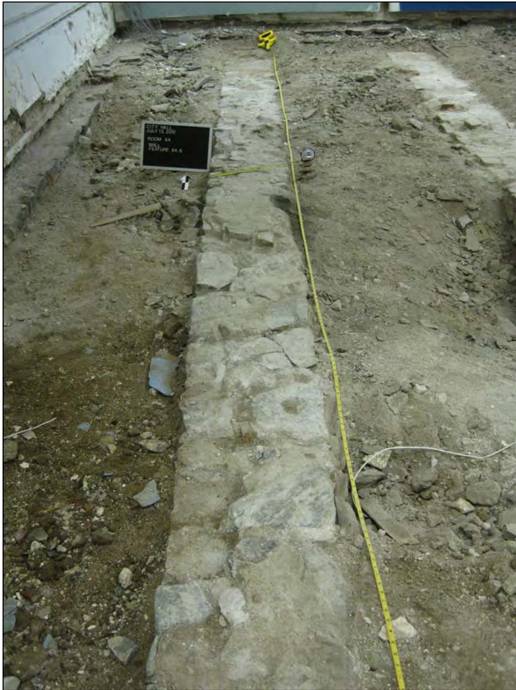
Image 7.30: Fully exposed stone footer within Room 6A.
