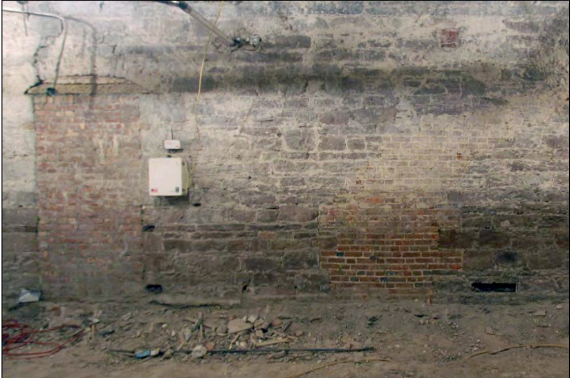
Image 7.49: Closed brick fireplace with stepped chimney flue visible within the stone wall.
