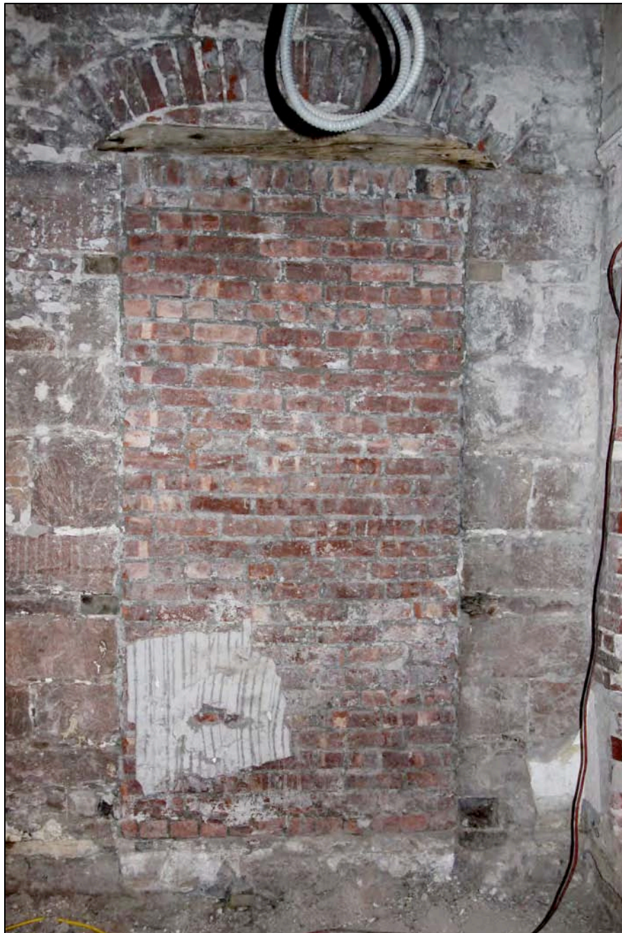
Image 7.48: Bricked-up doorway exhibiting original arched brick frame in Room 6B.
