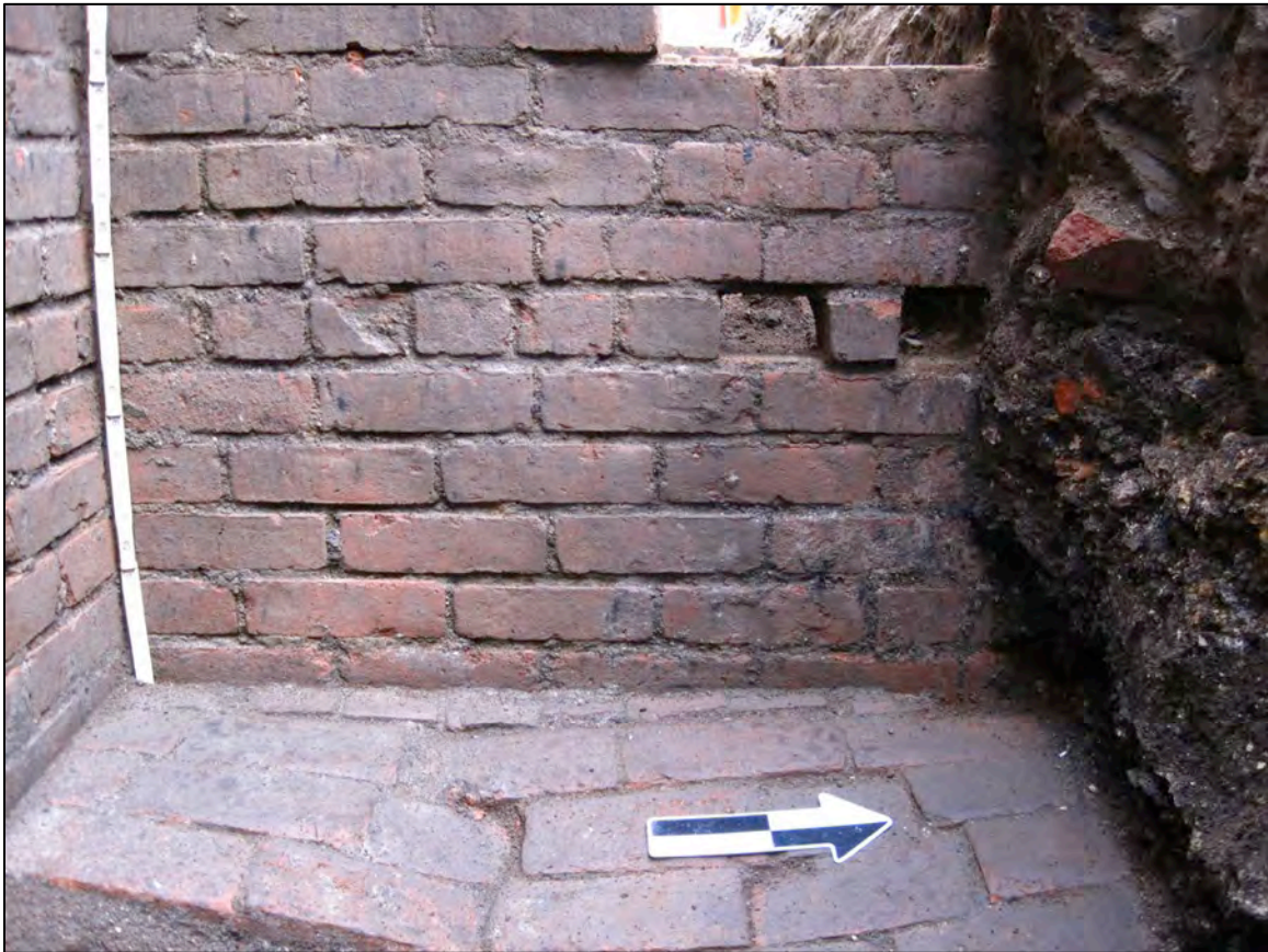
Image 7.71: Wall openings to facilitate drainage were present in the east and west walls of Feature 3.
