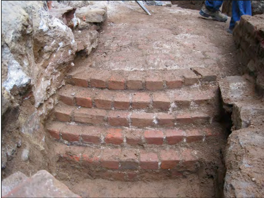
Images 7.58: Feature 2, a brick domed cistern with stepped sides.
