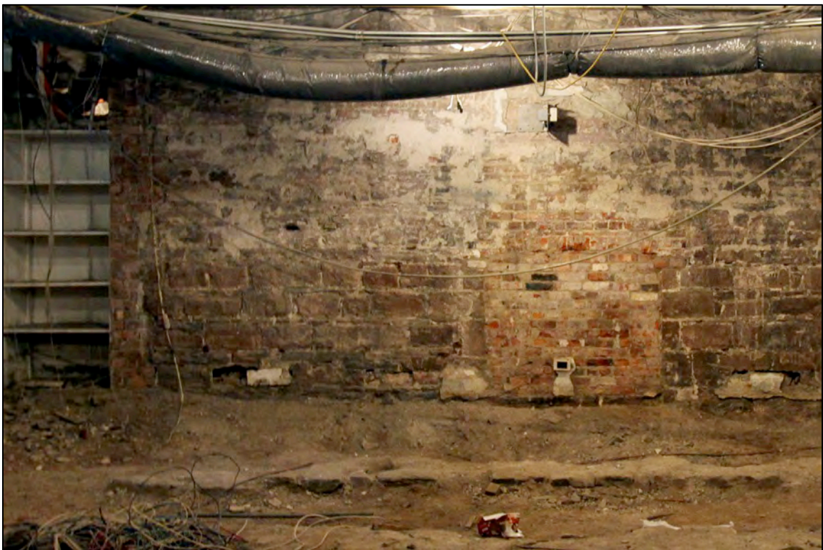
Image 7.50: Former fireplace in Room 8C, exposed after excavation of the fireplace foundation had been uncovered in Test Unit 8C.4.
