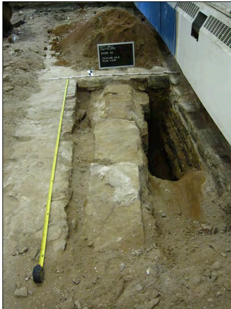
Image 7.31: Stone capped nineteenth-century drain line.
