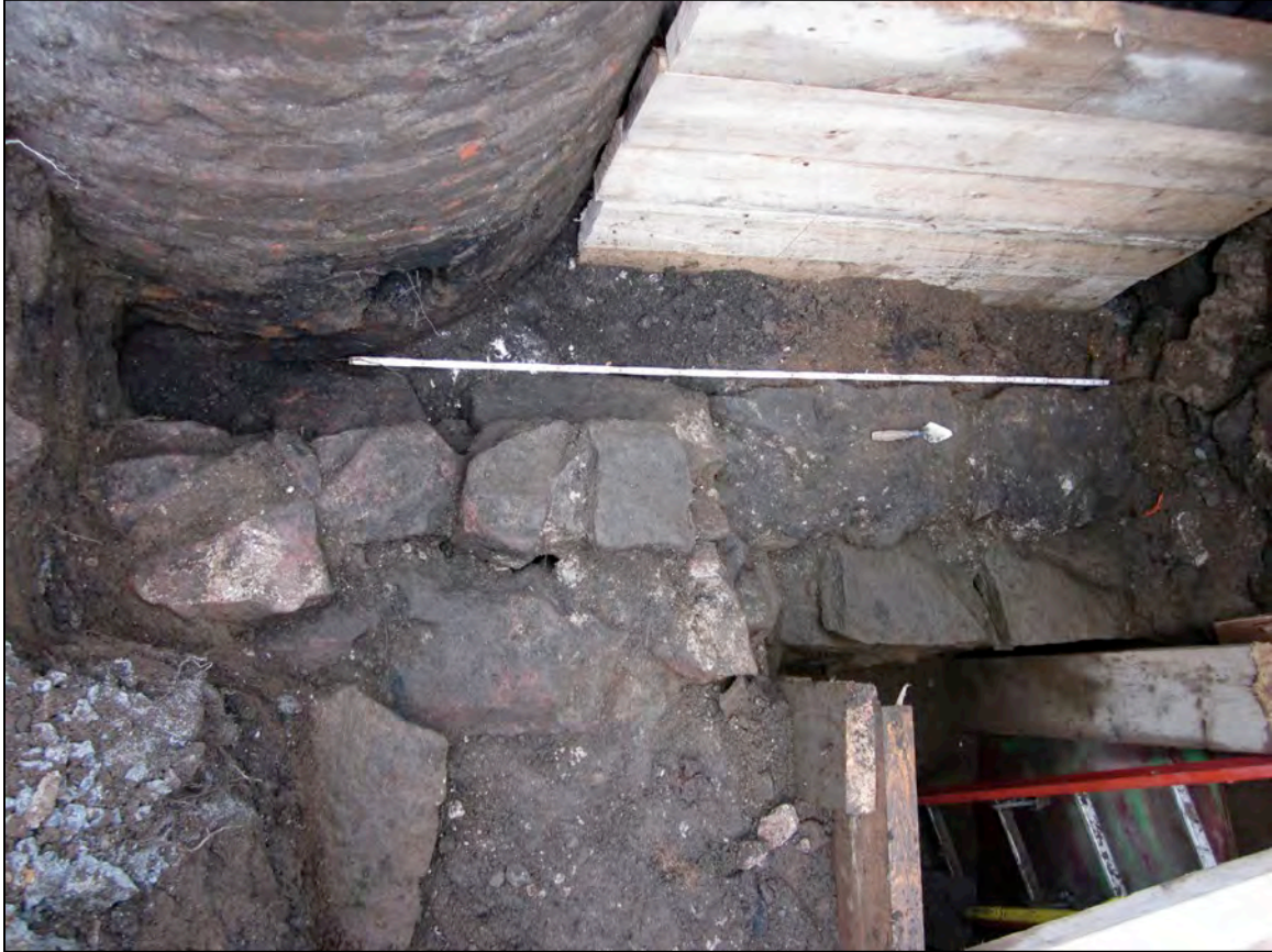
Image 7.129: Schist foundation wall exposed beneath Features 37 and 39.
