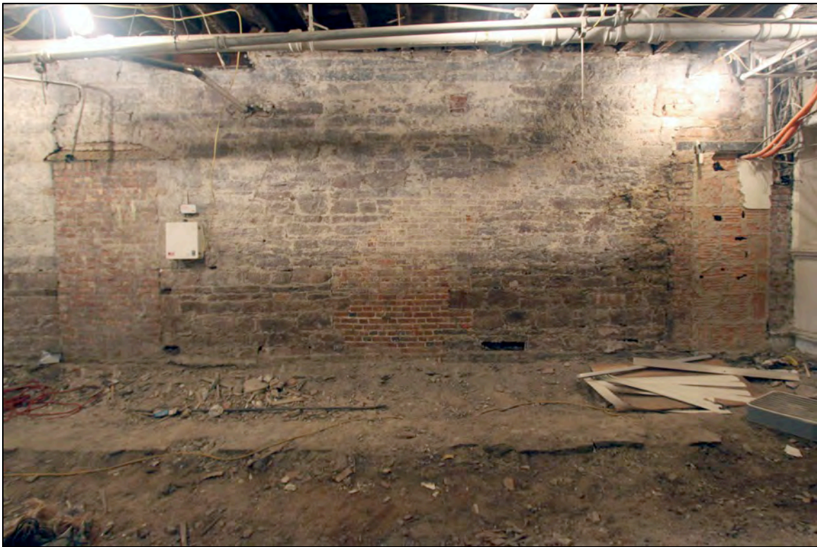
Image 7.45: West wall of Room 6B. Note the reverse side of the former chimney flue and fireplace first observed in Room 8C at the center.
