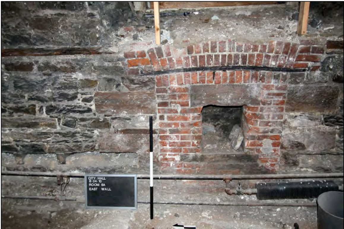
Image 7.47: Brick fireplace along the exposed east wall of Room 6A.
