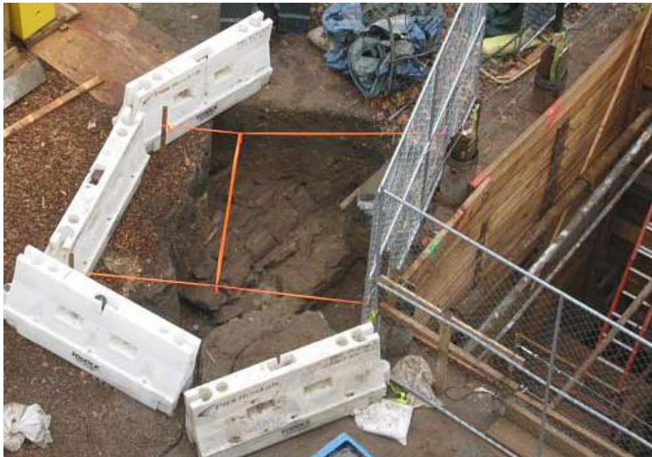
EXTENSION OF MANHOLE #3
