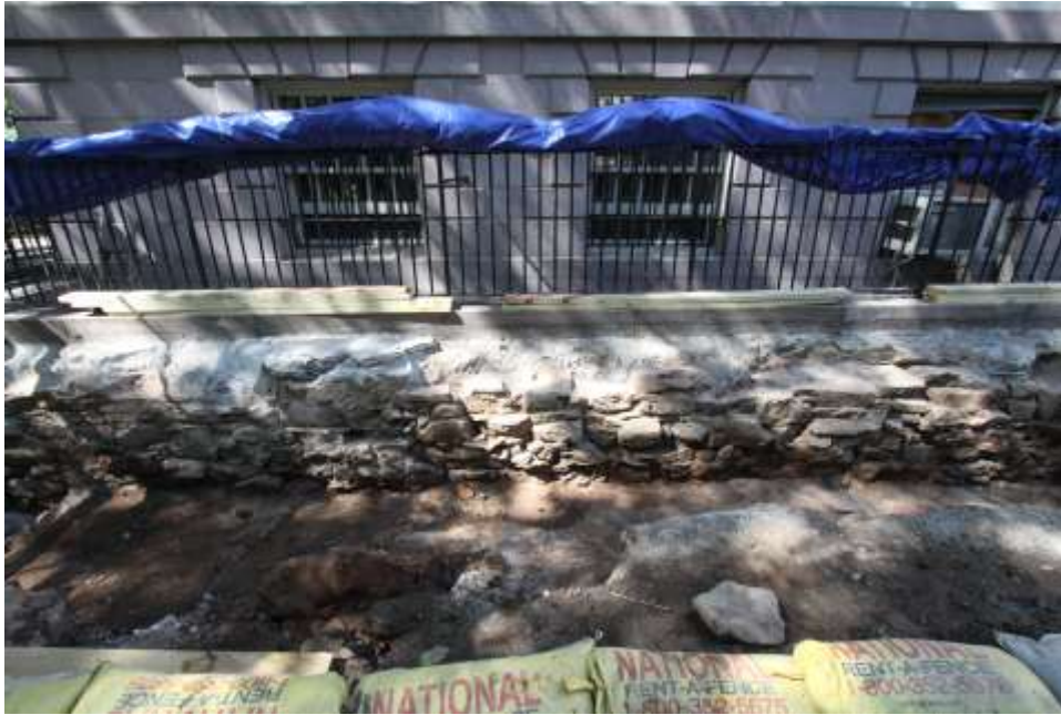
Image 01 - Northeast Area Original City Hall retaining wall
