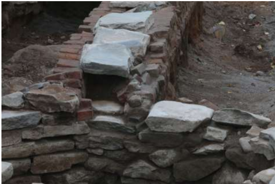
Image 62 – Northeast Area Flagstone and brick drainage
