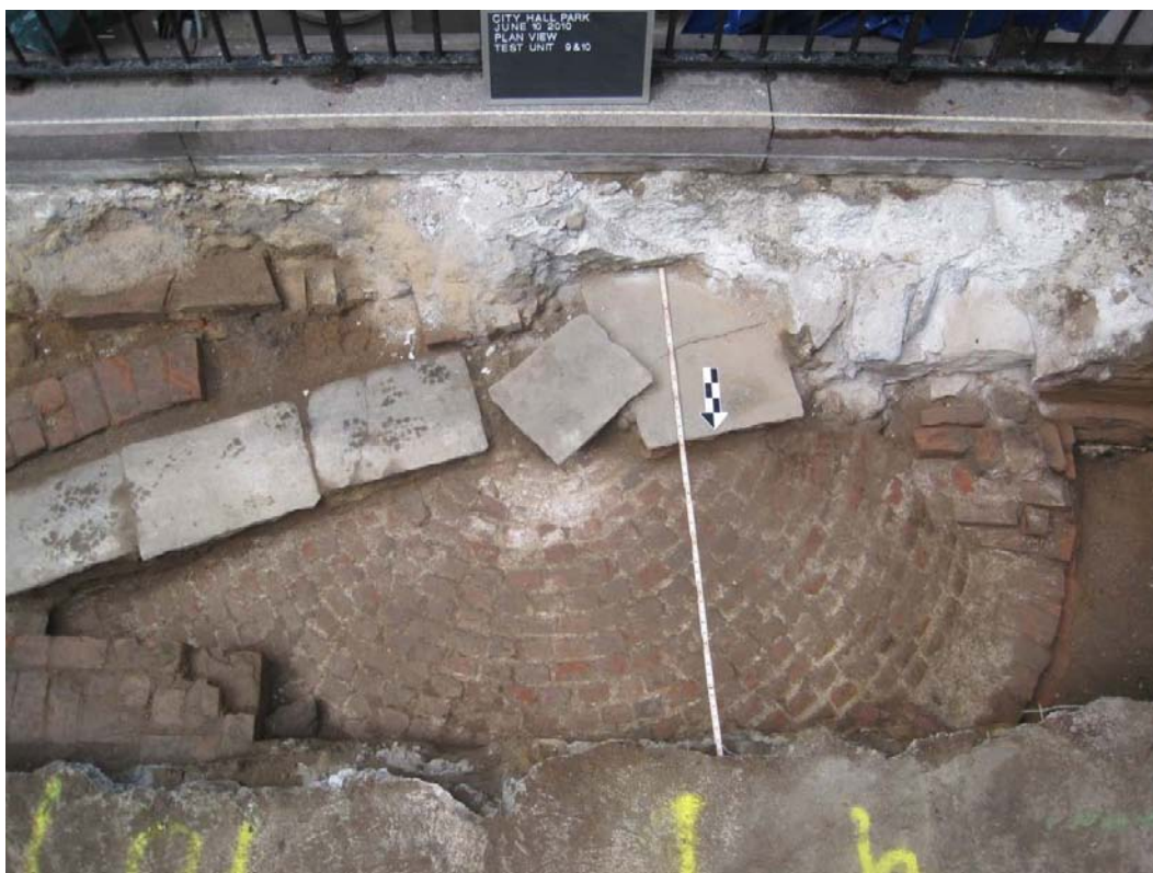
Image 06: Brick domed cistern and flagstone path (Test Units 9 & 10)
