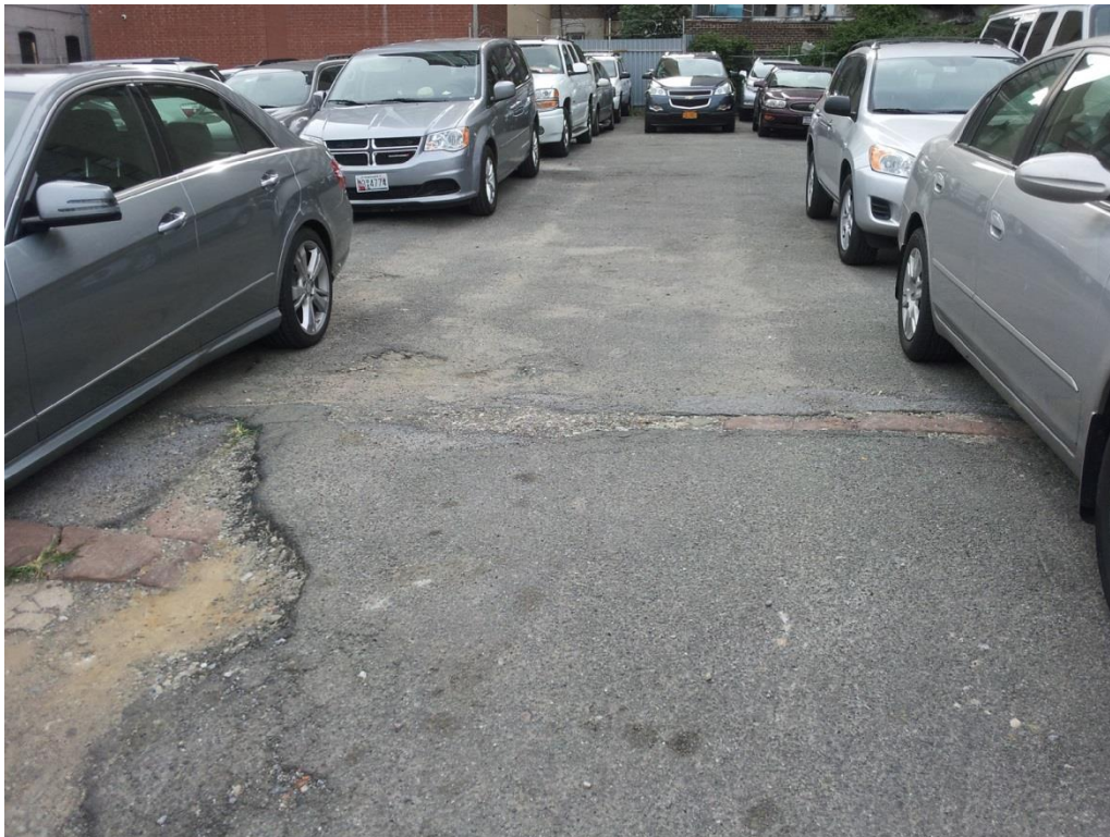
Photograph 14: Lot 41 showing detail of exposed foundation remains in foreground. View looking west from Gold Street.
