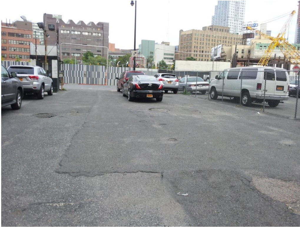
Photograph 9: Interior of Lot 37 parking lot showing patched pavement. View looking east toward Gold Street.
