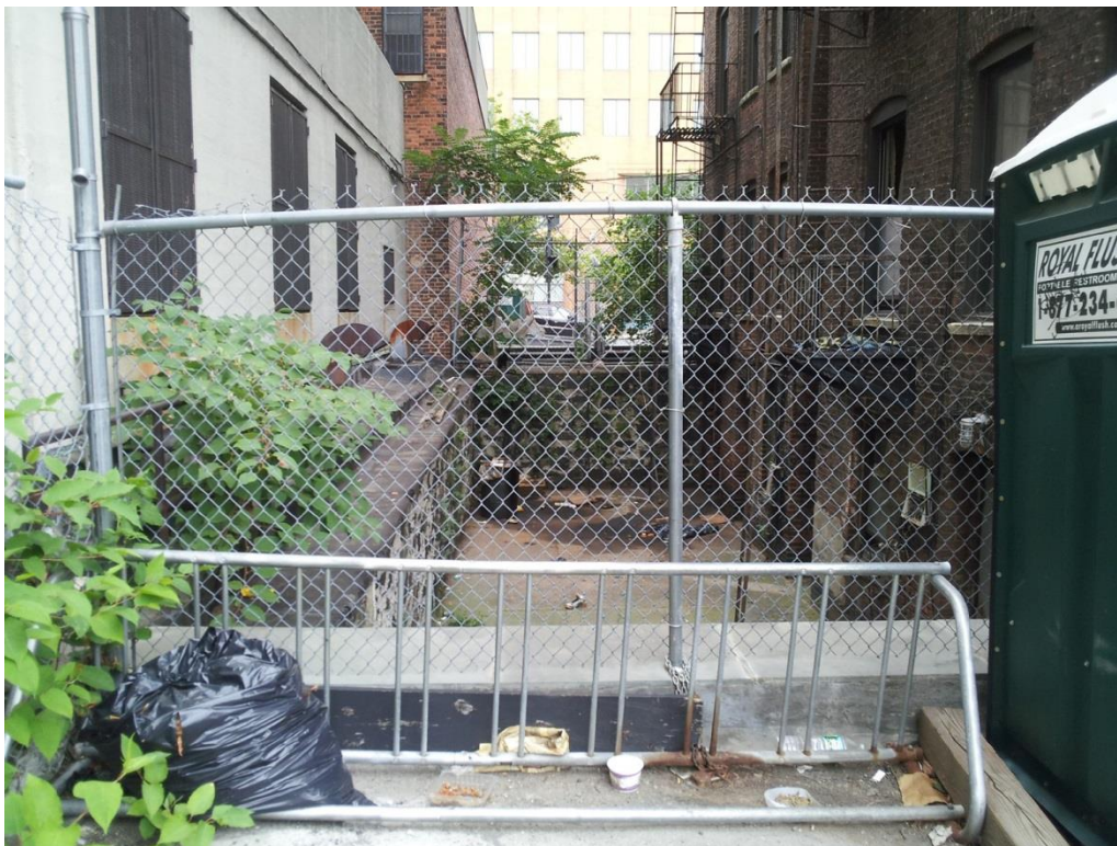
Photograph 10: Sunken yard of adjacent Lot 36 with retaining wall. Lot 29 of APE is visible in far background. View looking north from northwest corner of Lot 37.
