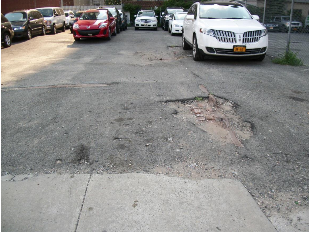
Photograph 13: Lot 41 showing detail of exposed foundation remains in foreground. View looking west from Gold Street.
