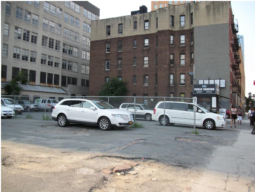
Photograph 12: Lot 41 parking lot with Lot 37 parking lot in rear. Note exposed foundation remains in foreground. View looking northwest from Gold Street.
