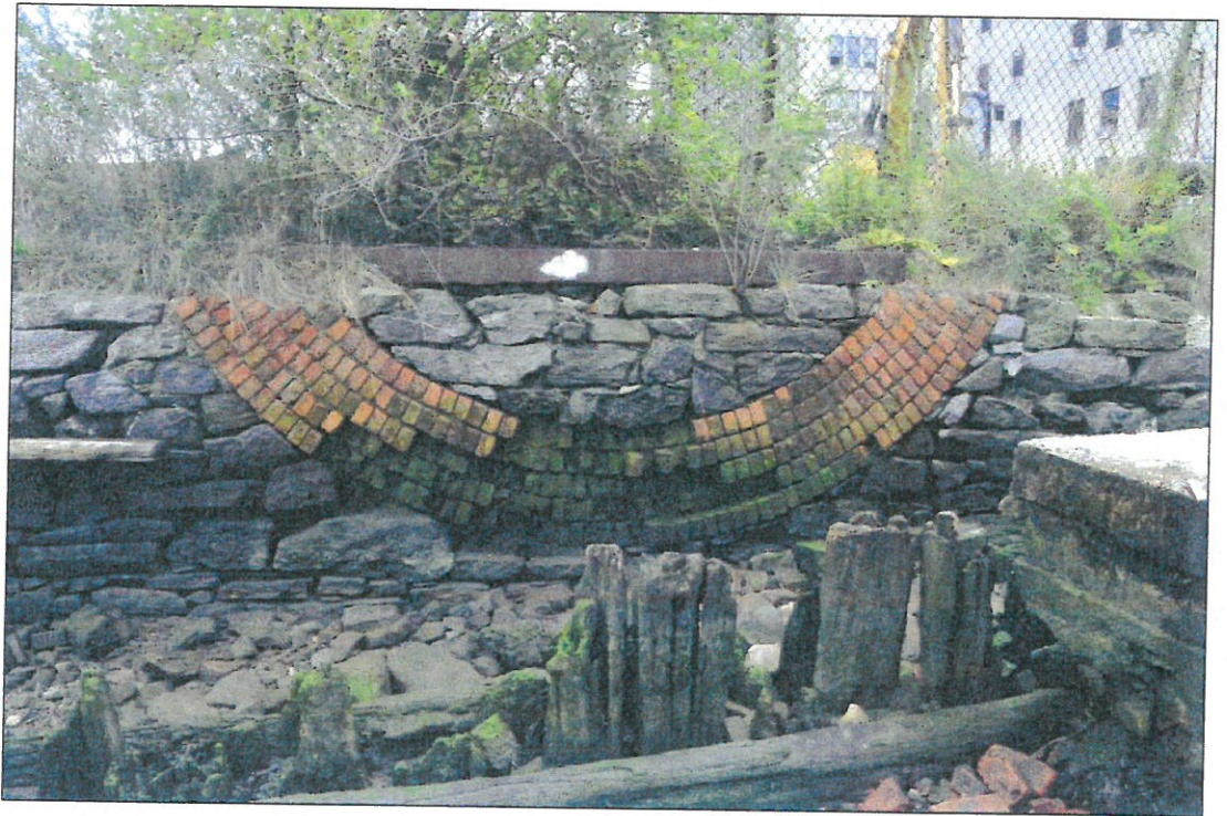
Facing east from the East River outside of the southwest corner of the project area showing brickwork incorporated into a stone retaining wall. Trench 1 is located several feet beyond this wall to the right 16
