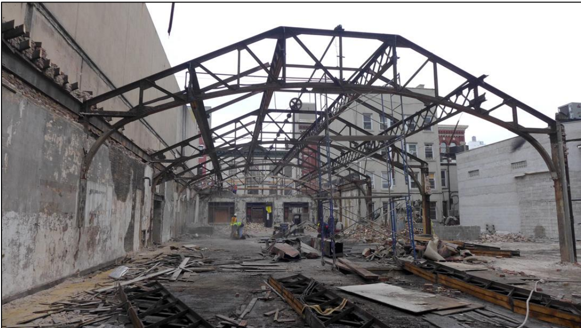
Image 19: The frame structure of the roof of 50 Bowery in the process of deconstruction.
