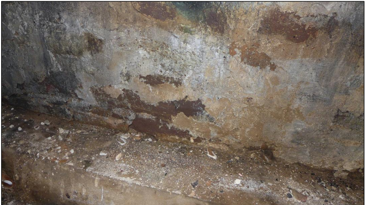
Image 12: Party wall between the basements of 50 Bowery and 52 Bowery with a poured cement curb at the floor. What appears to be brownstone is visible at the base of the wall and the curb.
