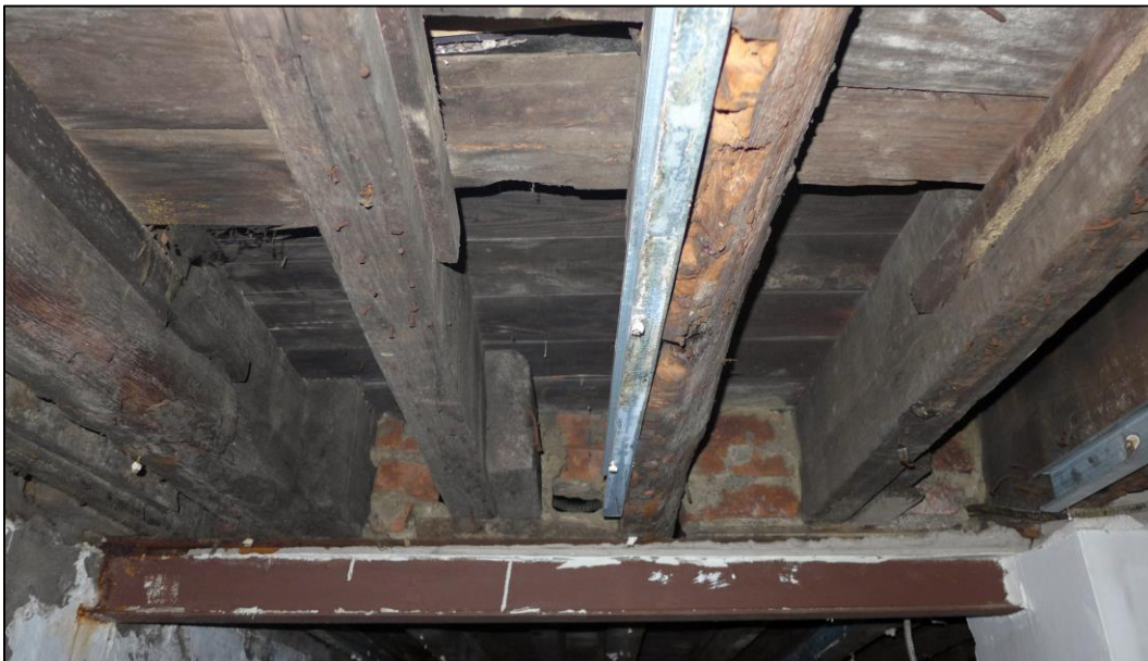
Image 10: Machine and axe cut beams visible in the basement level ceiling of 52-52½ Bowery.
