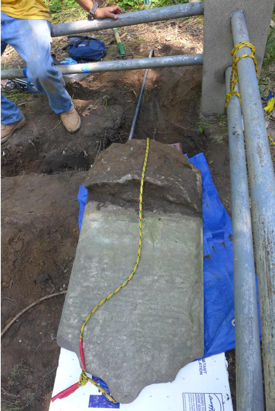
Image 13: Re-installation of tombstone.
