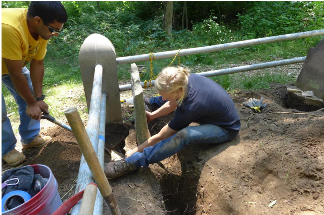
Image 12: Re-installation of tombstone.
