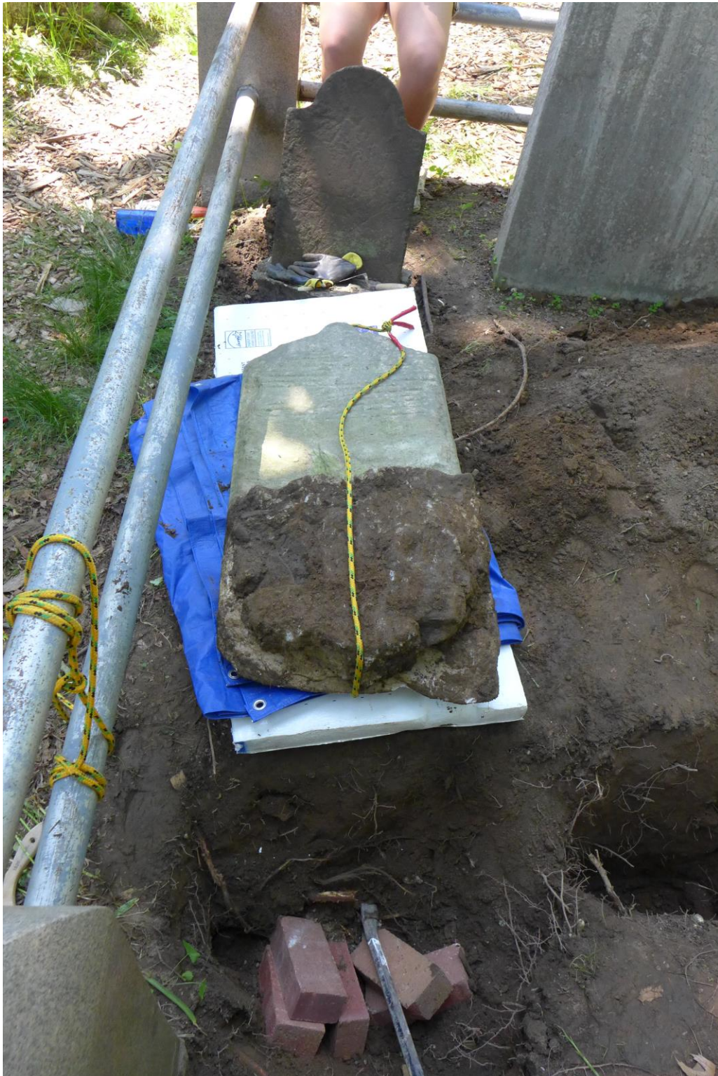
Image 04: Bricks to be installed in the “base” of the excavated area to act as supports for re-installed tombstones.
