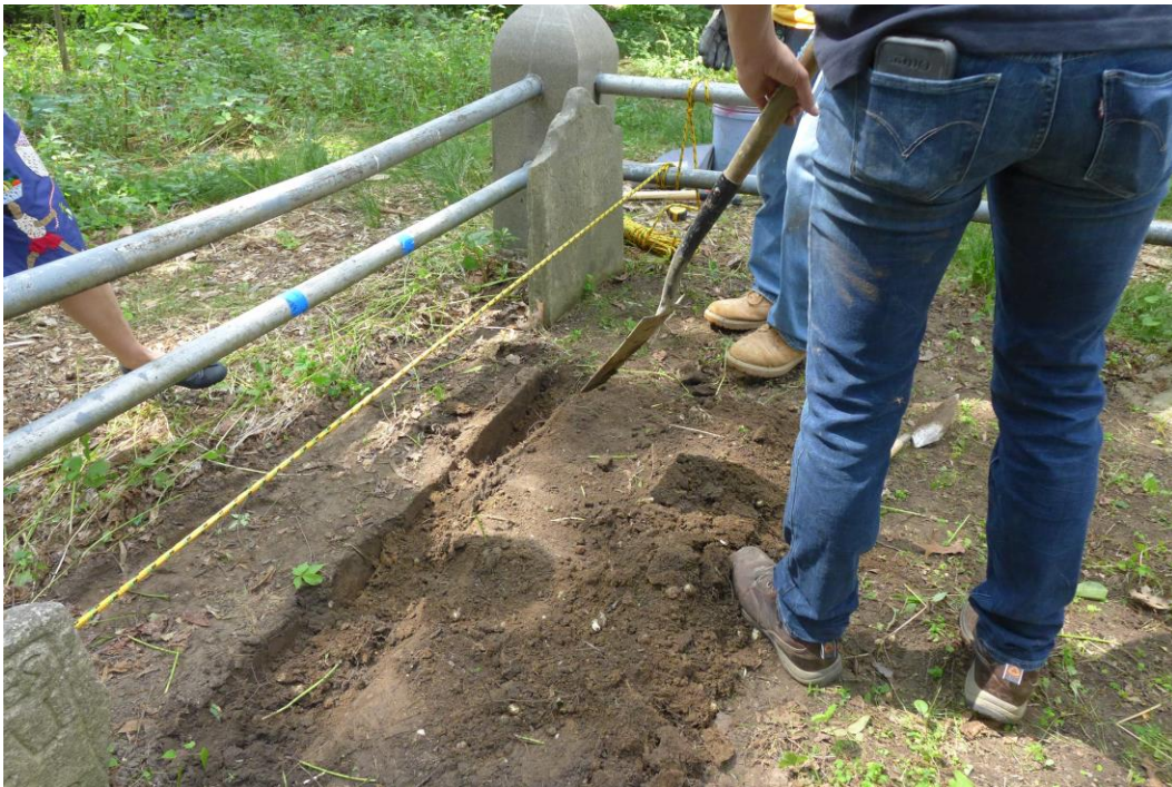
Image 08: Excavating for the installation of the conserved tombstone
