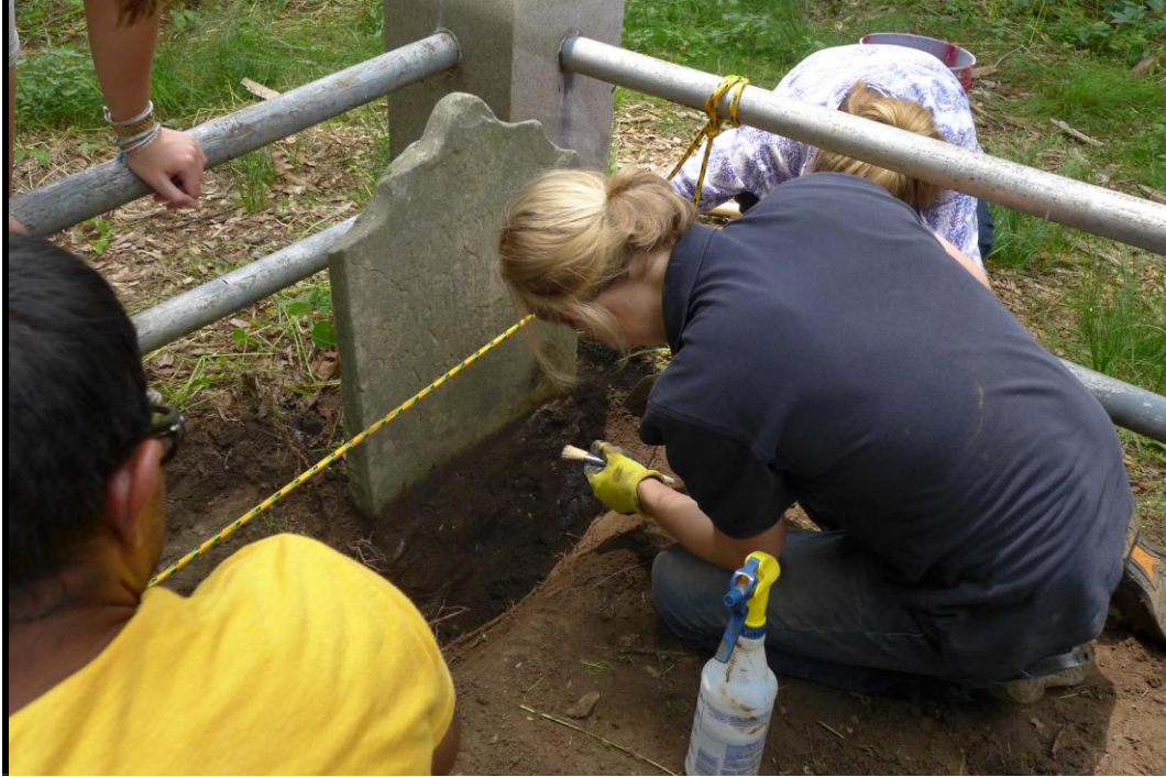
Image 11: Re-installation of tombstone.
