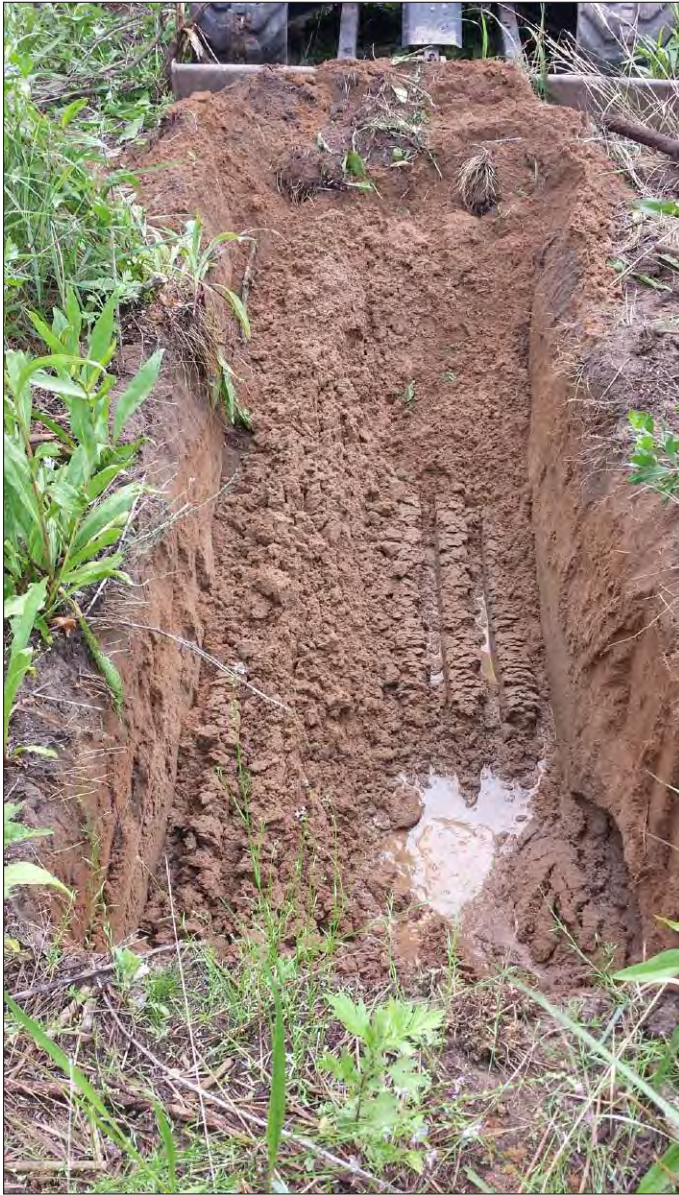
Trench 6 being excavated in a low-lying area near the southern end of the site. Groundwater was observed at a depth of 30 inches (2.5 feet)
