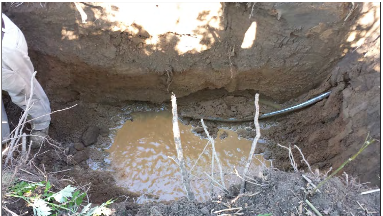
A metal pipe protruding from the northwest corner of Trench 3 at a depth of almost 36 inches (3 feet) and groundwater accumulating at a depth of 52 inches (4.34 feet)
