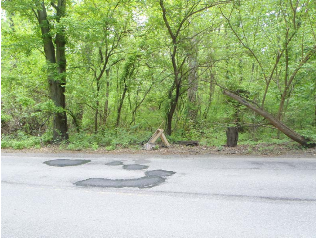
Photo 5. View east of the general location of Test 12 excavated in a wooded area located along the east side of Bloomington Road south of Ramona Avenue.
