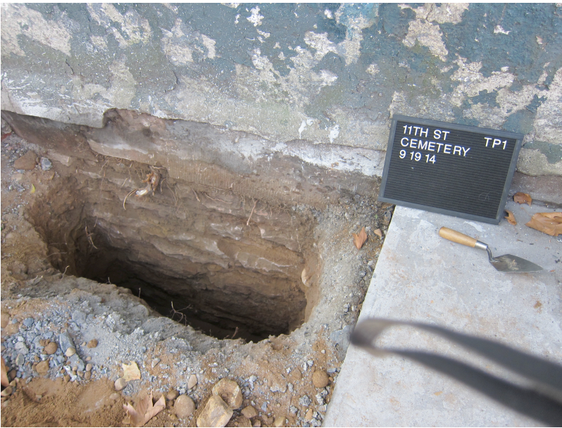
Photo 4. Test excavation along the north side of cemetery wall. Note the rough surface of the foundation stones that have been brushed clean. (9-19-14)
