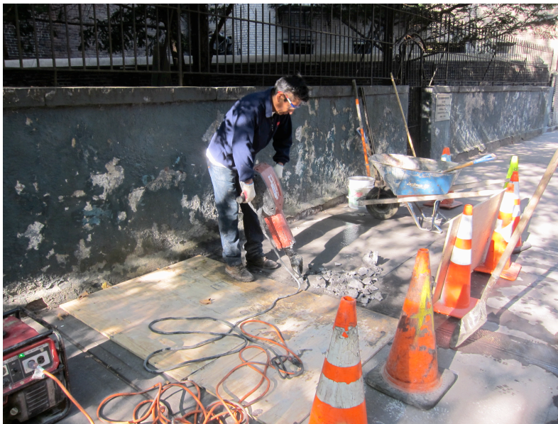
Photo 2. After the cement was cut, a jackhammer was used to break up the sidewalk square. The cement debris was then removed to an awaiting truck. The view is northwest from the north side of the cemetery wall. (9-19-14)
