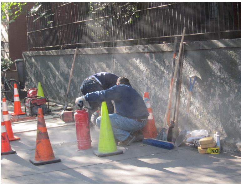
Photo 1. Cutting sidewalk cement, the first step in accessing the excavation area. The view is southeast from the north side of the cemetery wall. (9-19-14)
