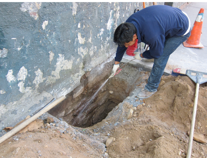
Photo 6. The exposed stones were then washed with water from a spring pump. (9-19-14)
