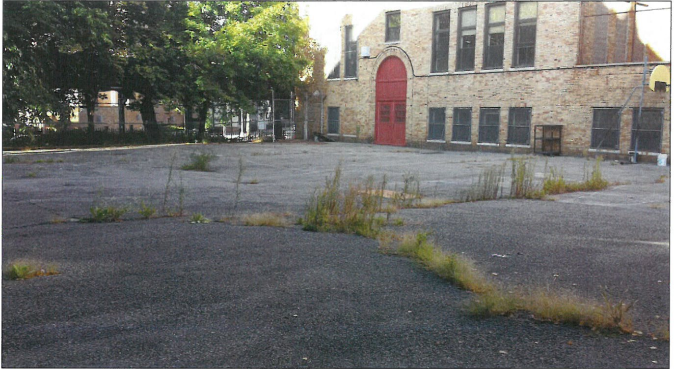
Looking southwest across the paved play area to the rear of the school (in background). Storm water drains and utility vaults are visible in the pavement in the center of the photograph 1
