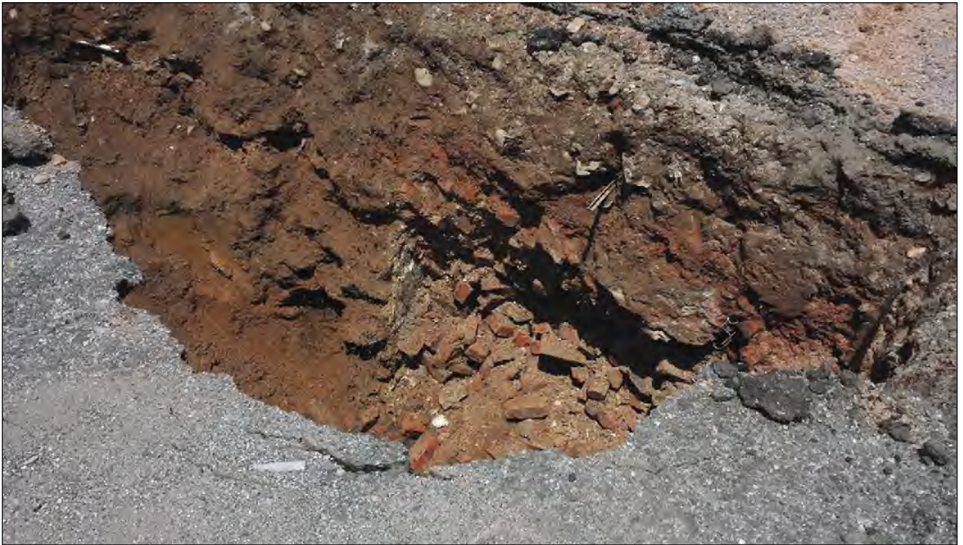
The northern wall of Trench 3.3. The undocumented basement foundation is to the right (east) of the photograph and clean sandy soil is to the left (west)
