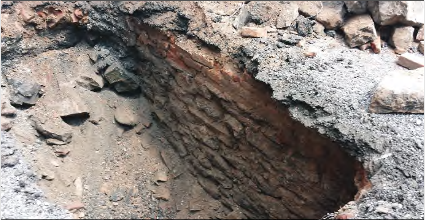
Brick and stone foundation wall lining the eastern wall of Trench 2.5
