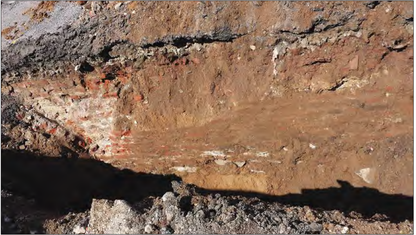
A brick foundation wall along one wall of Trench 3.2. Clean dark yellowish brown sand is visible at the bottom of the trench, beneath the depth of the wall
