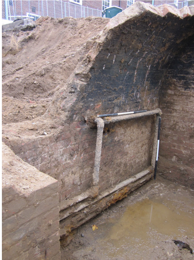
Photo 5 Feature 1 after removal of interior fill showing the pipes present along the eastern wall and soot along the interior of the roof, facing southeast (Image 1470: October 25, 2012).
