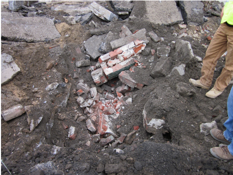
Photo 11 Sections of mortared brick demolition debris and broken pavement exposed in the vicinity of Feature 3 as the then existing parking lot was being removed, facing northwest (Image 1305: October 15, 2012).
