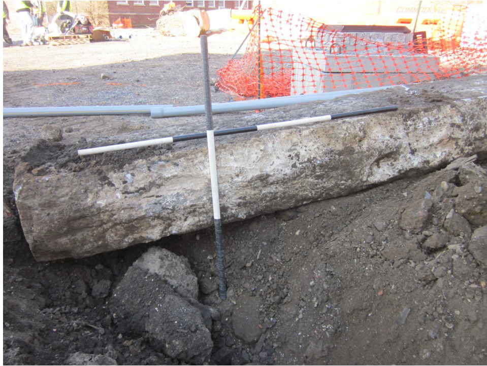
Photo 15 Large previously displaced granite foundation-type stone found during excavation monitoring of an electric trench in Tile 13 - South Battery Zone (Image 2778: April 8, 2013).
