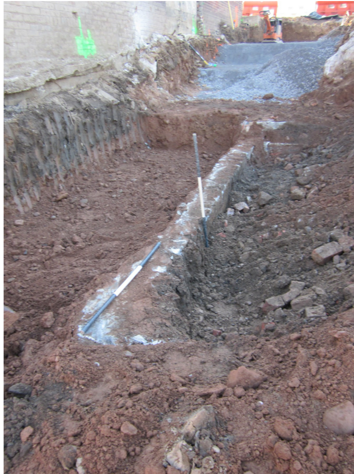
Photo 9 Completed excavation of the G wall footing segments 1 and 2 showing the portion of the eastern side of Feature 2 that was preserved, facing south (Image 1789: January 7, 2013).
