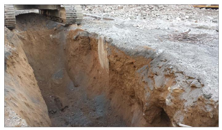
A support pier and fill deposits encountered during the excavation of Trench 2 showing disturbed fill deposits typical of those seen elsewhere on the site
