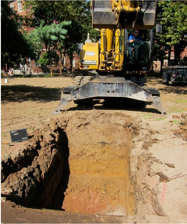
Photo 1. (above) East wall of LP19. The gray sand in the upper left corner is evidence of a previously backfilled utility trench. The “yellow” sand next to and below the trench is old park fill (an animal bone was found below the trench fill). See Figure 4e for a schematic profile. (Geismar 7-10-12)
