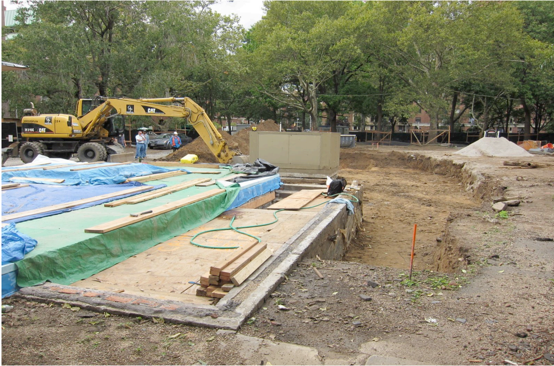
Photo 5. Former comfort station after demolition (foreground). Its foundation and basement (under plywood and tarps) will be incorporated into the new building. Excavation of the shallow trench (CSF) for the new building's slab (right and rear) was monitored. The view is looking west. (Geismar 9-20-12)
