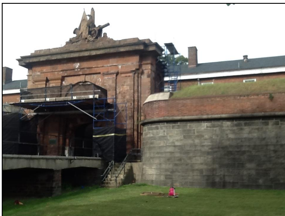
Figure 14. Looking southwest at Dry Moat -- North of Bridge Area. STP 1 (coordinates N 0/E+1; the northwestern corner is in line with the North datum and 1 m [3.2 ft] to the east of it) is being excavated.
