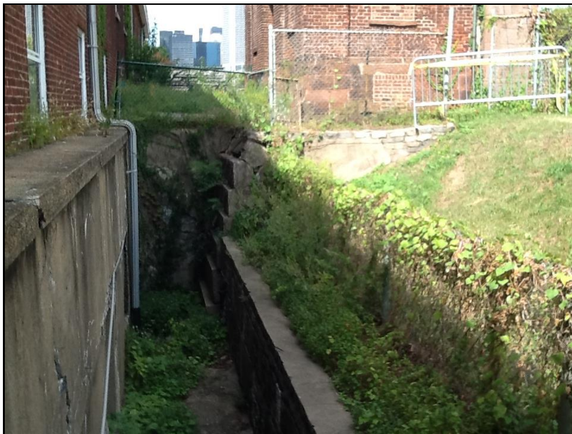
Figure 22. Guardhouse Area, looking north, with areaway in foreground. Note condition of retaining wall below hurricane fence. Photograph taken in September 2014.
