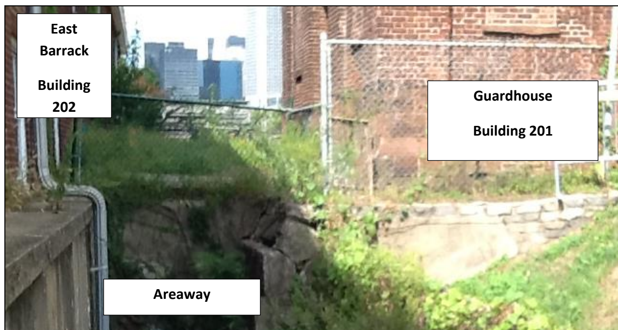
Figure 11. Guardhouse Area, looking north. Note condition of retaining wall.
