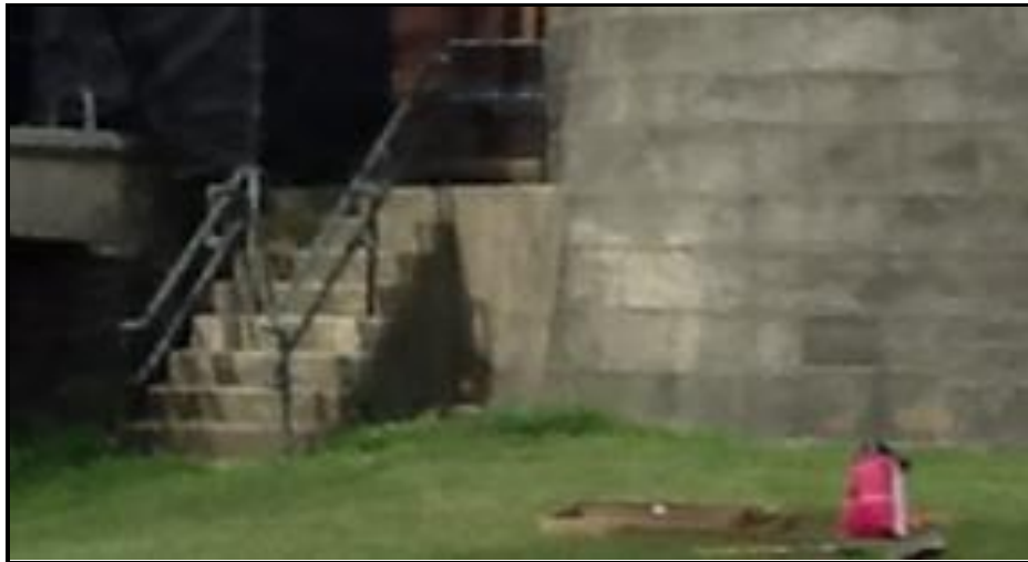
Figure 7. Dry Moat – North of Bridge Area, looking southwest.
