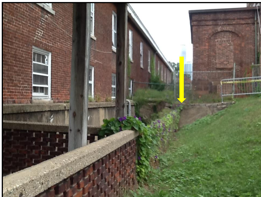
Figure 20. Looking south towards Guardhouse Area. Building 201, right; eastern wall of Building 202, left. Unit A excavated at arrow.
