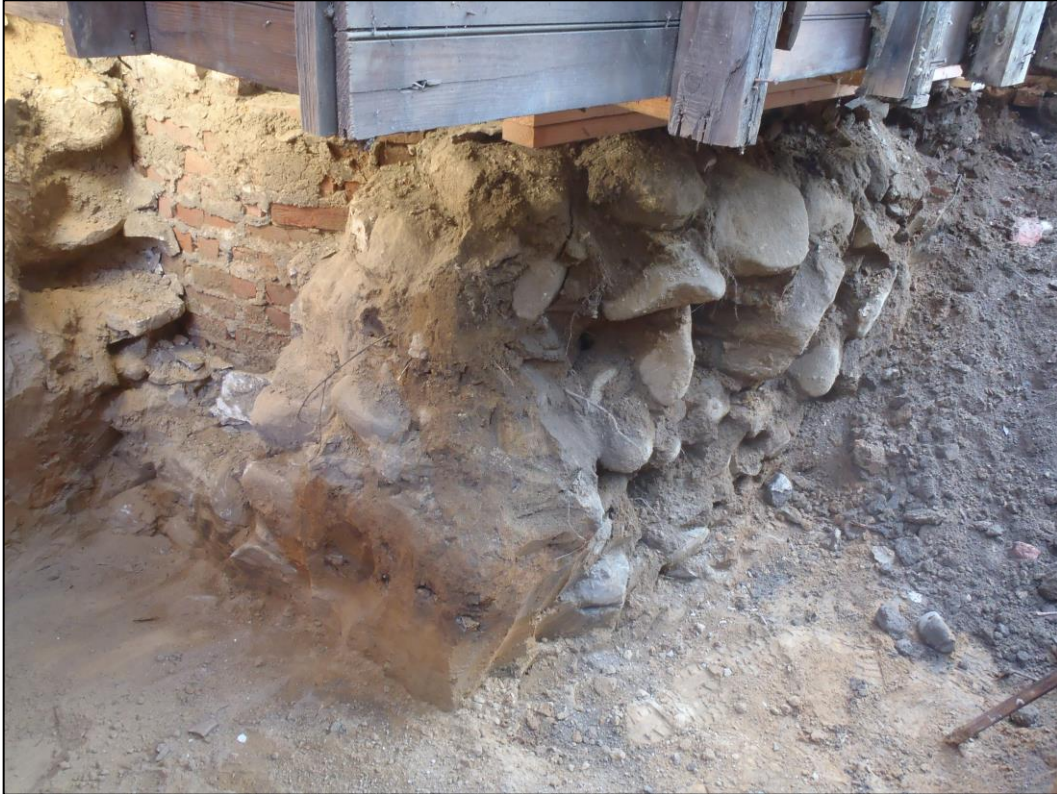
Image 16: Trench 3 showing the Feature 1 cistern and surrounding foundation stones.
