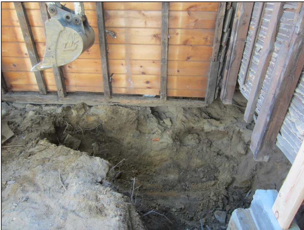
Image 60: Trench 2 – Excavation adjacent to Room 113 east wall/Room 115 north wall.
