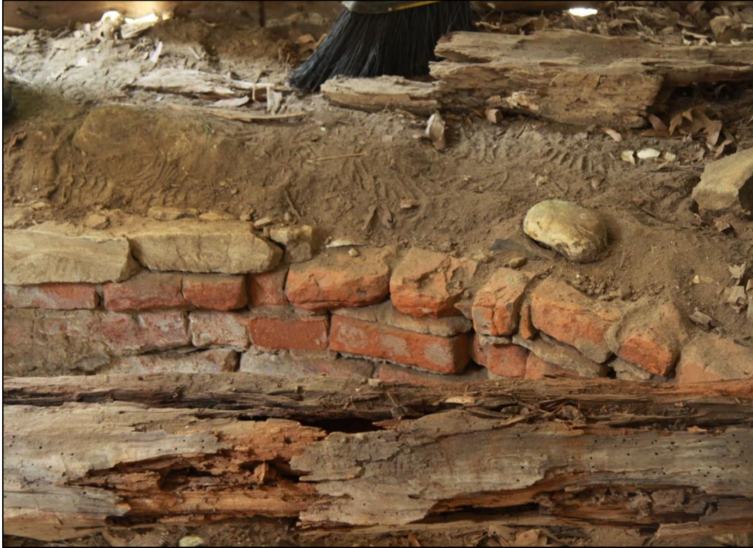
Image 47: Feature 1 – interior south wall of cistern.
