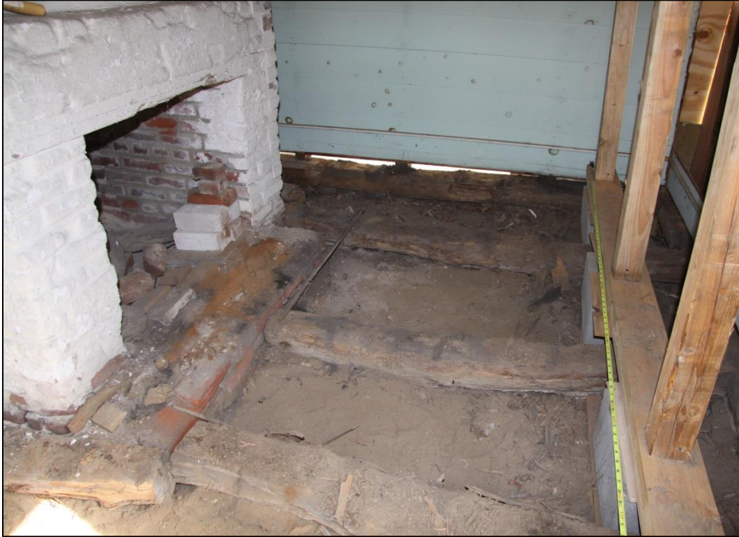
Image 49: Room 115 - Domed oven in NW corner of the room with adjacent joists.
