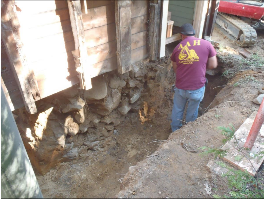
Image 39: Trench 3 – Excavation in progress; southern house exterior, Room 115 foundation stones in profile.
