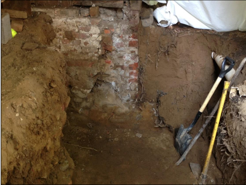
Image 21: Trench 2 – West profile, brick foundation of Room 104.
