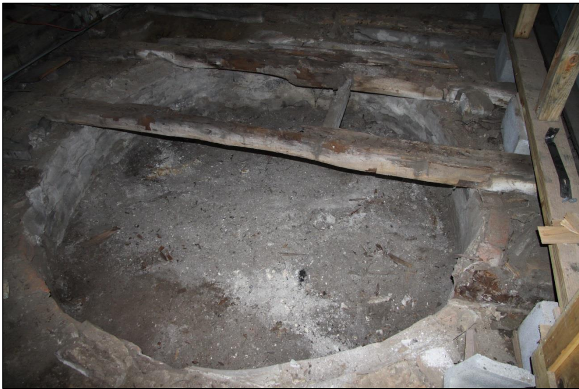
Image 52: Feature 1 – Floor joist removal in progress.
