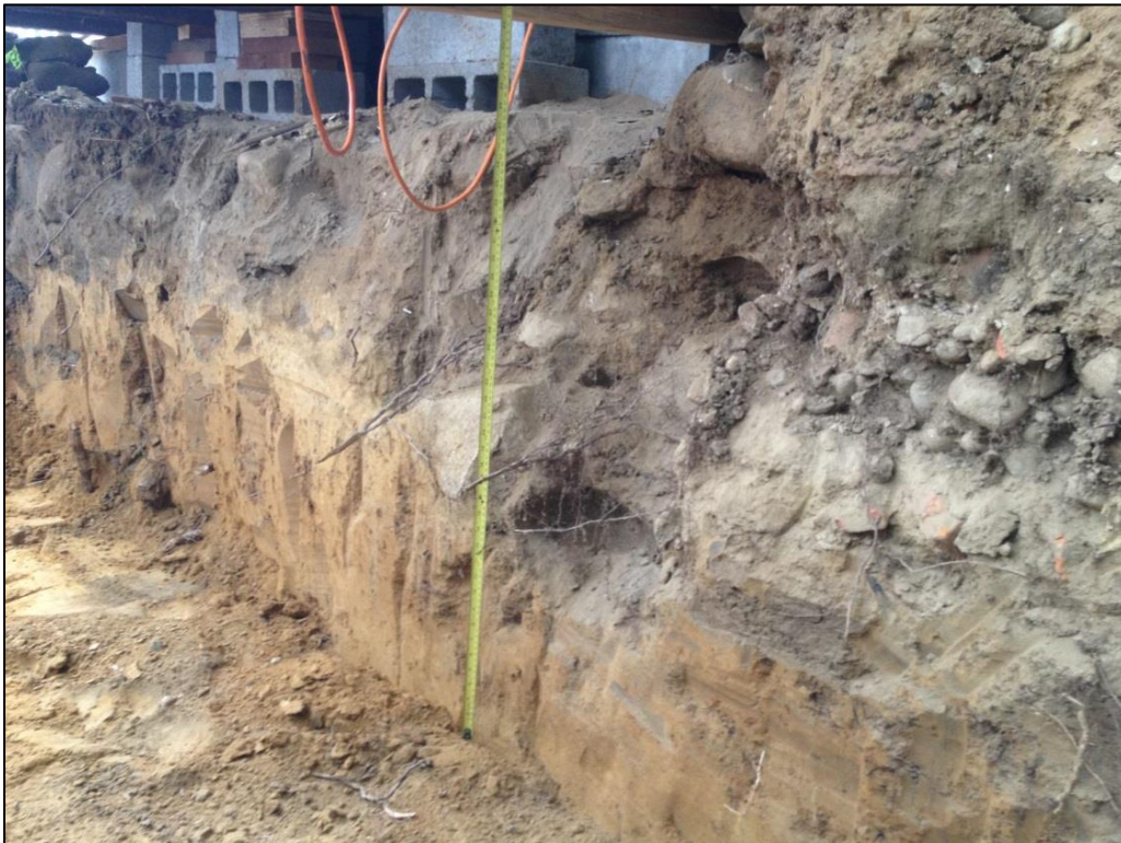
Image 26: Trench 2 – South profile, adjacent to Room 113 and 111.
