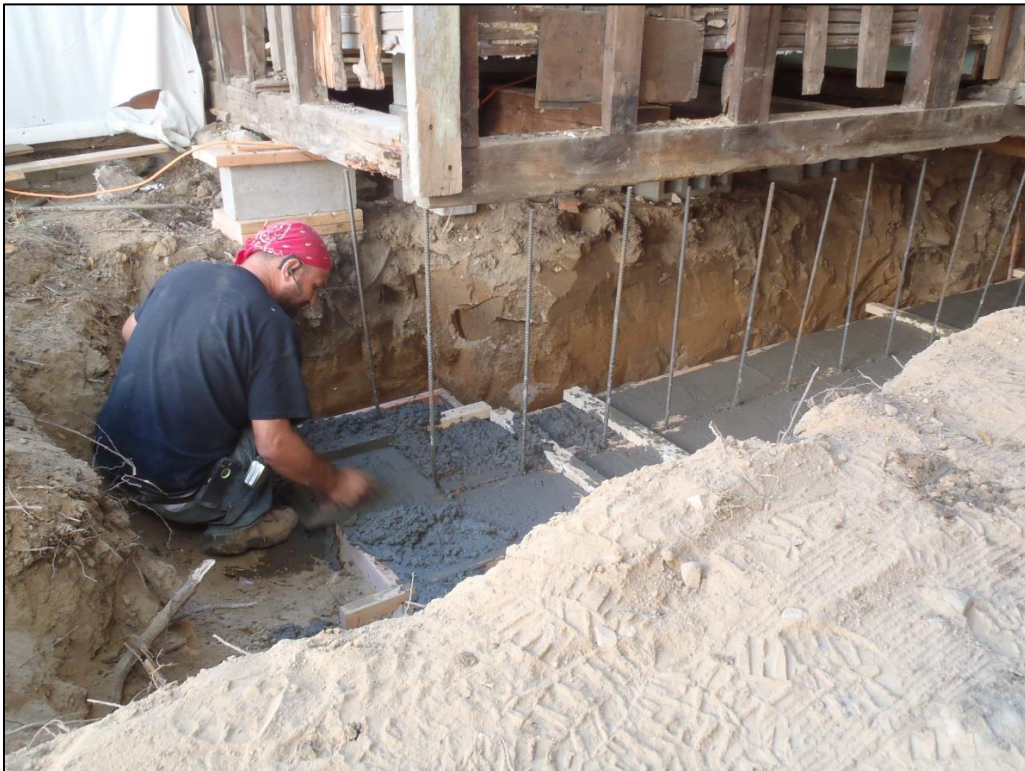
Image 34: Trench 2 – Concrete foundation poured; adjacent to Room 113.
