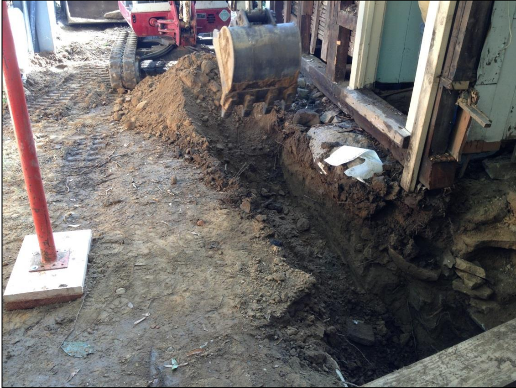
Image 23: Trench 2 – Excavation in progress; adjacent to Room 113.
