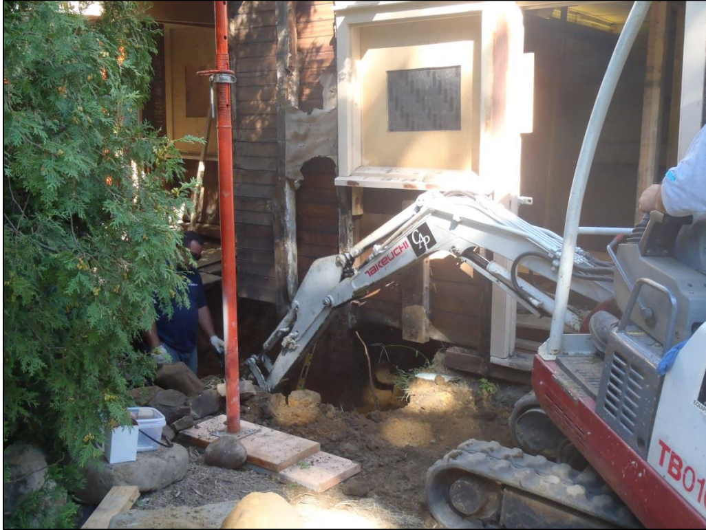
Image 35: Trench 3 – Excavation in progress; southern house exterior, adjacent to south wall of Room 115.
