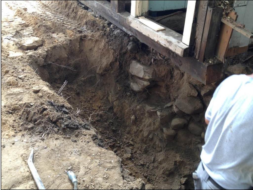
Image 25: Trench 2 – Excavation in progress, foundation in profile; adjacent to north wall of Room 113.
