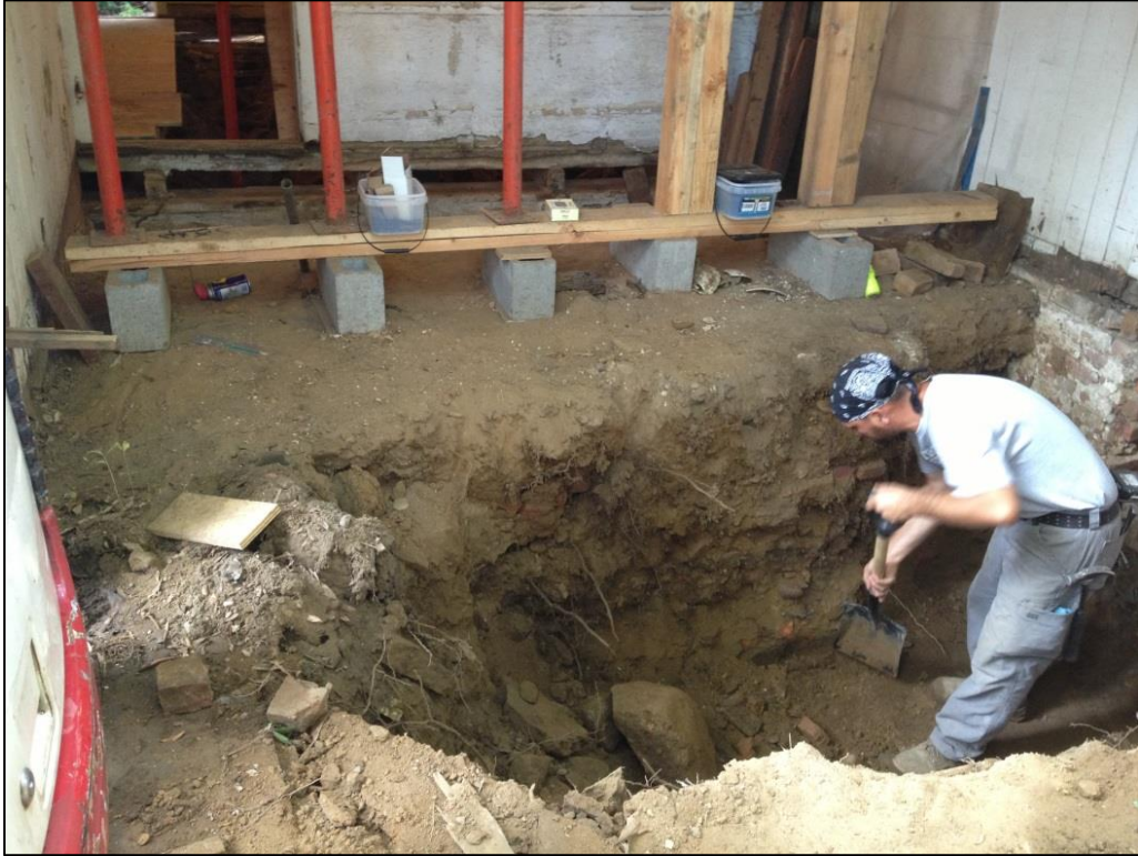
Image 19: Trench 2 – South profile, excavation in progress; adjacent to Room 111.
