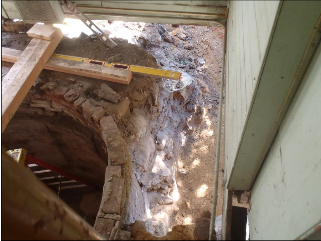
Image 33: Room 115 interior, view of Feature 1 and west wall of Room 115 following removal of foundation stones.
