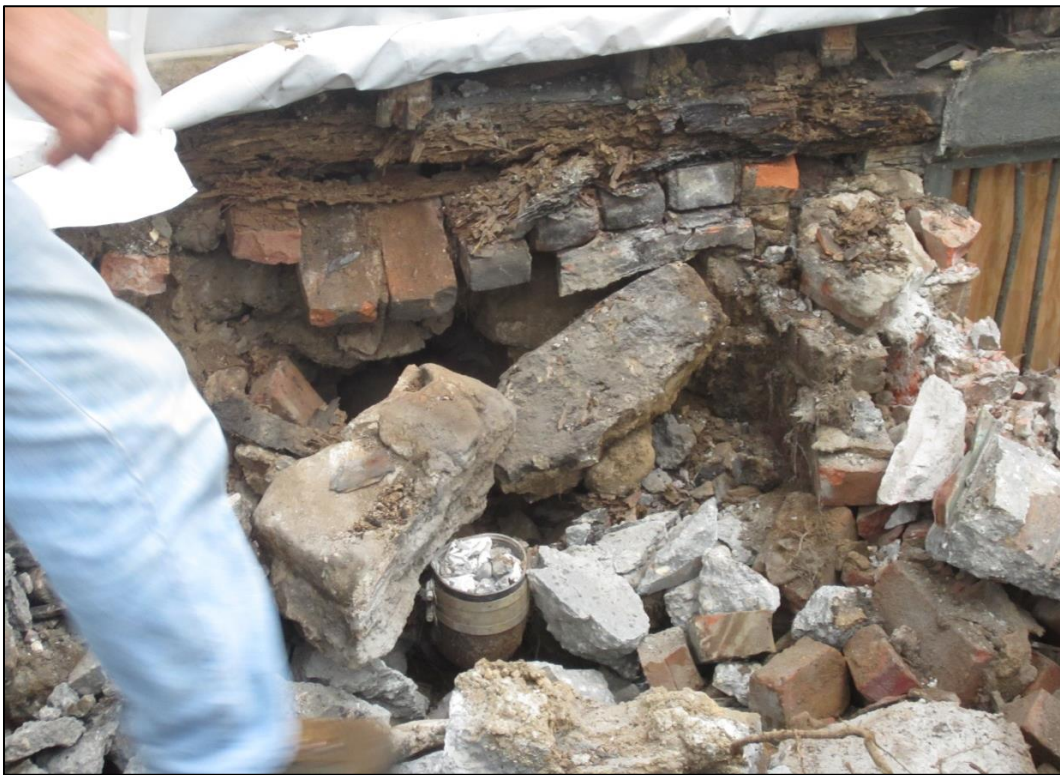
Image 58: Trench 4 – Excavation in progress, rubble fill from Room 104 west foundation.
