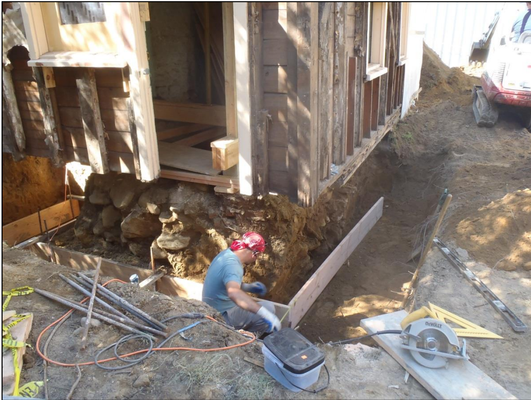
Image 42: Trench 3 – Form for concrete foundation; adjacent to Room 115.
