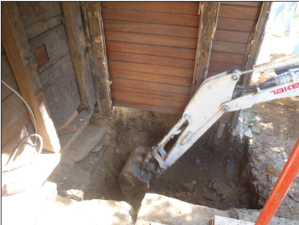
Image 30: Trench 3 – Excavation in progress; southern house exterior, adjacent to west wall of Room 115.
