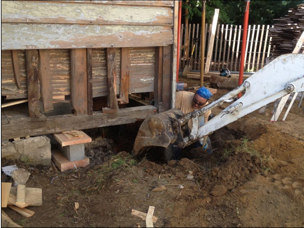
Image 27: Trench 2 – Excavation in progress; adjacent to east wall of Room 113.
