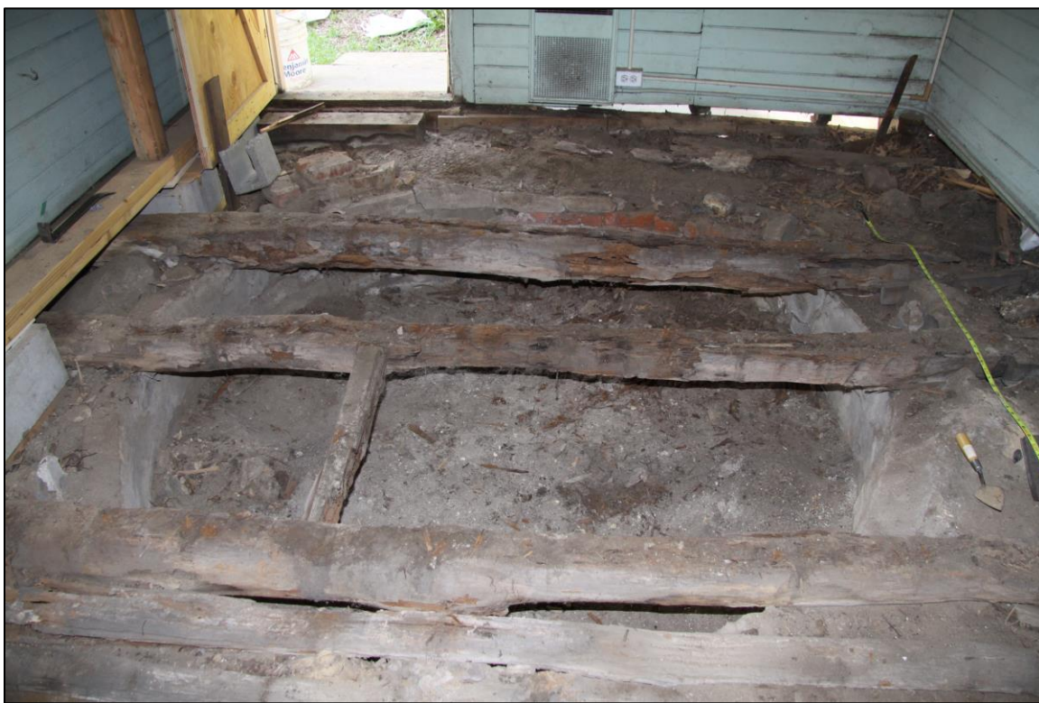
Image 04: Feature 1 – Opening plan view beneath wooden floor joists.
