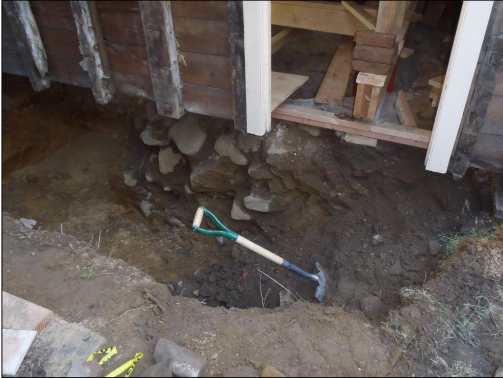
Image 37: Trench 3 – Excavation in progress; southern house exterior, Room 115 foundation stones in profile.
