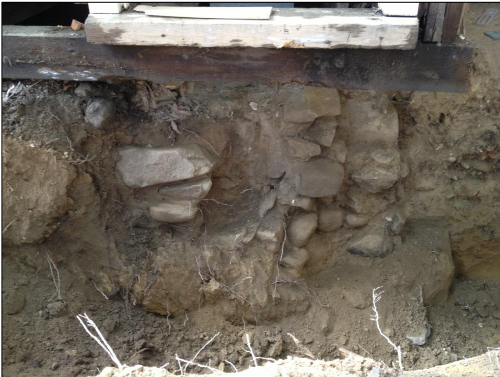
Image 24: Trench 2 – South profile, stone foundation in profile; adjacent to Room 113.
