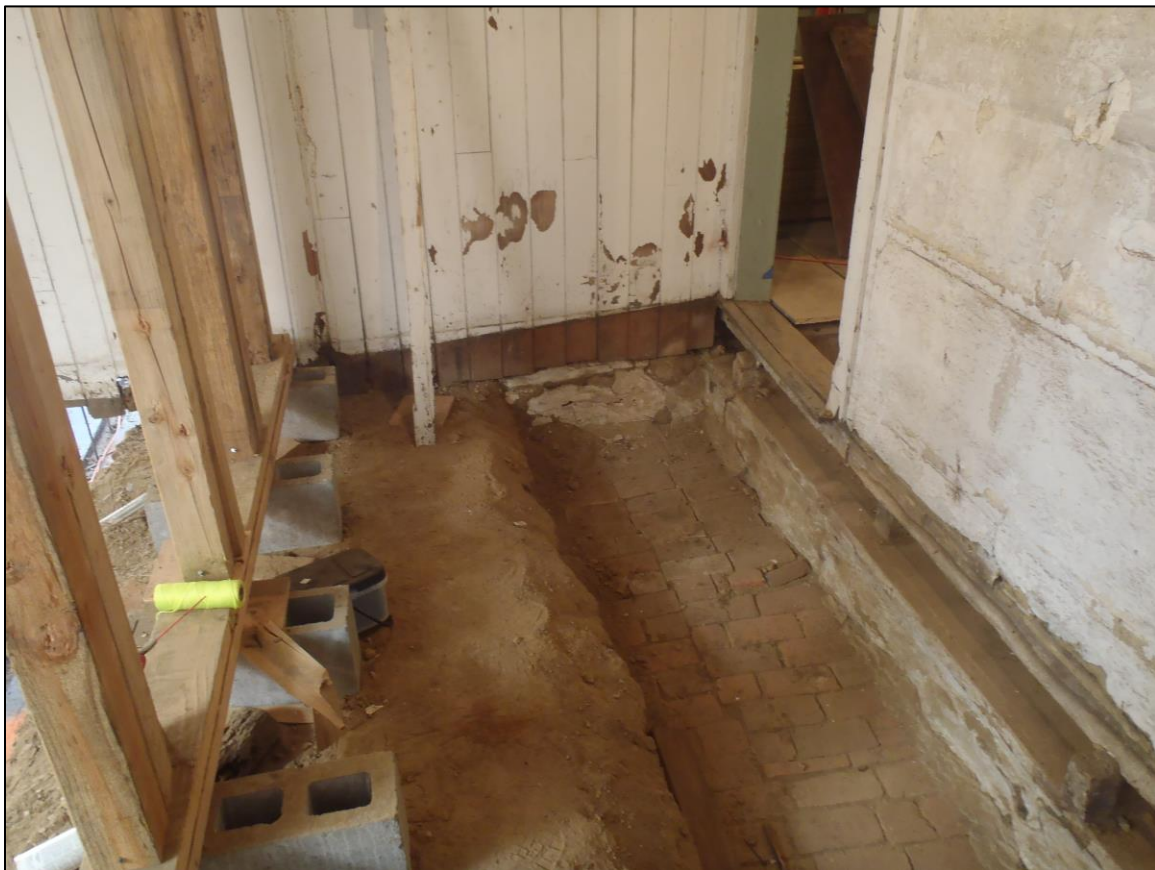
Image 13: Room 111 – exposed brick floor.
