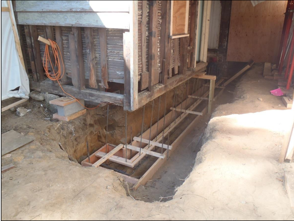
Image 29: Trench 2 – Form for concrete foundation; adjacent to Room 113.
