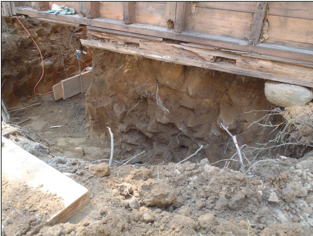
Image 40: Trench 3 – West profile, excavation in progress; adjacent to east wall of Room 115.
