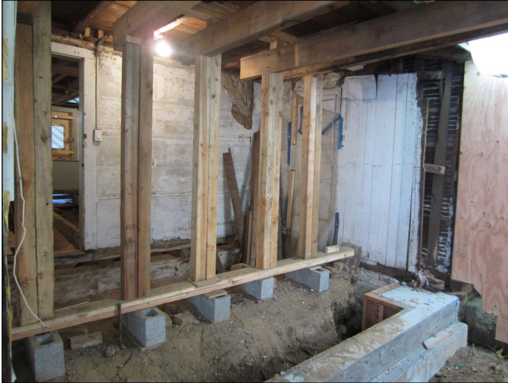
Image 59: Trench 2 – Concrete foundation and porch (Room 111).
