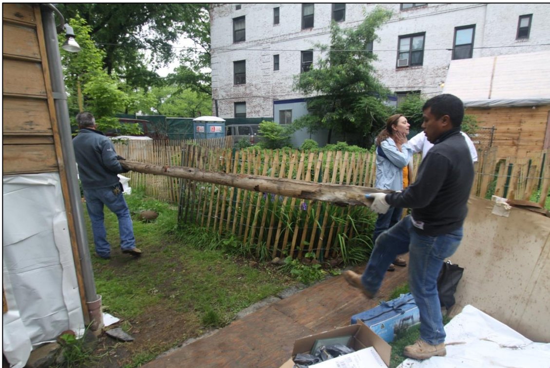
Image 54: Floor joist removal in progress.
