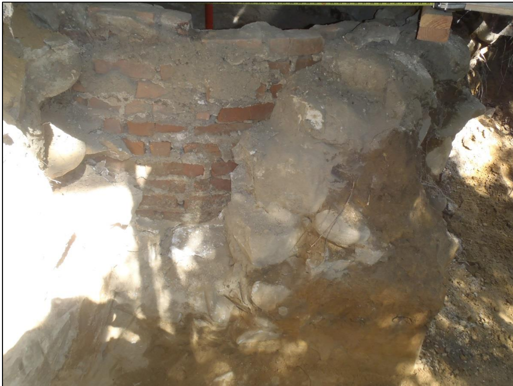
Image 36: Trench 3 – Exterior of Feature 1, beneath west wall of Room 115.
