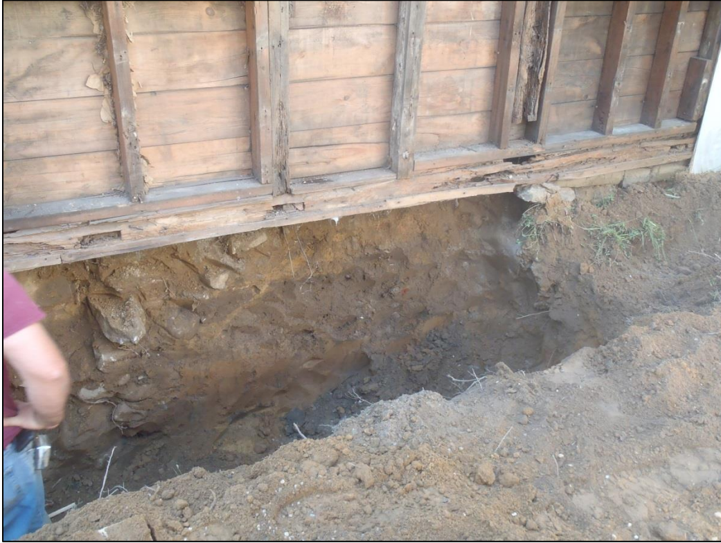
Image 41: Trench 3 – West profile; adjacent to east wall of Room 115.
