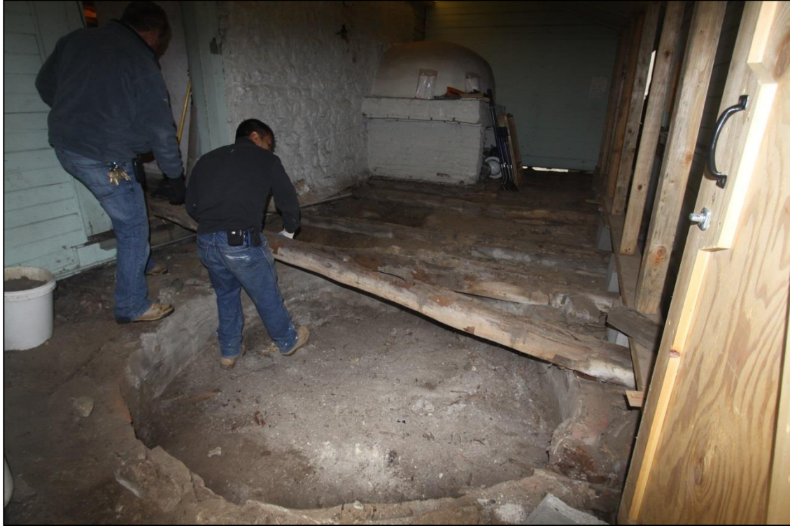
Image 53: Feature 1 – Floor joist removal in progress.
