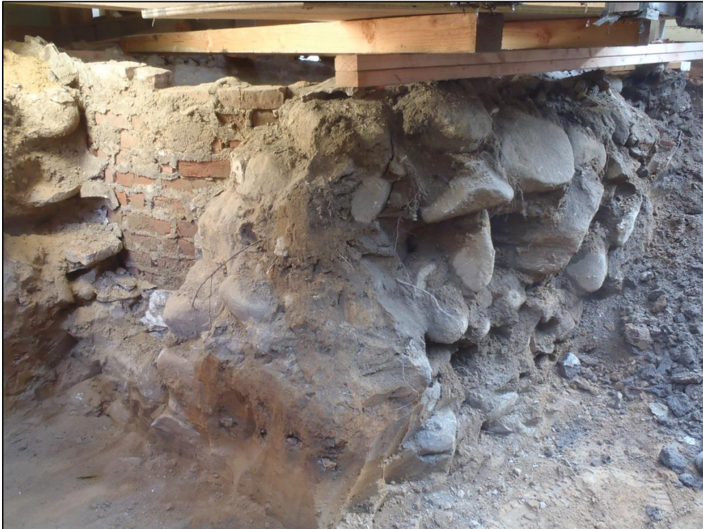
Image 38: Trench 3 - Feature 1 and Room 115 foundation stones in profile.
