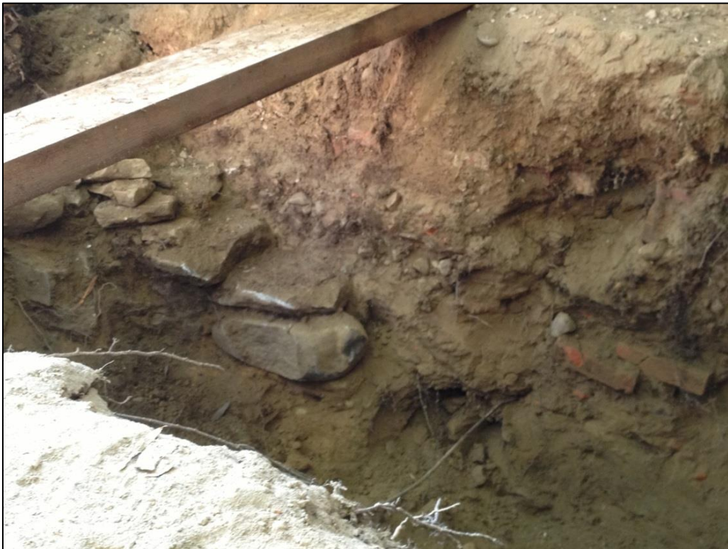
Image 22: Trench 2 – South profile, stone foundation in profile; adjacent to Room 111.
