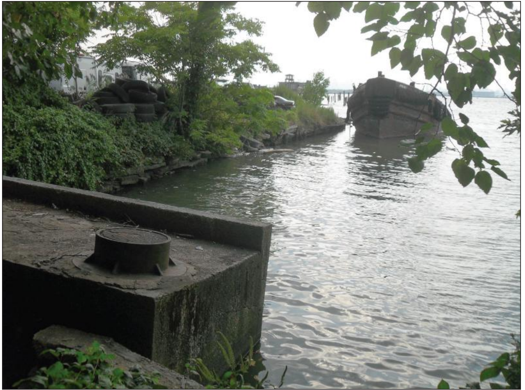
View of abandoned boat and shoreline with rip rap, facing west 11
