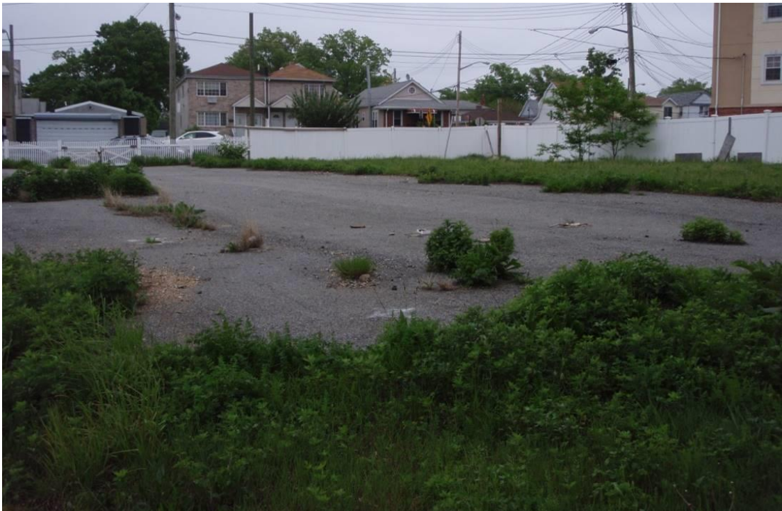
Photo 2: View of the cracking blacktop taken from the northwest corner of the site, facing southeast. Photograph taken by K. French 5/18/2015.
