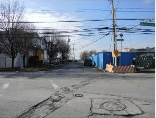
Photograph 24: Existing Woodrow Road at Bloomingdale Road intersection. Note multiple utilities under roadway. View looking west.
