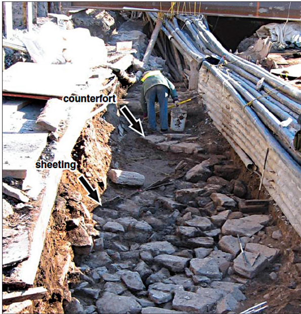
Figure 11. Wall 3 showing the counterfort and white pine sheeting. The buttress might have reinforced the Wall against enemy fire, while the sheeting may have reinforced it from the elements.
