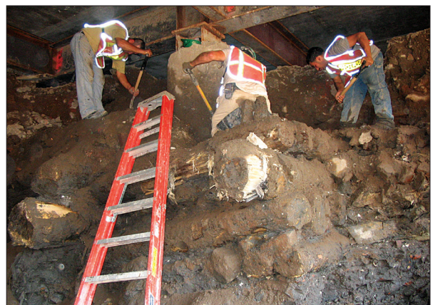
Figure 44. Construction workers clear off soil at the top of the cribbing.
