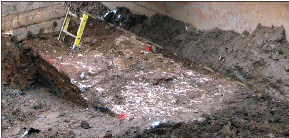
Figure 8. Wall 2 was a small segment of the Battery Wall that had been demolished during construction of Battery Park.
