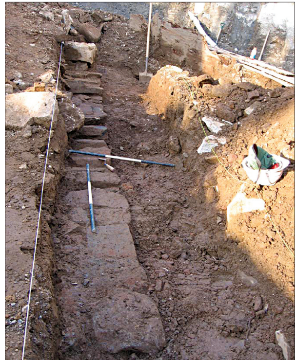
Figure 10. The exposed eastern face of Wall 3 under street utilities which can be seen at the top of the frame near the shovel.
