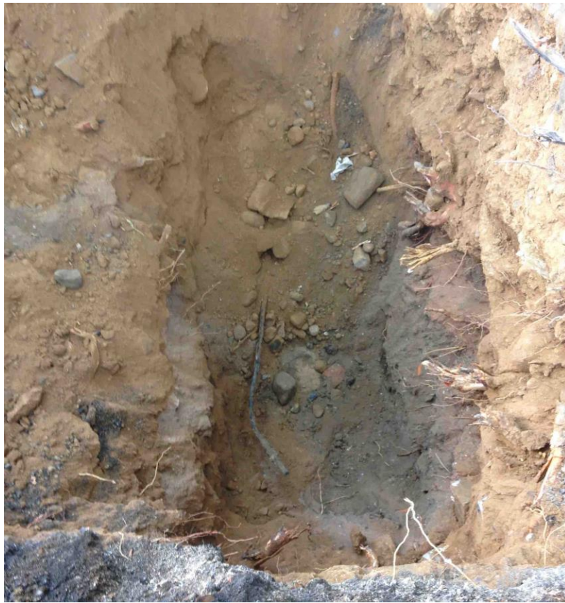
Photograph 8. Utility Pipe in Trench C.
