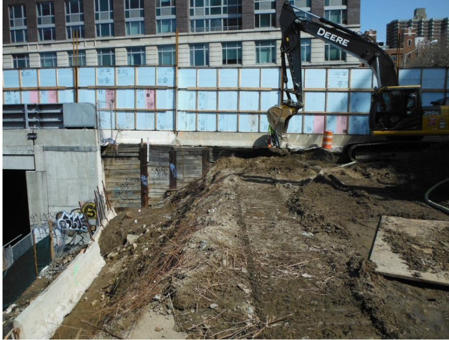
Figure 4.82. Looking north within the east side of Parcel 2, during removal of the uppermost twentieth century fill sediments. 61st Street lies behind the light blue construction fencing.
