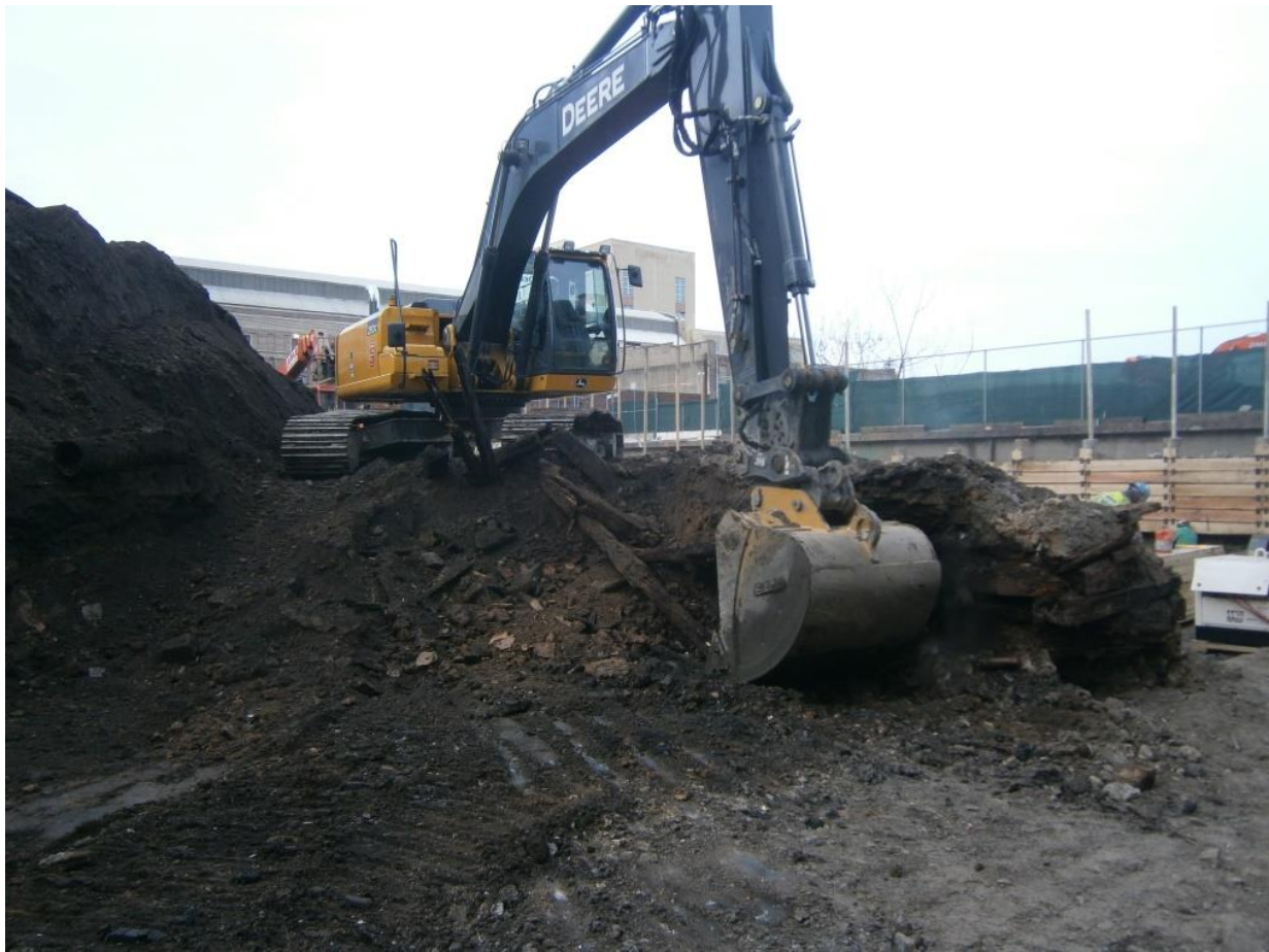
Figure 3.4. Large excavator removing sediment in Sensitive Area 1.
