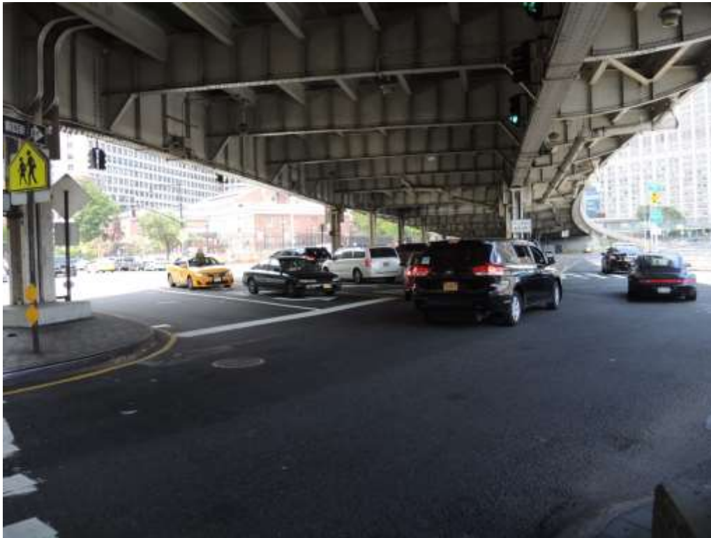
Photograph 1: East 23 rd Street intersection with the FDR Drive overpass. View looking northwest.
