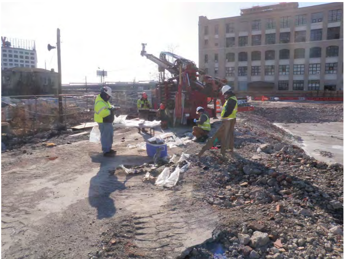
Plate 3. View of the soil boring process monitored by archaeologists. The extracted sediment tubes are in the foreground.
