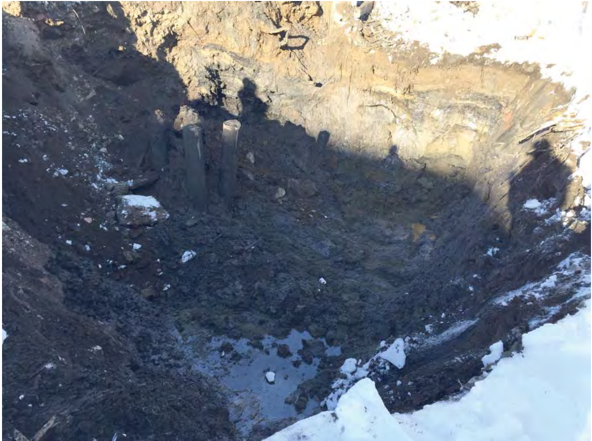
Plate 6. View of Trench 3 (looking east) profile with a final depth of approximately thirteen feet below ground surface. The cement cylinders standing upright to the left of the profile are micro-piles.
