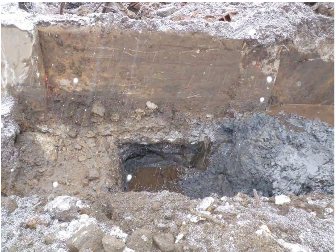
Plate 7. View of Trench 4 (looking west) with a window dug to approximately ten feet below ground surface. The water inundation was problematic in this trench.
