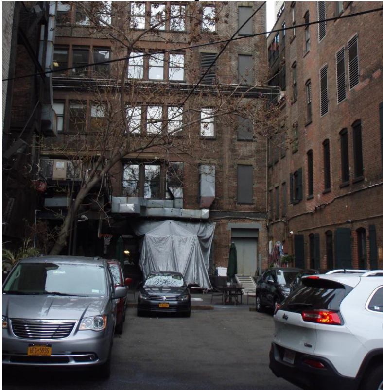
Photograph 4 - View of the courtyard behind the archaeological-APE, looking north
