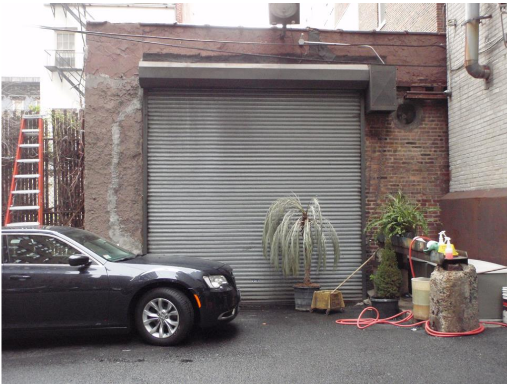
Photograph 2 – View of the rear exterior of the building, taken from the asphalt courtyard behind the building and facing south.
