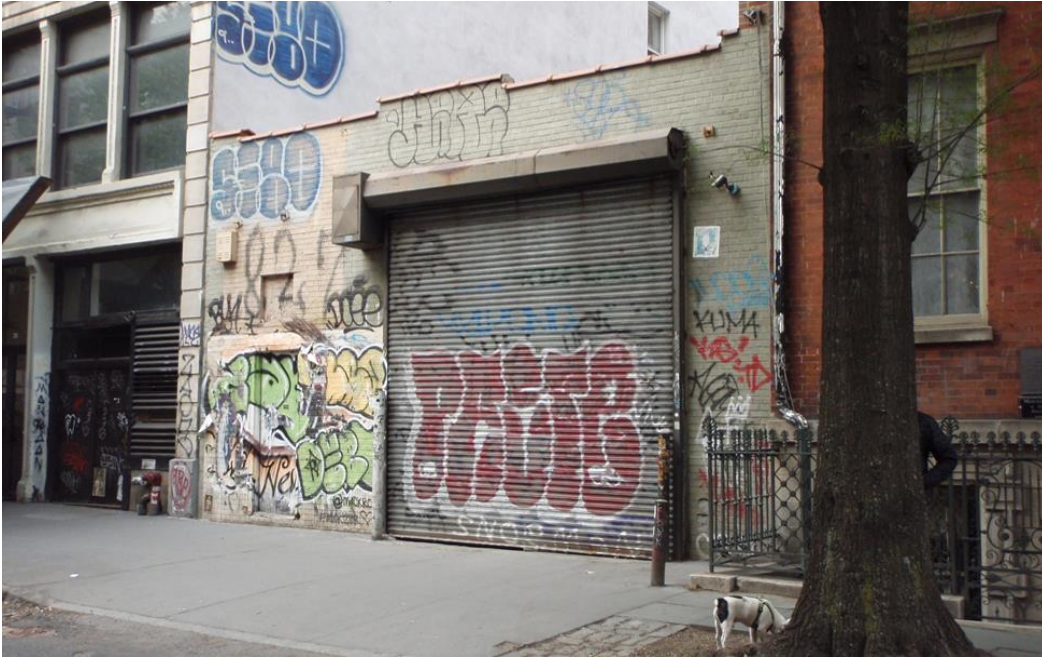
Photograph 1 - View of the front building entrance on East 4th Street, facing northwest. The Merchant House Museum is the red brick structure located to the right of the image.
