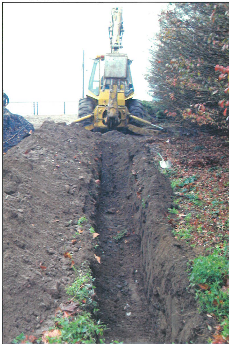
PHOTOGRAPH 6: Trench 4 and Feature 5, View East
