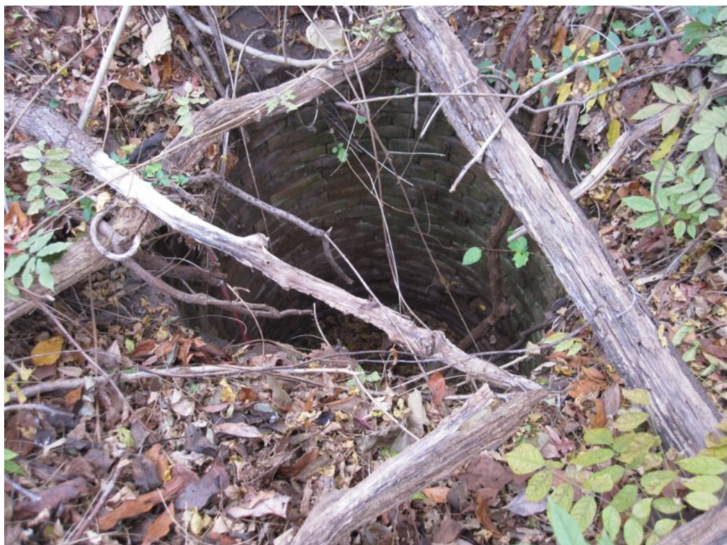
Photo 7. A brick well (B2), approximately 5 feet (1.5 m) in diameter, was originally identified as a cistern (JMA 2000, 2005). However a soil boring revealed that it extended down more than 31 feet (9.5 m) BGS to an unknown depth and was instead a well. (Photo: B. Seamans 11-19-2015).
