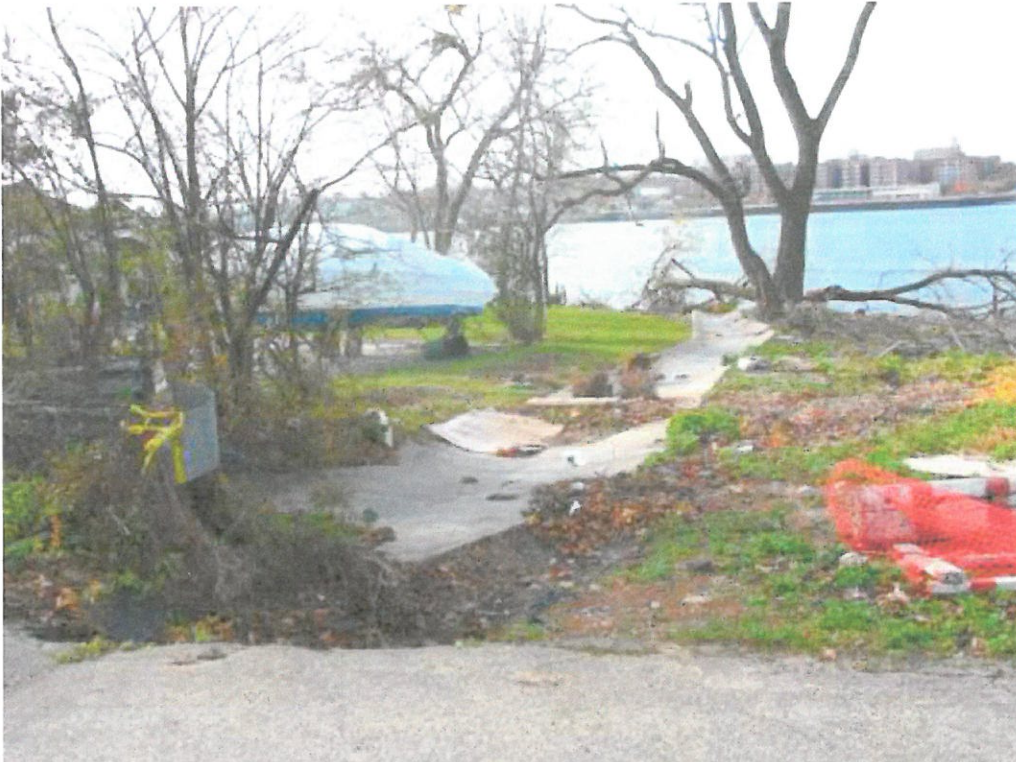
Photograph 1: Project site section from the intersection of Amboy Road and Wards Point Boulevard to the beach, showing concrete drainage culvert or swale. View looking west from Amboy Road terminus.
