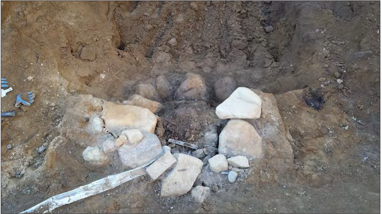
The top of the well on Lot 42 before excavation; the lead pipe is at the left 13
