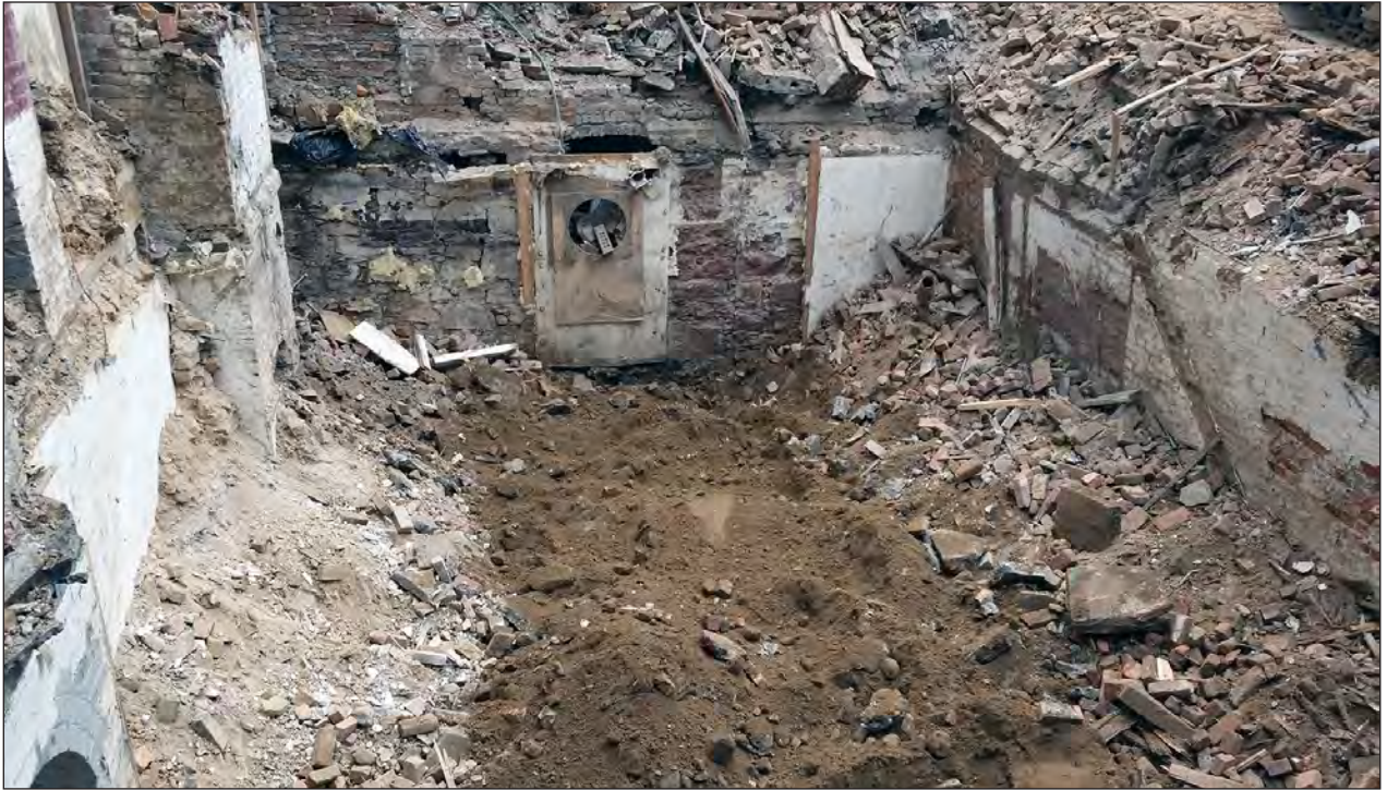
View east of the sub-cellar cavity showing the north (left), east (center), and south (right) walls of the foundation of the former building at 233 Duffield Street. The arched doorway to the stone ventilation shaft is covered with plywood in this photograph
