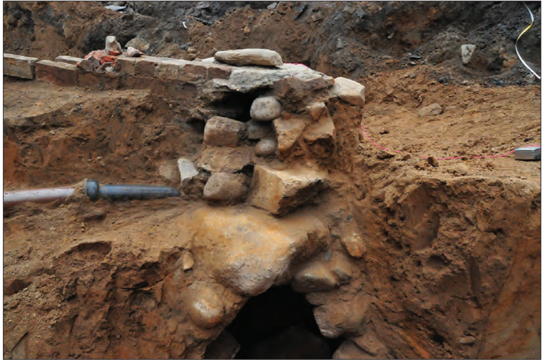
The northern façade of the intact stone cap of the well on historic Lot 45 before excavation. 23 The missing stones at the bottom of the wall collapsed inward prior to the start of the Phase 2 work
