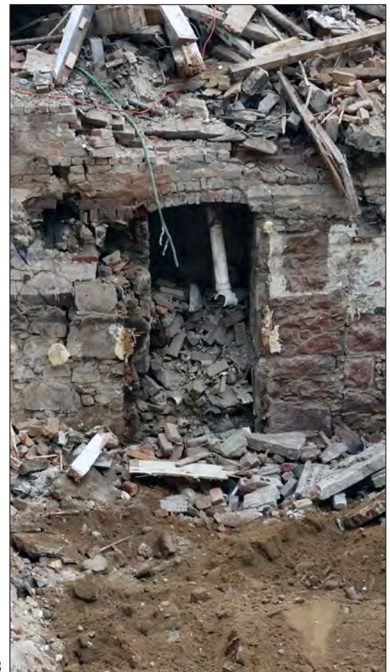
View east of the sub-cellar cavity showing the north (left), east (center), and south (right) walls of the foundation of the former building at 233 Duffield Street. The arched doorway to the stone ventilation shaft is covered with plywood in this photograph
