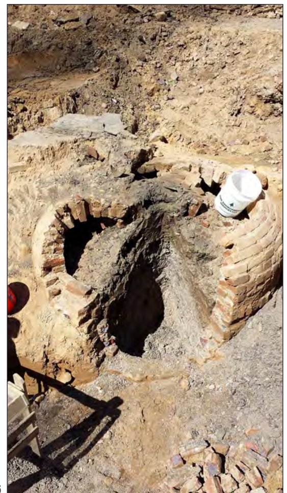
The top of the intricate dome of the cistern on Lot 42 with an intact brick ring in the center 15
