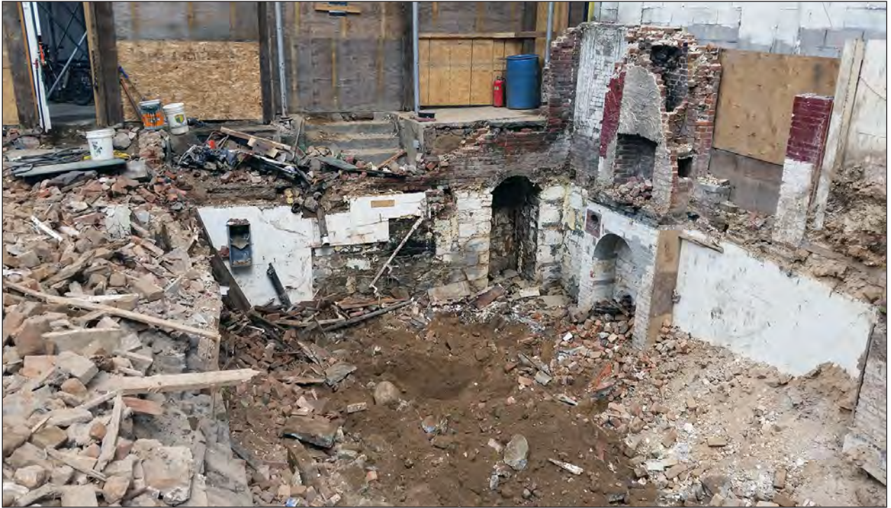
View west at the western (center) and northern (right) foundation walls of the 233 Duffield Street sub-cellar. The arched doorwar to the former coal vault is near the center of the photograph, adjacent to the stacked fireplaces from the sub-cellar (lower) and basement (upper) levels
