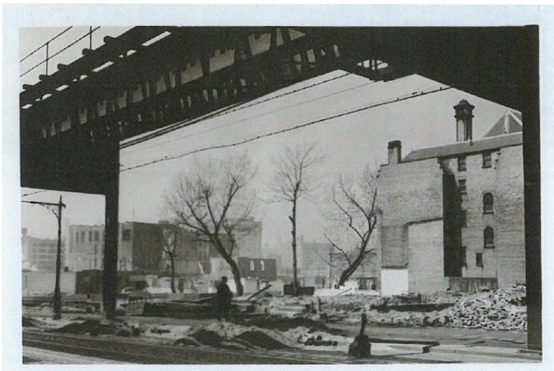
Image 13: Myrtle Avenue - St. Edward's Place (NW Corner, South Face of church after corner buildings demolished) (NYPL 1941).
