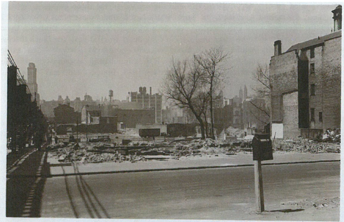
Image 12: Myrtle Avenue - St. Edward's Place (NW Corner, corner buildings demolished, Church Rectory on right) (NYPL 1941).
