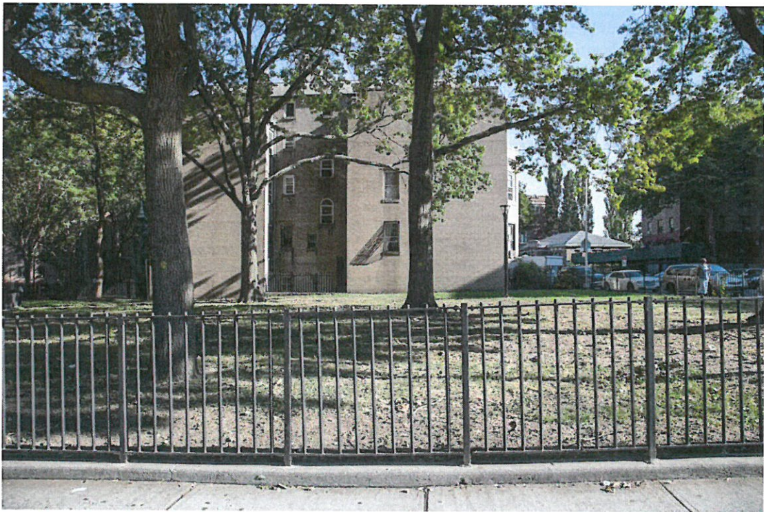
Image 08: Rectory (side view)
