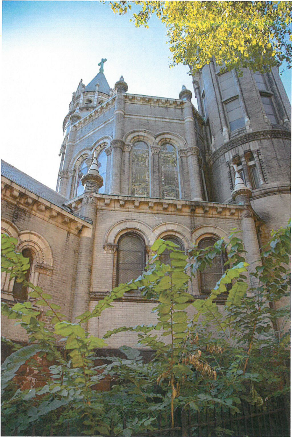
Image 10: Church – existing conditions
