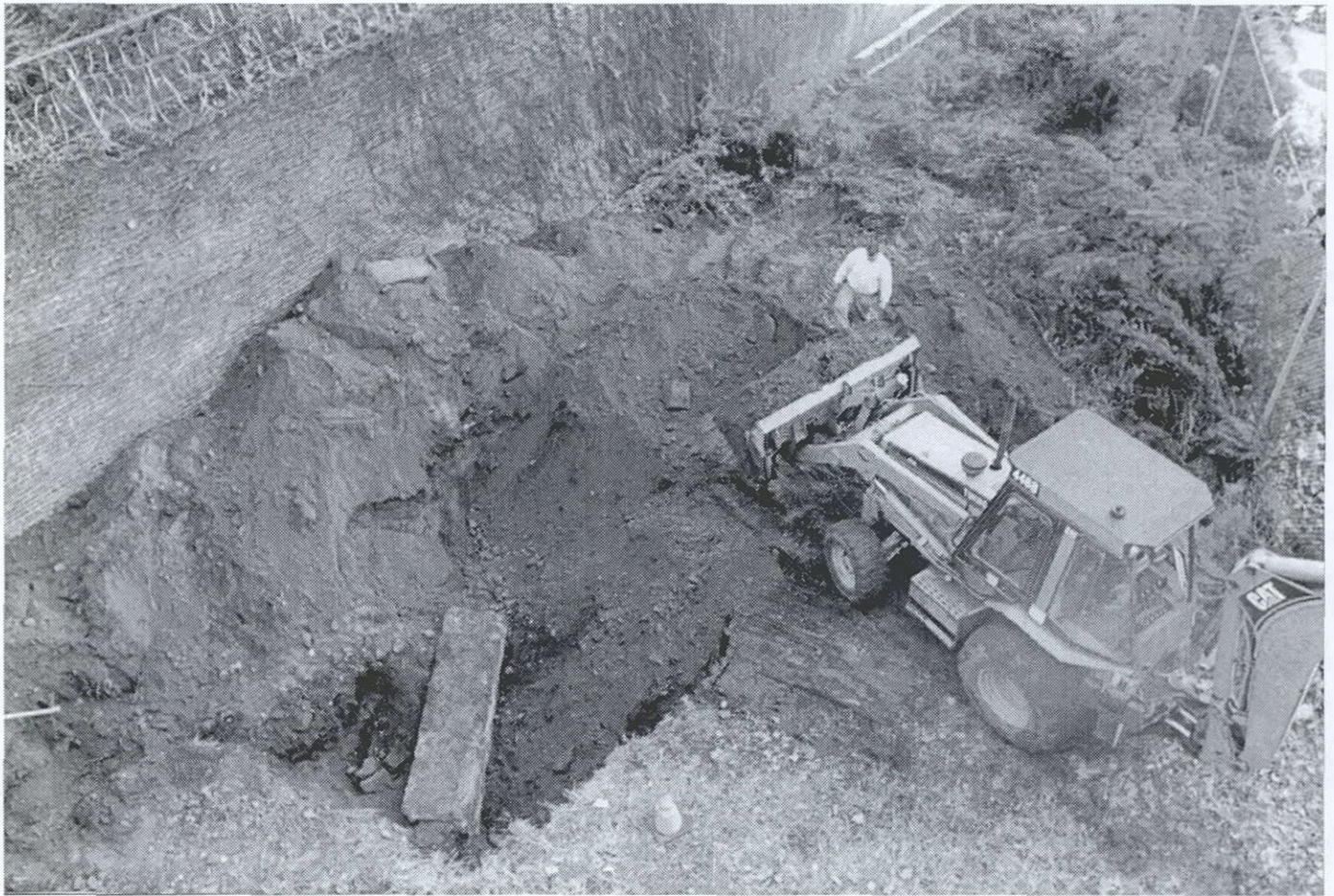
5 "Aerial" view of exposed mortared stone wall from a third floor window of 87 Hudson Avenue. Note angle of wall compared with Navy Yard's brick wall and compare with Figures 2 and 6. (Geismar 11/12/03)
