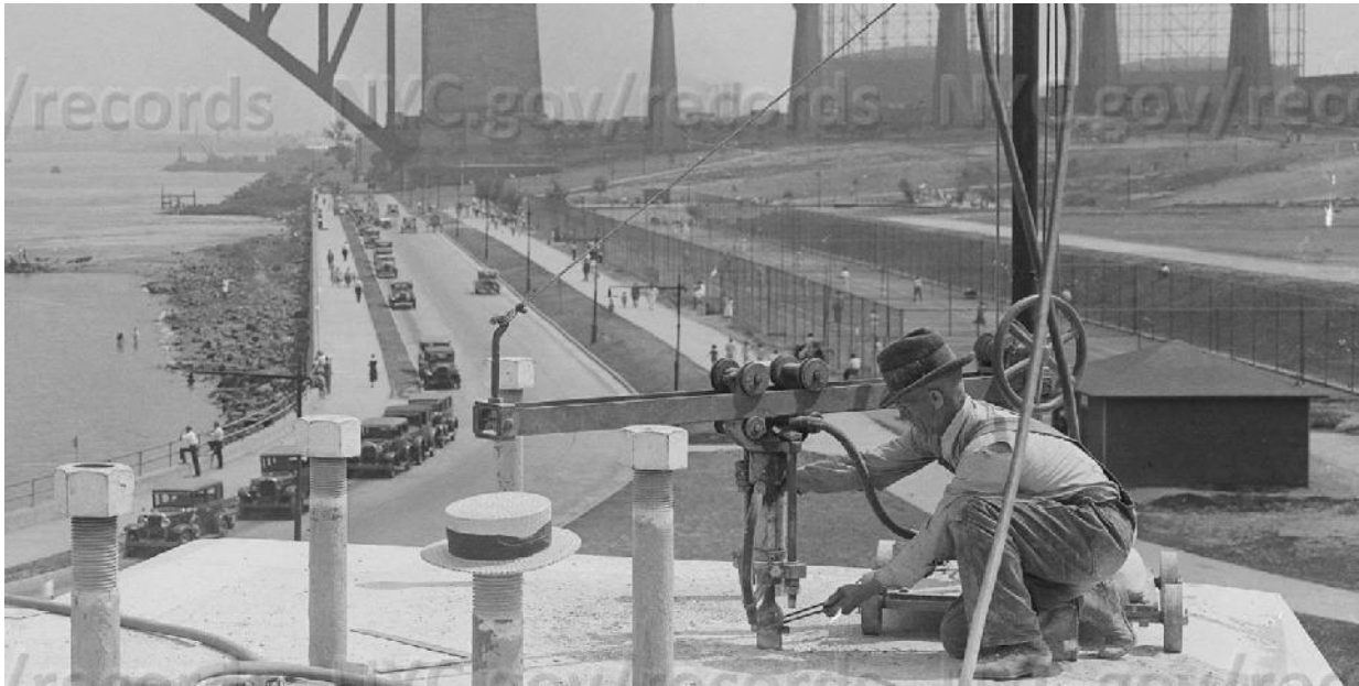
Photograph 13: Detail, Triborough Bridge Astoria Park pier. July 14, 1932. Image bps_15323. Courtesy New York City Municipal Archives.
