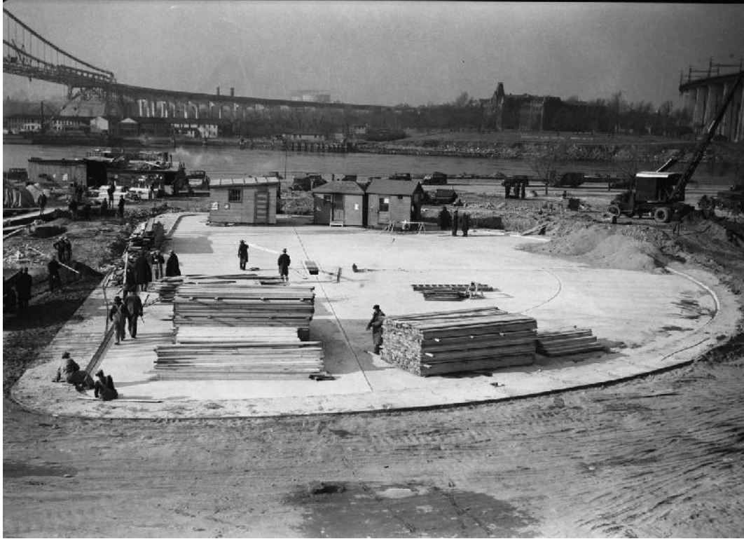
Photograph 19: Astoria Park pool under construction. November 27, 1935. Image 1844_Q004_11-27-1935. Courtesy New York City Parks Photo Archive.
