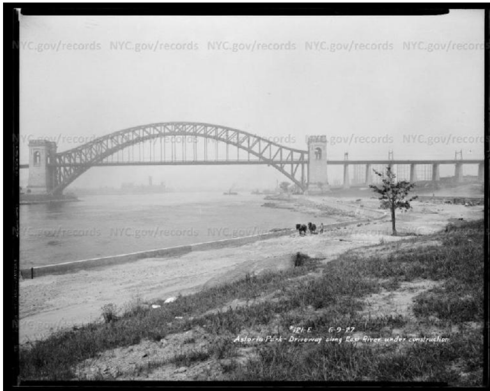
Photograph 10: Astoria Park – Driveway along East River under construction. June 9, 1927. Image bpq_0121-e. Courtesy New York City Municipal Archives.
