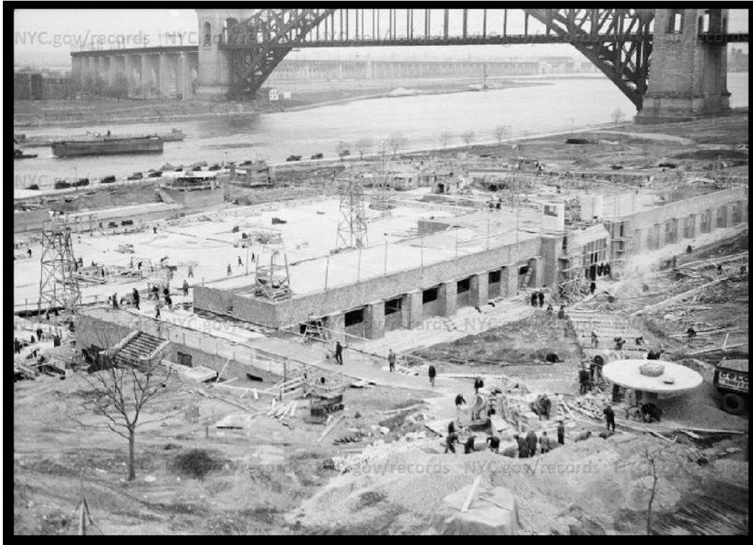
Photograph 21: Astoria Park swimming pool construction. April 3, 1936. Image dpr_2644. Courtesy New York City Municipal Archives.
