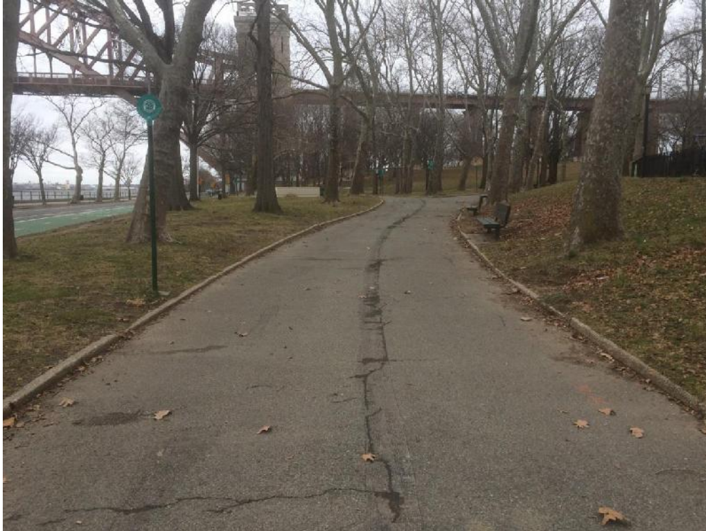
Photograph 5: Continued route of proposed sanitary sewer under pedestrian pathway. View looking northeast.
