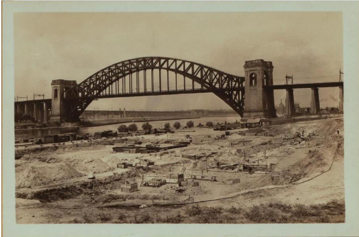
Photograph 15: Hell Gate Bridge, showing Astoria Park in Queens, while under construction. June 11, 1935. P.L. Sperr. Courtesy New York Public Library.
