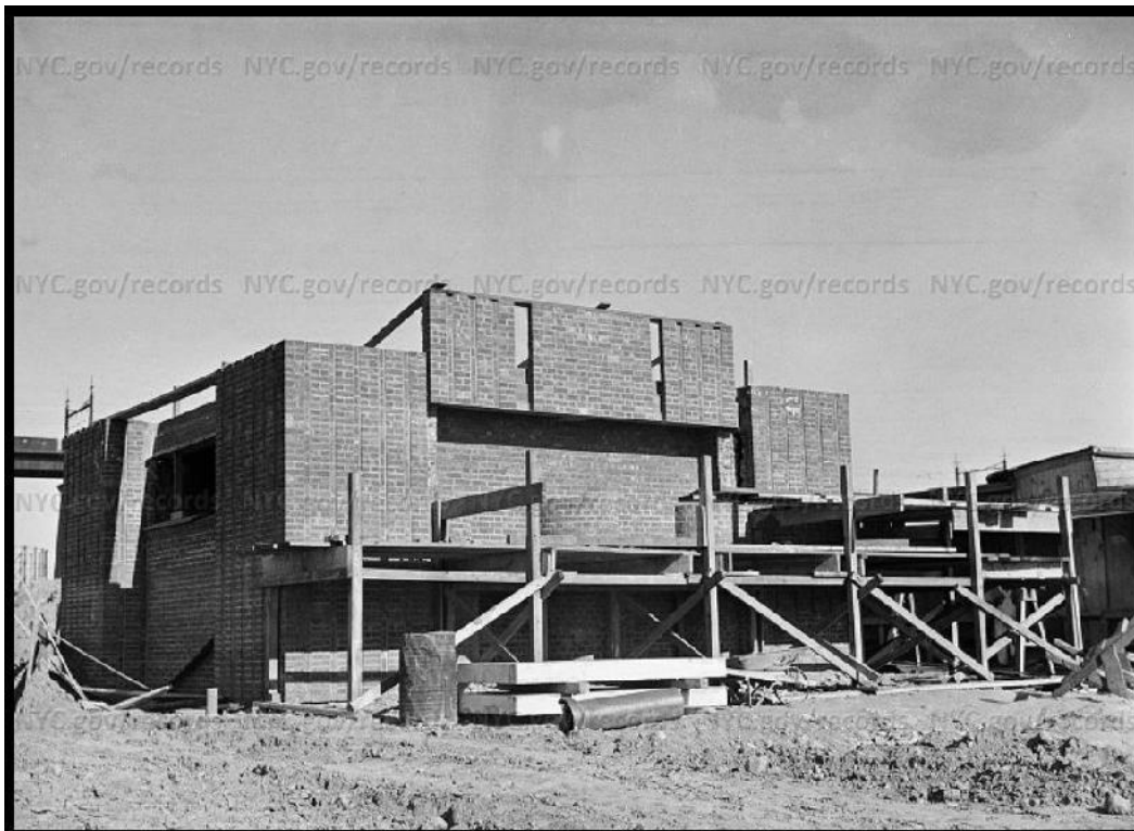
Photograph 18: Astoria Park north comfort station under construction. October 24, 1935. Image dpr_01753. Courtesy New York City Municipal Archives.
