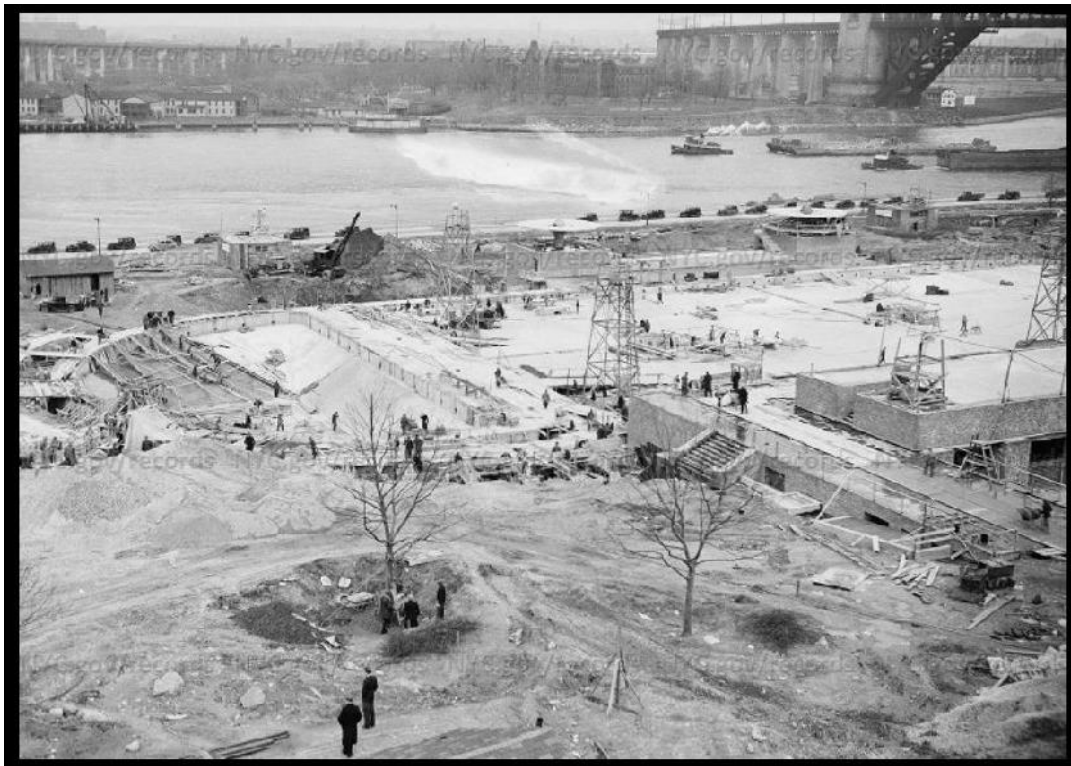
Photograph 20: Astoria Park swimming pool construction. April 3, 1936. Image dpr_2643. Courtesy New York City Municipal Archives.
