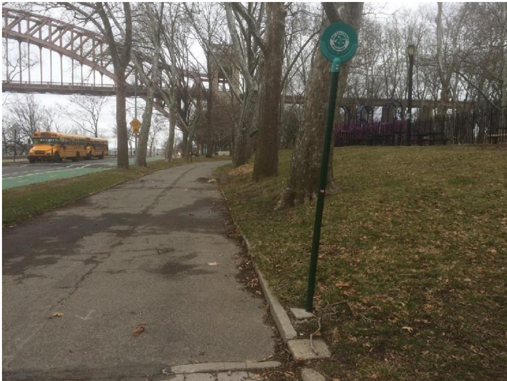
Photograph 4: Route of proposed sanitary sewer under pedestrian pathway with Hell Gate Bridge in background. View looking northeast.
