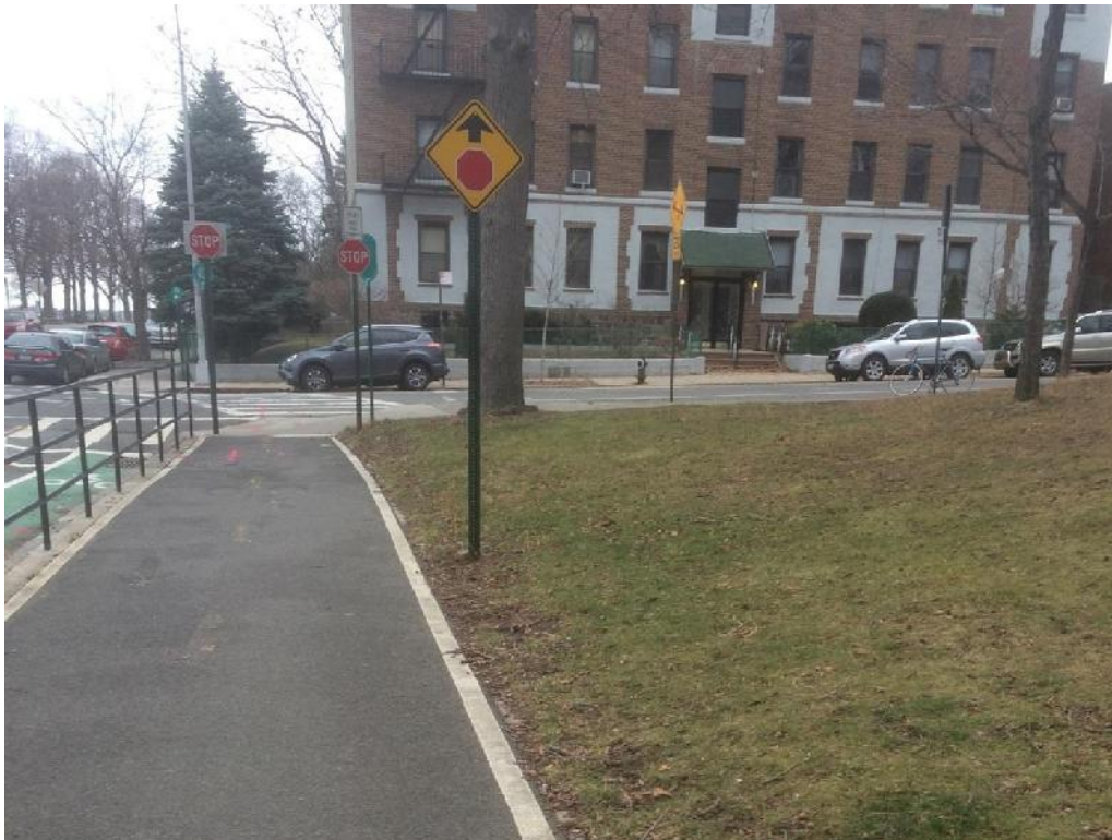
Photograph 8: Terminus of proposed sanitary sewer route at Ditmars Boulevard. View looking northeast.
