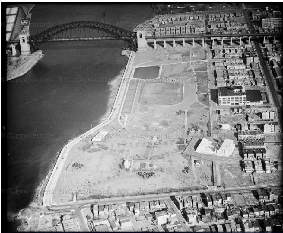
Photograph 14: Astoria Park, aerial photograph. January 1934. Image dpr_13744. Courtesy New York City Municipal Archives.
