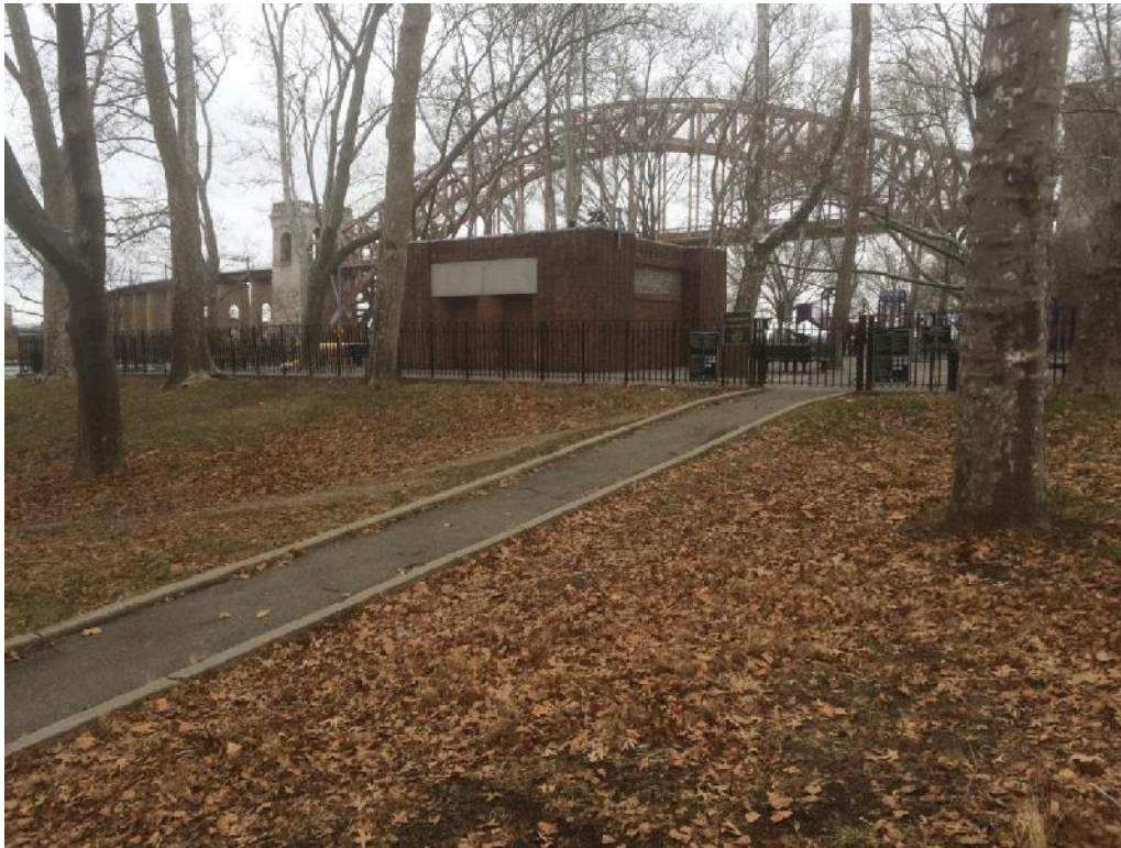
Photograph 1: North playground comfort station. Proposed sanitary sewer will run from building under pathway. View looking north.
