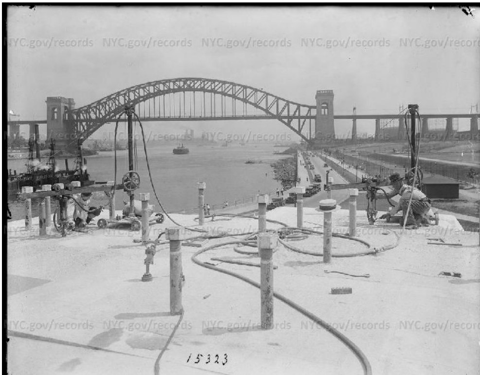
Photograph 12: Triborough Bridge Astoria Park pier. July 14, 1932. Image bps_15323. Courtesy New York City Municipal Archives.
