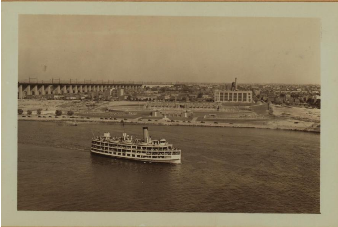
Photograph 25: Astoria Park. July 25, 1936. P.L. Sperr. Courtesy New York Public Library.
