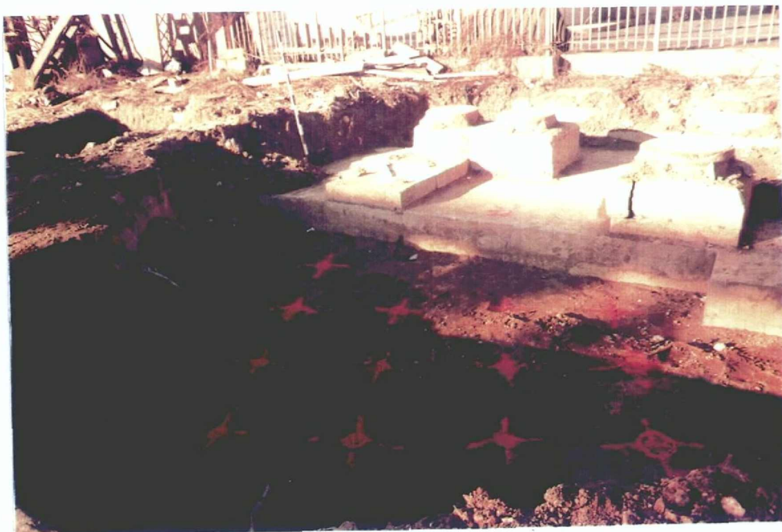
PHOTO 12 - Overhead steam line support excavation at east end of former Craneway location (view to N)
