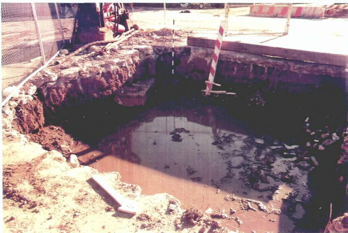
PHOTO 11 - Overhead steam line support excavation near north end of Second Street (view to SW)
