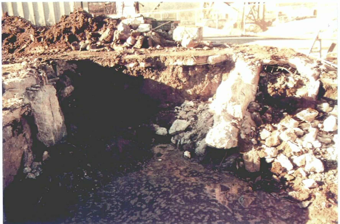
PHOTO 10 - Overhead line support base excavation near north end of Second Street (view to N)
