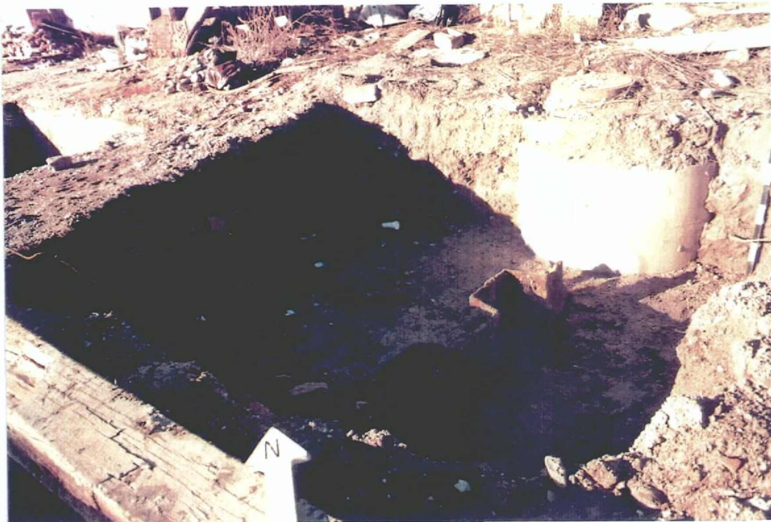
PHOTO 13 - Overhead line support excavation in former Craneway showing extent of impact and material encountered (view to N)
