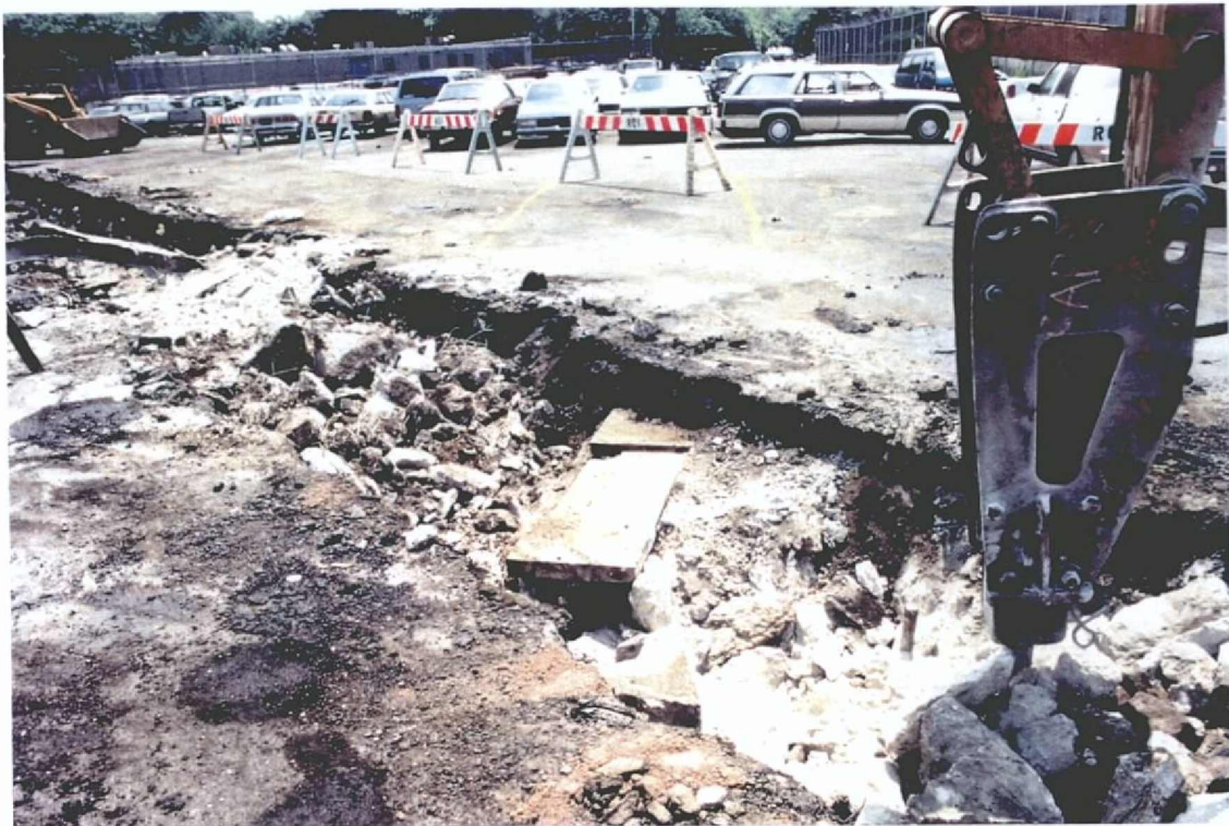
PHOTO 7 - Profile of one steel I-beam surrounded by concrete rubble (view to N)
