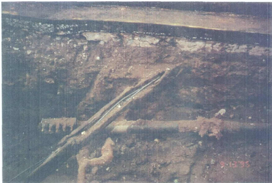
PHOTO 19 - Conduit excavation just east of Hudson Street intersection on Plymouth Street showing existing utilities encountered to base of trench (view to S)
