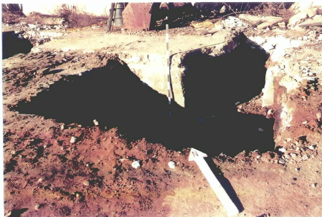
PHOTO 14 - Overhead line support excavation in former Craneway showing avoidance of concrete utility structure; edge of adjacent excavation visible at upper left (view to NNE)
