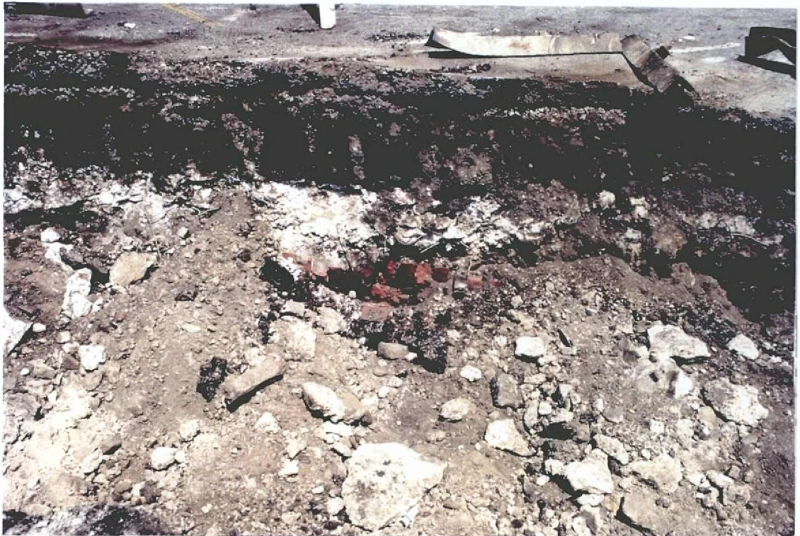
PHOTO 3 - Detail of conduit trench wall northwest of Third Street showing concrete and brick rubble and bituminous pavement in profile (view to NE)
