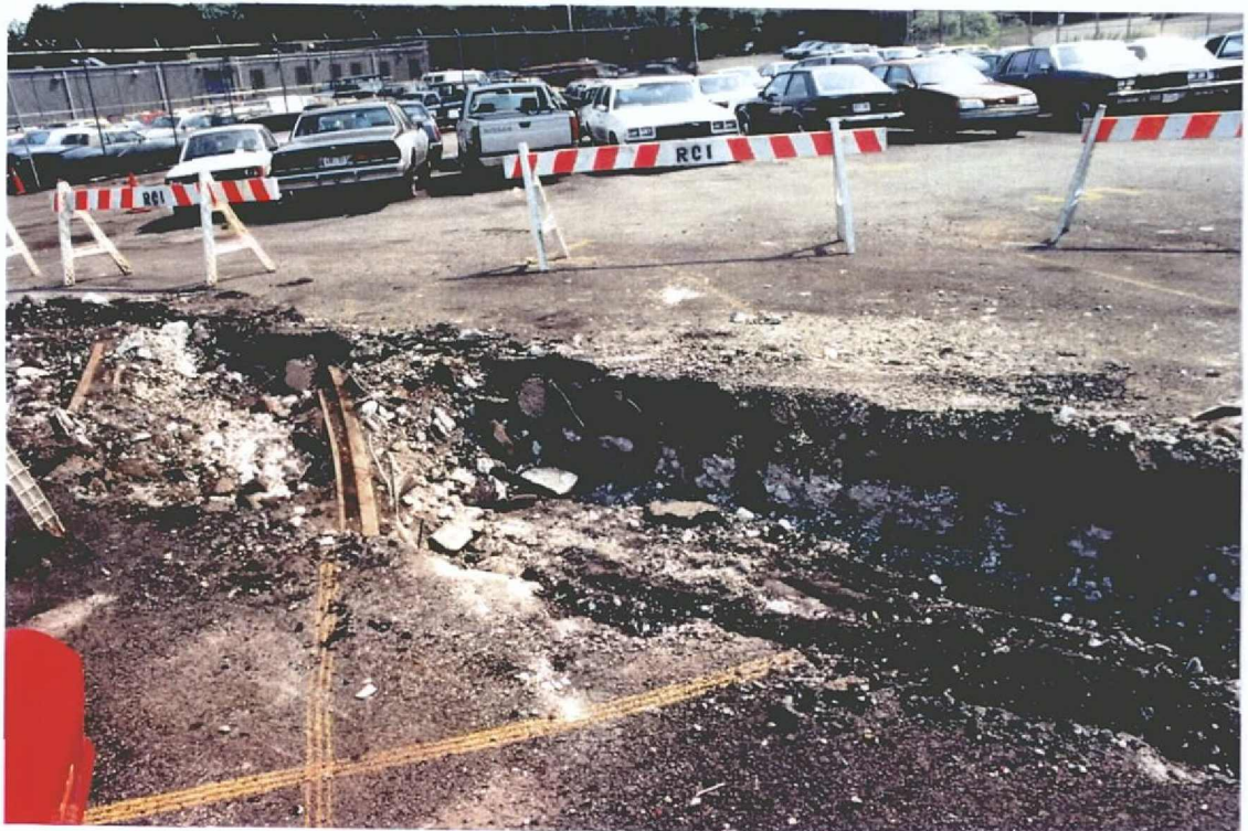
PHOTO 4 - Detail of conduit trench wall northwest of Third Street showing track remnants at left and concrete support base extending to right (view to N)
