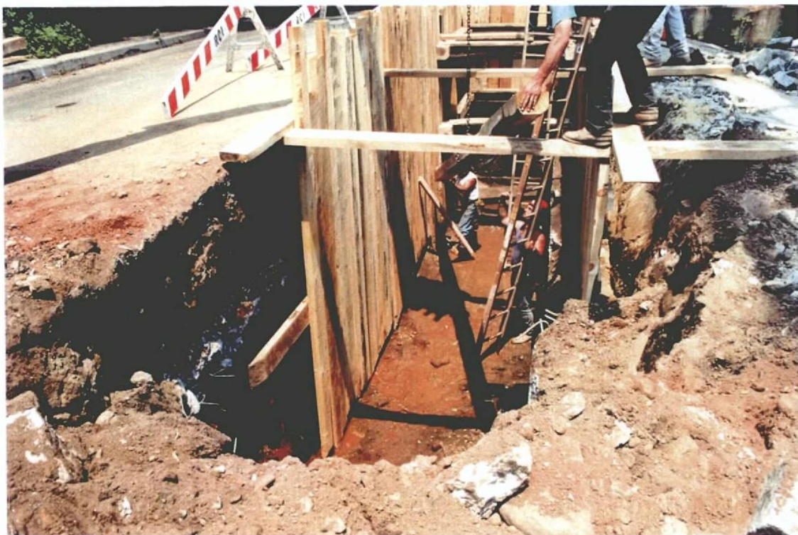
PHOTO 8 - Conduit trench along west side of First Avenue near manhole location showing previous road surface or slab of concrete with large aggregate and steel reinforcement ( view to N)
