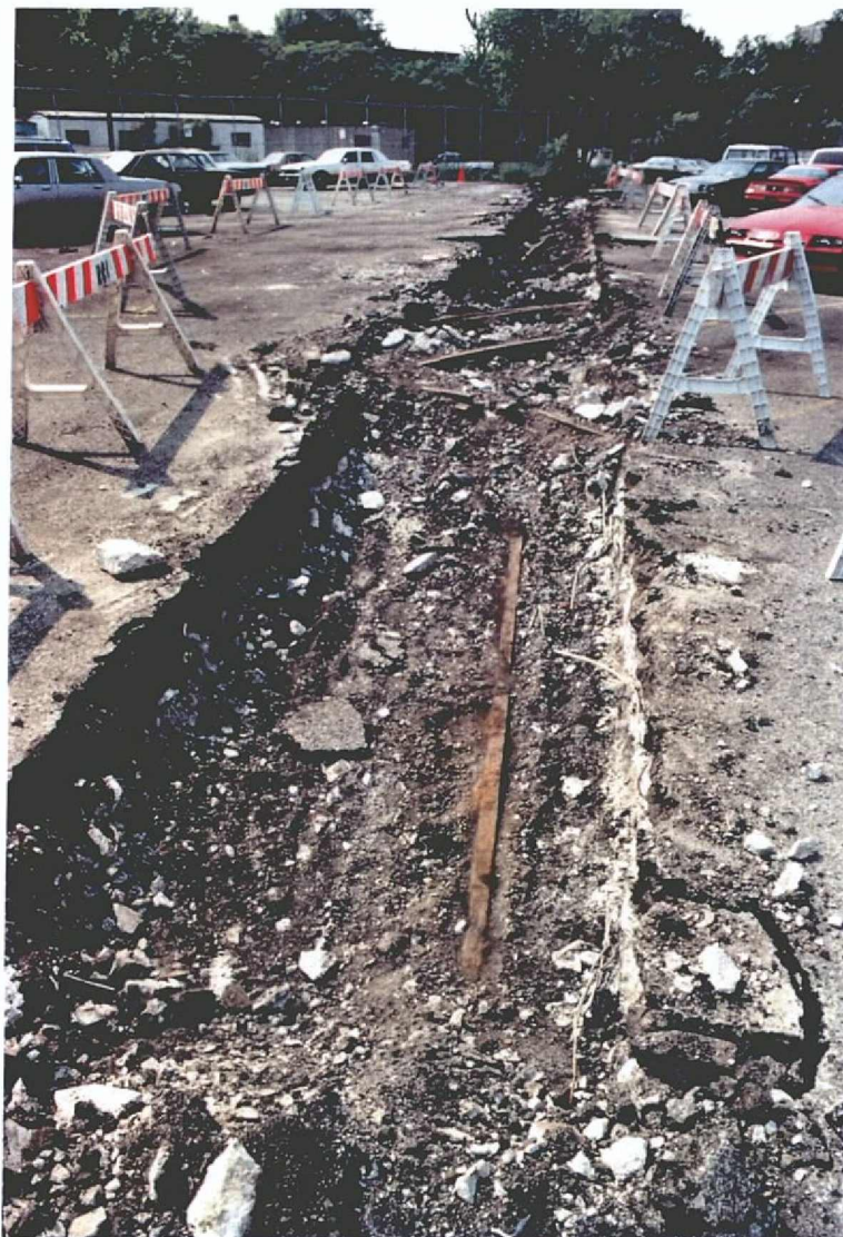
PHOTO 5 - Conduit trench along former course of Perr Avenue northwest of Third Street, now NYS impound lot, showing three sections of tra remnants (view to NW)
