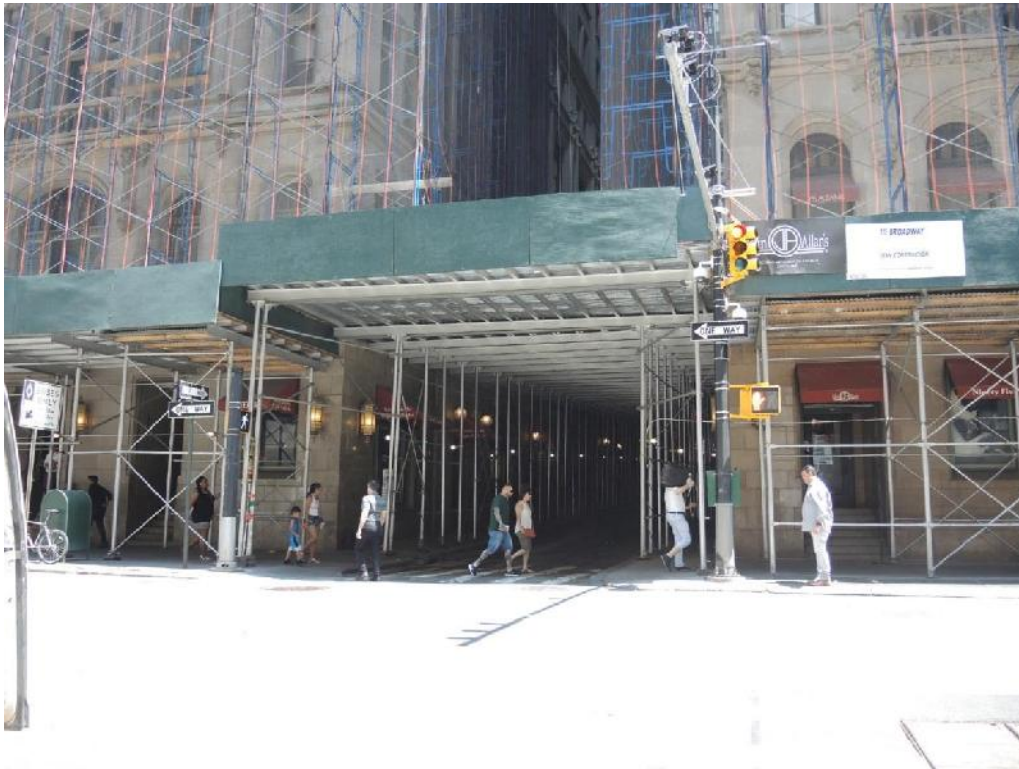
Photograph 2: Thames Street at Trinity Place with sidewalk shed scaffolding. View looking southeast.
