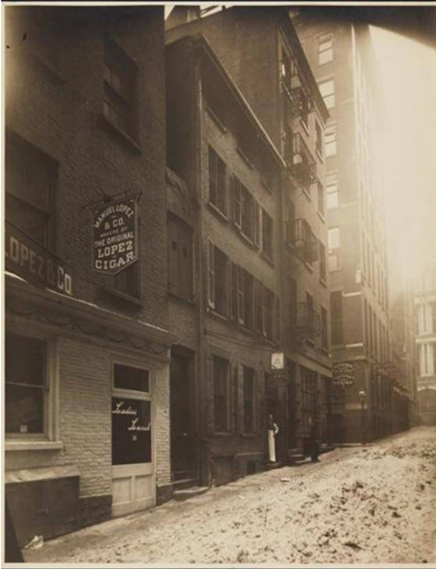
Undated photograph of original Thames Street in foreground, buildings on north side of Thames Street on left and background, with former Temple Street at lamppost. Rear of second Boreel Building is beyond lamppost. Courtesy Museum of the City of New York.
