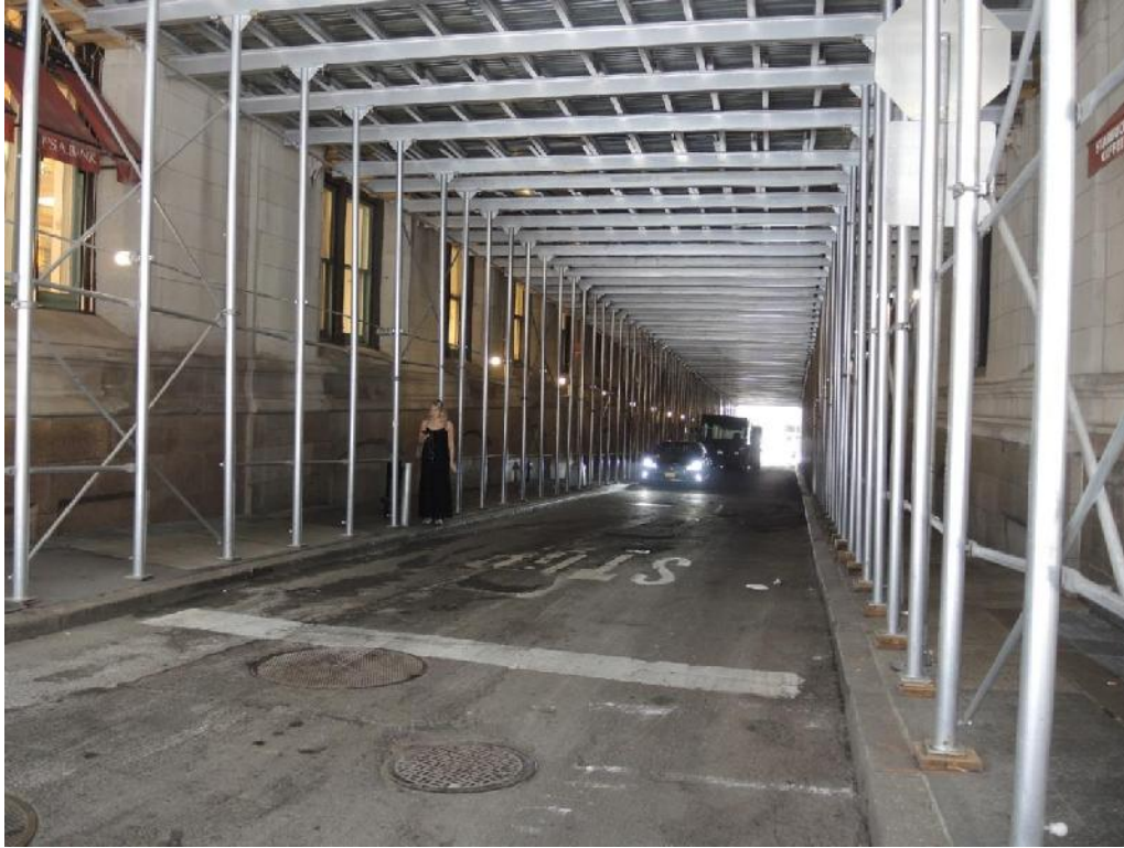
Photograph 3: Thames Street roadbed with sidewalk shed scaffolding. Note manholes in foreground. Trinity Place is in far background. View looking northwest.
