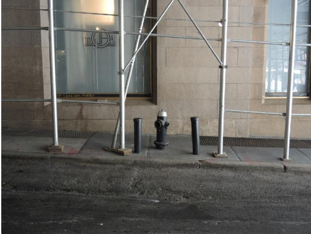
Photograph 7: Detail of hydrant and bollards on south side of Thames Street near Trinity Place. View looking southwest.
