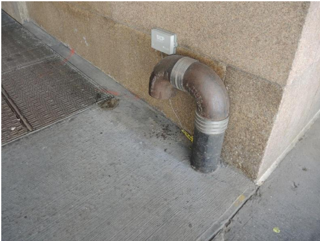
Photograph 8: Detail of sidewalk vaults and standpipe on south side of Thames Street at corner of Trinity Place. View looking southwest.
