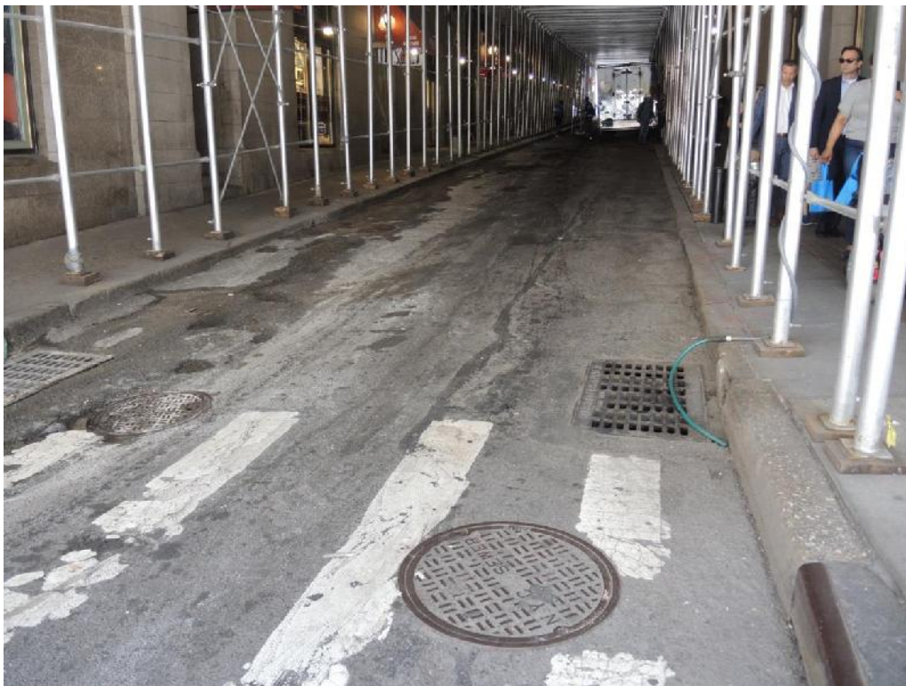
Photograph 4: Thames Street roadbed with sidewalk shed scaffolding. Note sewer manholes and catch basins in foreground. Broadway is in far background. View looking southeast.
