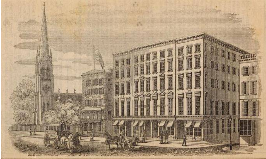
1851 image of the newly constructed Boreel Building stores. Original Thames Street is to the left, with New England House and Trinity Church to left of Thames Street. Modern Thames Street runs under the Boreel Building. From The Great Metropolis or New York Almanac for 1851 (Trow 1851).
