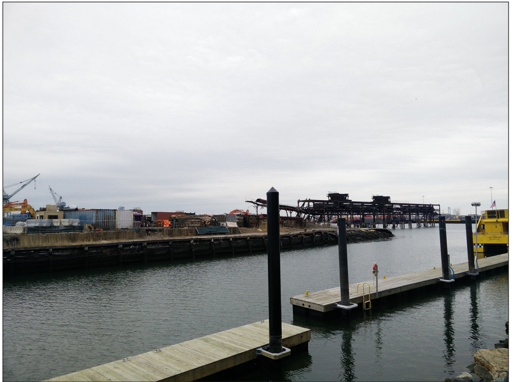
The southwestern portion of the project site including the existing steel pier that extends south from the bulkhead 6
