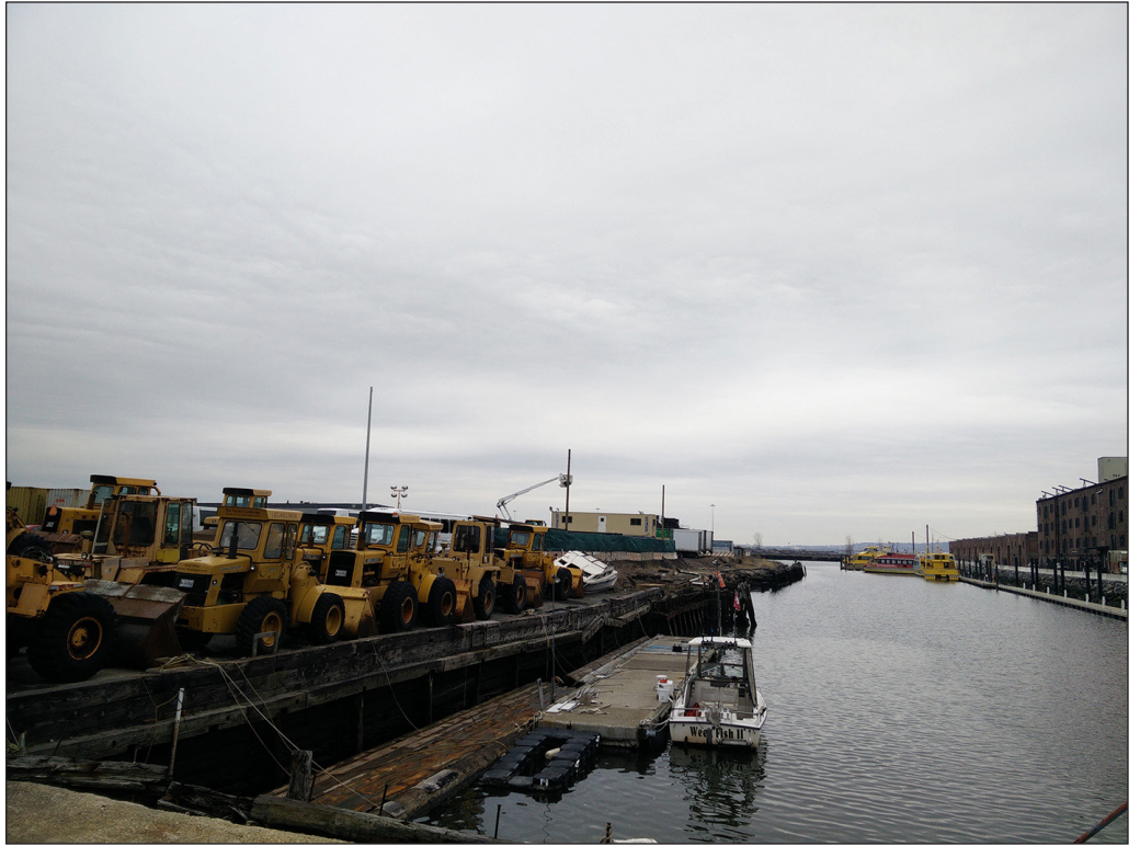
View south at the deteriorating bulkhead lining the northwestern side of the project site 5
