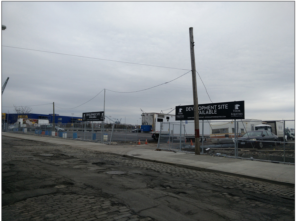
View southeast from Beard Street at the northern portion of the project site 4
