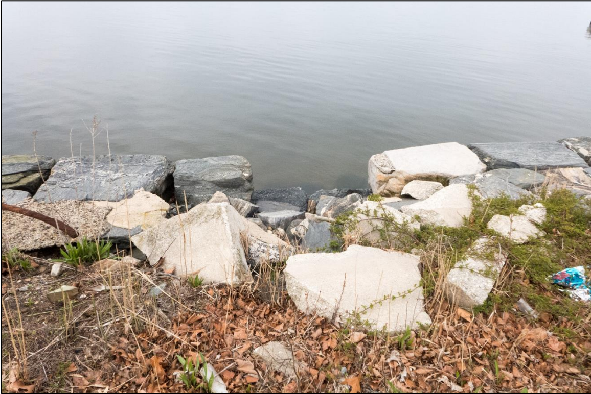
Image 21: Areas of missing stone in dry-laid seawall; looking west.
