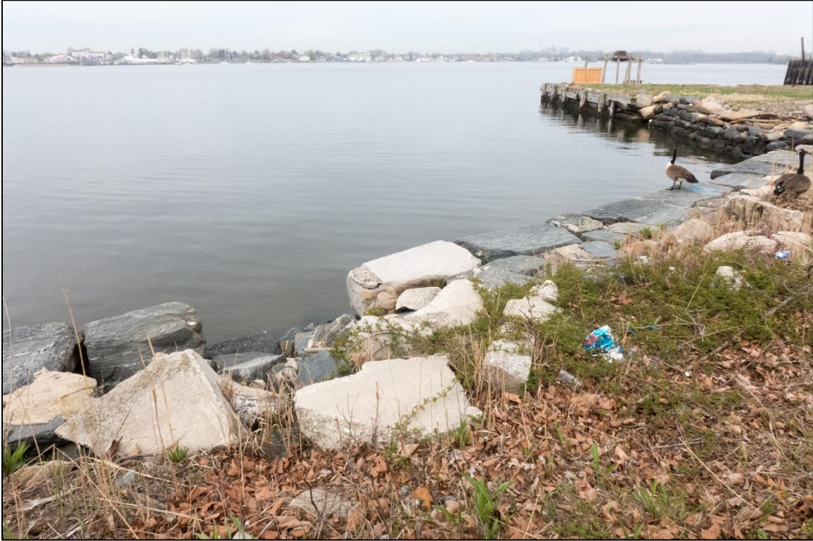
Image 26: West APE, dry-laid stone seawall; facing northwest.
