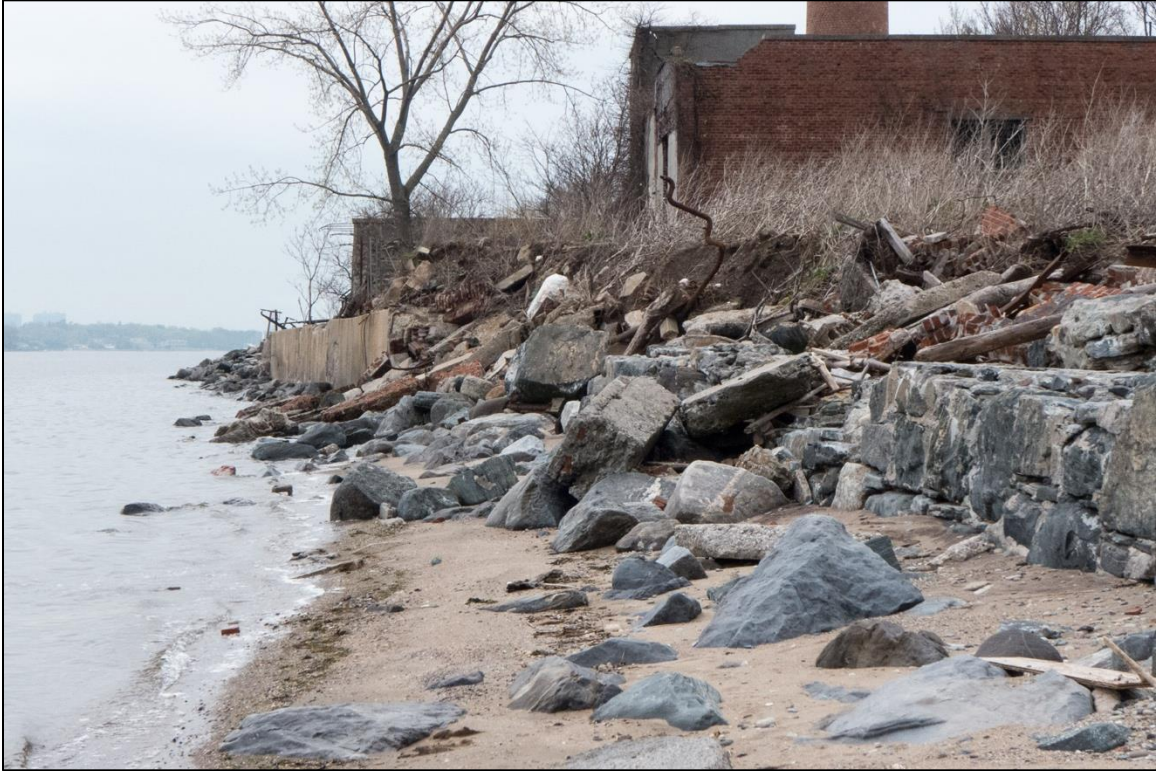
Image 18: Loose stone and large debris between concrete wall and the stone seawall (beginning of APE); looking south.
