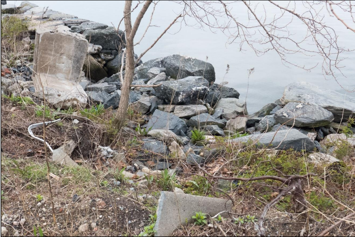
Image 22: Seawall damage and large debris on slope abutting seawall; looking southwest.
