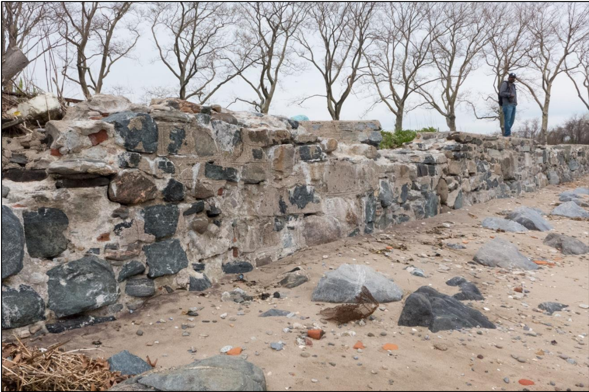
Image 33: East APE, damaged seawall, large stones scattered on beach; facing northwest.
