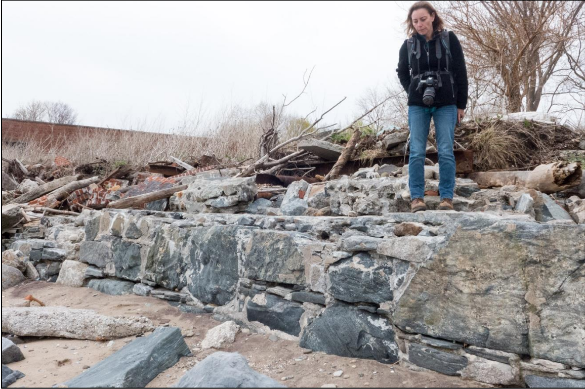
Image 32: East APE, damaged mortared stone seawall and surrounding debris; facing southwest.
