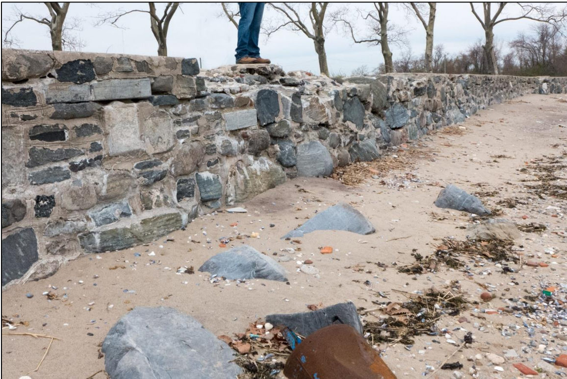
Image 19: Damaged section of seawall in the APE; looking northeast.
