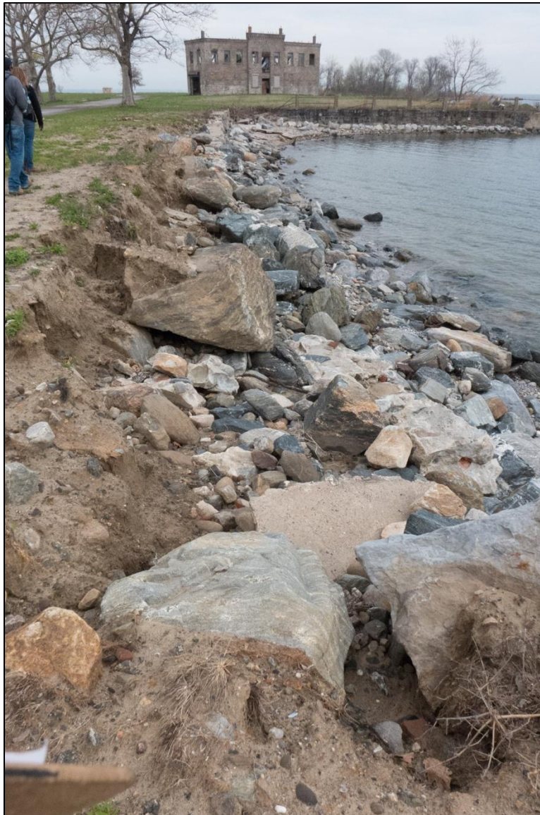
Image 34: East APE, damaged seawall and loose stone and debris obscuring beach; facing north.
